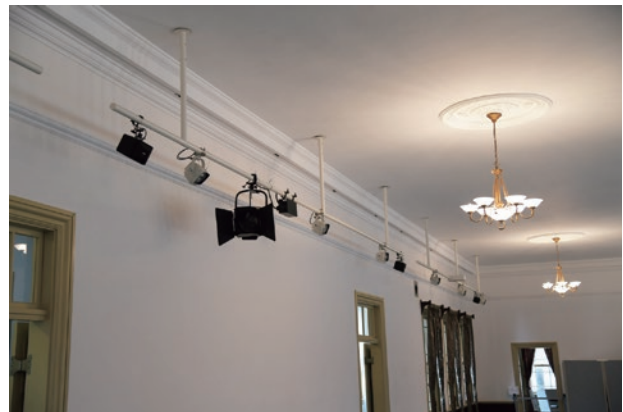
photo Baton installed on both sides of the ceiling wall of the hall, Additional lighting equipment, fire alarms, speakers, etc., are installed on this baton
