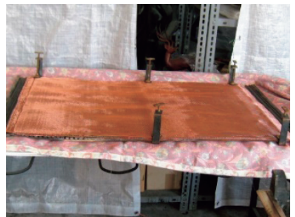
photo app.2-20 Wire mesh welding
