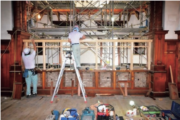
photo 38 Screen frame mounting
