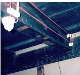
photo 12 Insulator wiring work construction example, Yachiyoza (Photo provided by : Yamaga City Board of Education)
