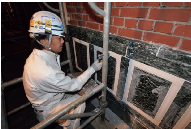
photo 20 West side public space waist wall stone construction
