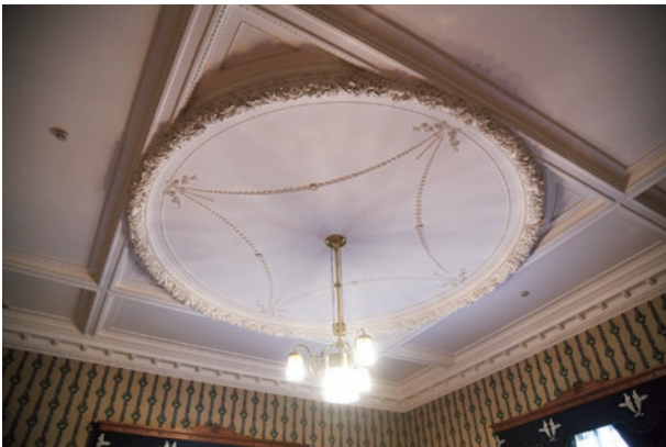
photo Plaster ceiling in the “governor's office”
