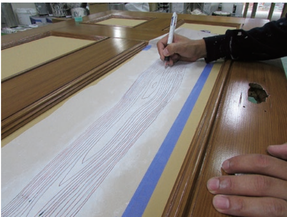
photo 18 Graining process (medium figured grain) ⑥ -1 panel board medium figured grain marking
