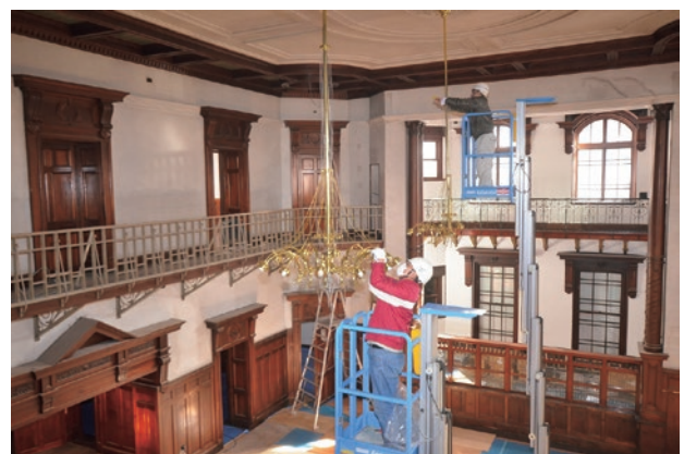
photo 45 Restoration lighting equipment installation
