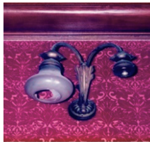
photo app.2-35 Cafeteria: damaged lamp
