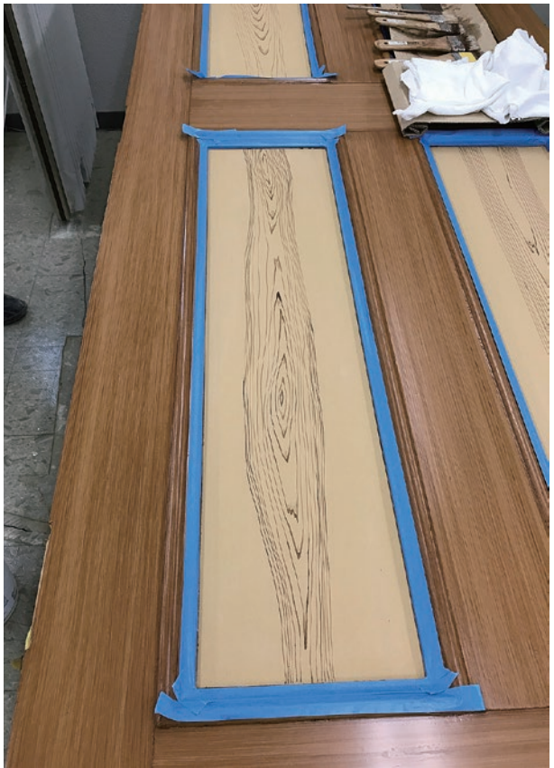
photo 20 Graining process (medium figured grain) ⑥ -3 panel board medium figured grain-2
