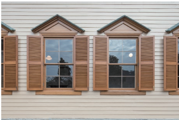
photo 13 Main building shutter (after repair)
