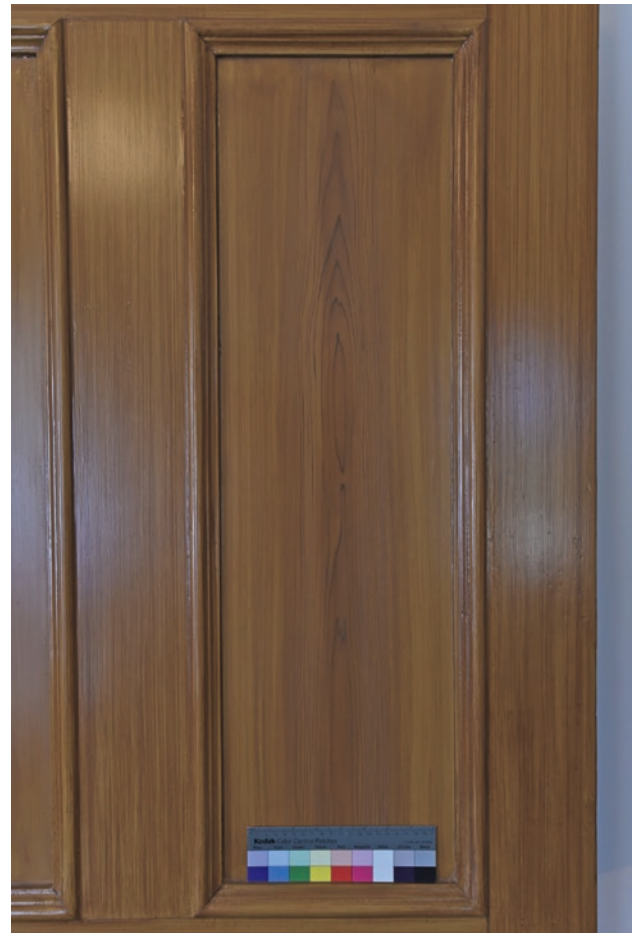
photo 31 Graining completed (medium figured gain) - panel board
