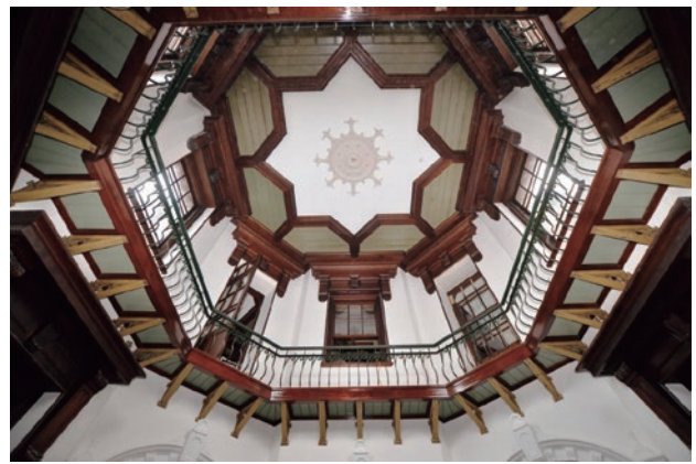
photo 32 Octagonal tower handrail completed
