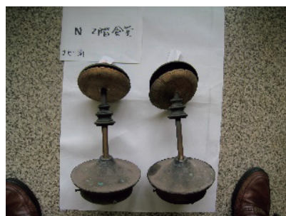
photo app.1-60 Corrosion
