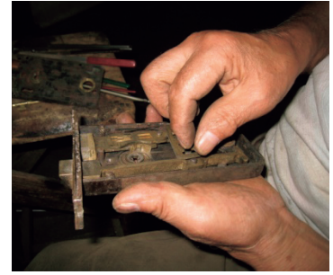
photo app.2-30 Box lock adjustment
