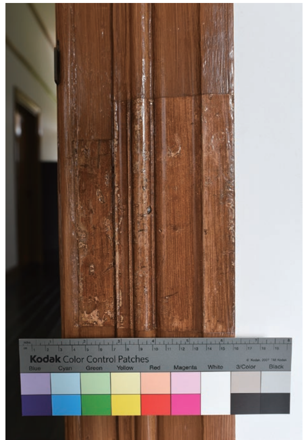
photo 7 Bottom graining-straight grain (Main building No. 4 room door frame)
