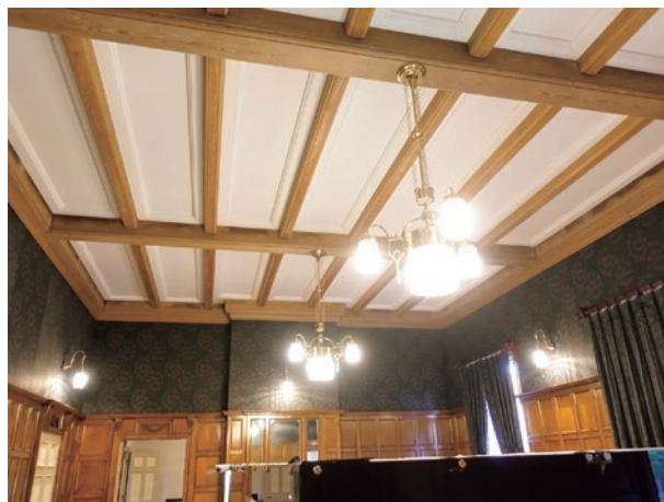
photo Plaster ceiling in the “high government cafeteria”
