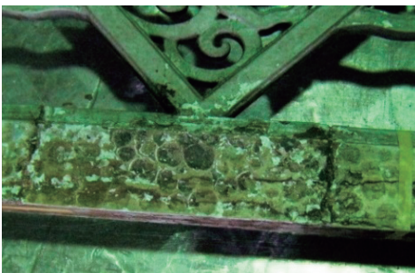
photo app.2-4 Cracks
