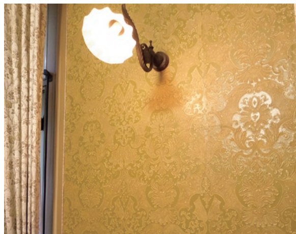
photo Restored Gold-embossed wallpaper "Kinkara-kawashi" *1 in bedroom 1 (northeast room) on the 2nd floor
