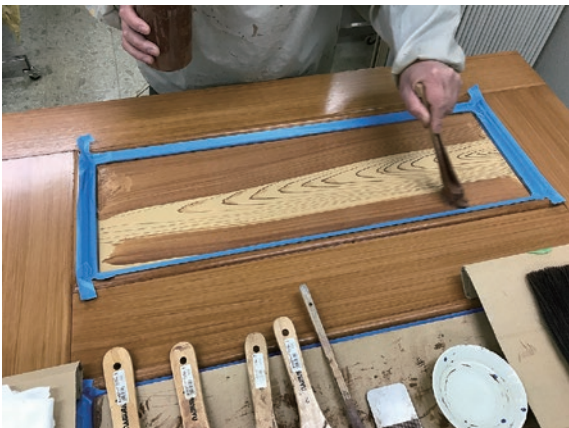
photo 21 Graining process (medium figured grain) ⑥ -4 panel board medium figured grain-3
