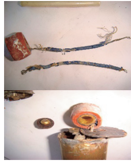
photo app.1-10 Electric wire state in socket
