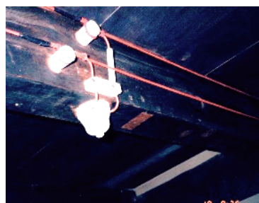
photo 12 Insulator wiring work construction example, Yachiyoza (Photo provided by : Yamaga City Board of Education)
