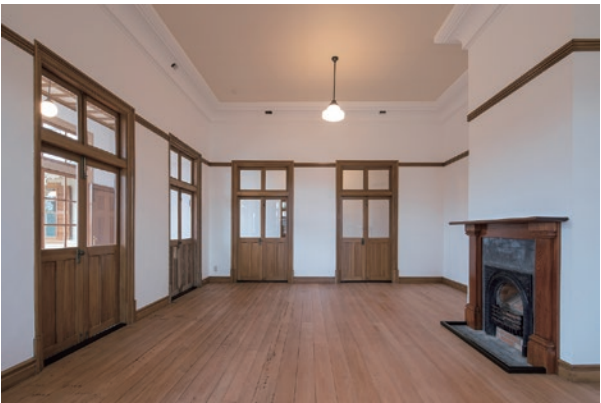
photo 10 Annex No. 7 room (after repair)
