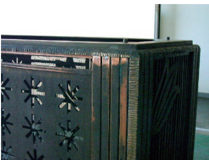
photo app.2-21 Damaged frame casting molding
