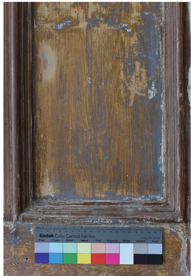
photo 6 Bottom graining-bamboo figured grain (Main building No. 4 room door endplate)
