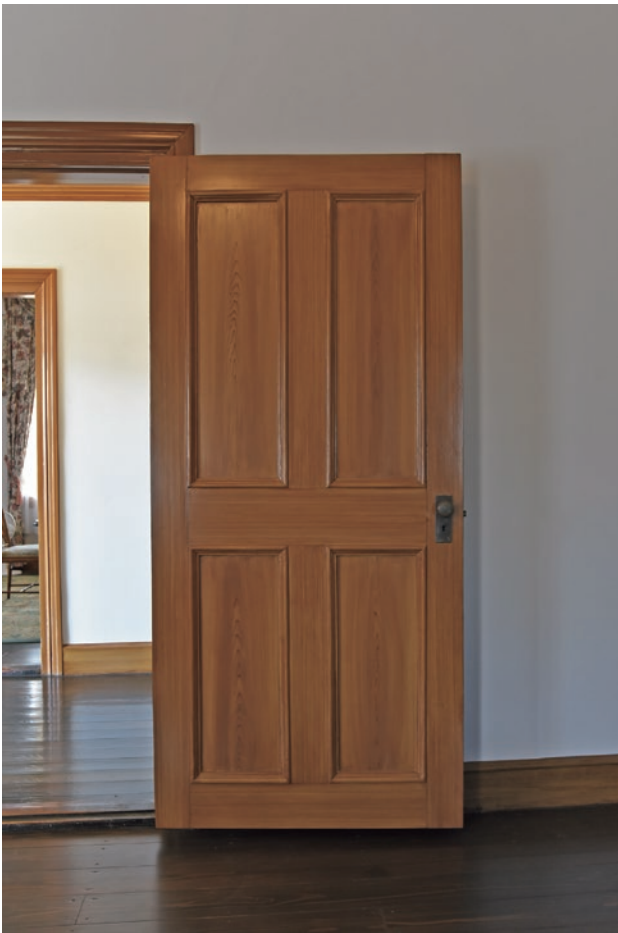
photo 30 Graining completed - door
