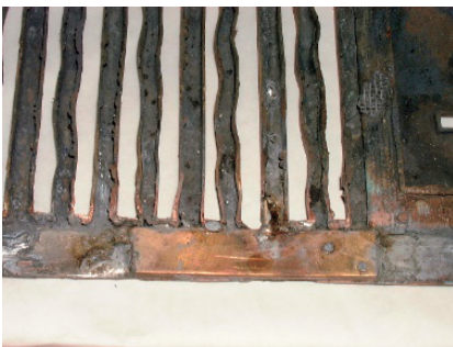
photo app.2-15 Back refill metal fitting welding
