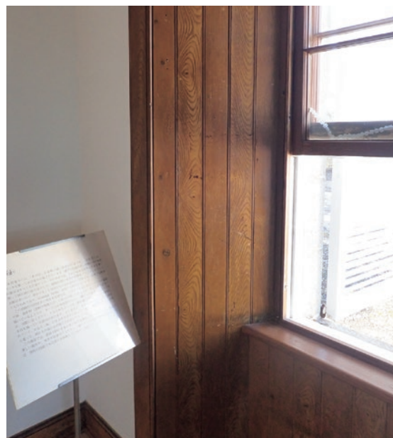
photo Graining that remains on the window frame, probably original
