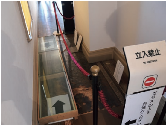
photo The original linoleum floor that remains in the corridor of the north wing of the chamber
