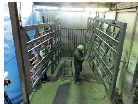
photo app.2-8 Repair work
