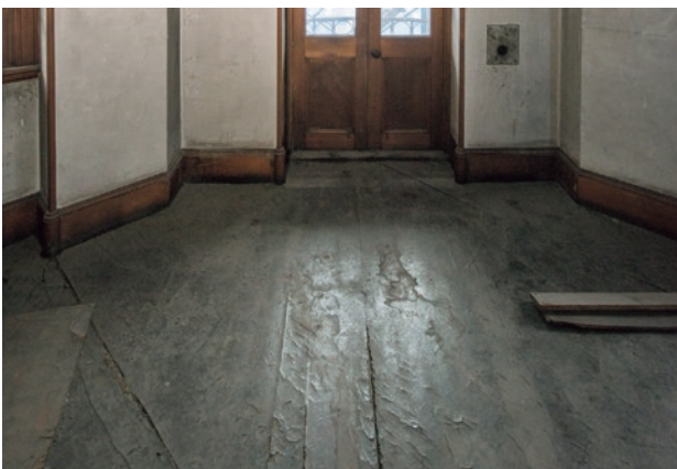
photo 10 Linoleum with floor finish of warehouse (octagonal penthouse)
