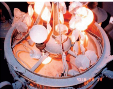
photo app.2-45 Defective beads
