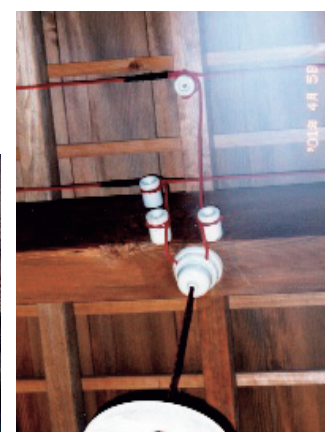
photo 12 Insulator wiring work construction example, Yachiyoza (Photo provided by : Yamaga City Board of Education)
