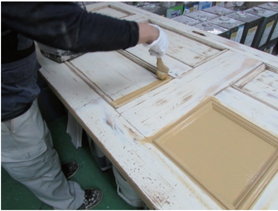
photo 16 Graining process ④ intermediate coating
