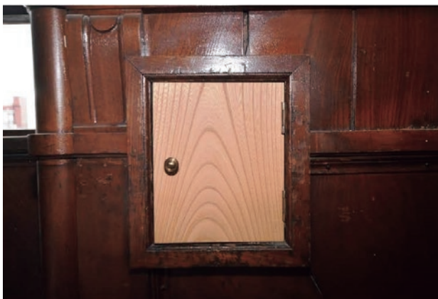
photo 25 Shutter winder lid supplement
