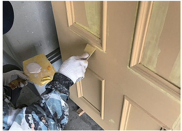
photo 17 Graining process ⑤ putty application
