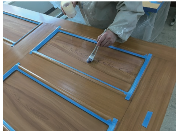
photo 24 Graining process ⑦ clear finish
