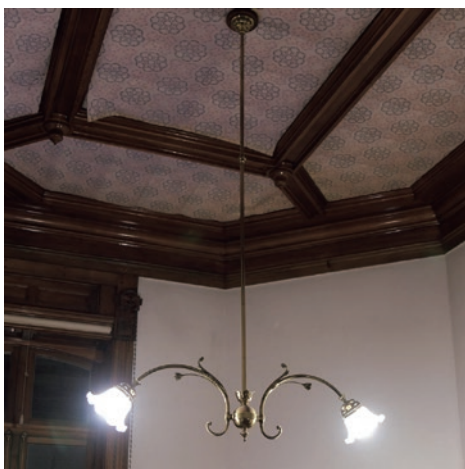
photo Lighting equipments in the branch manager's room (restored based on old photographs; the same applies to the first reception room)
