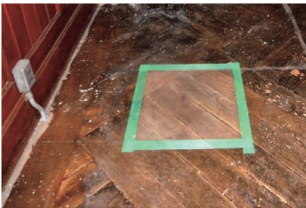
photo 12 Branch manager's room (former second reception room) parquet floor
