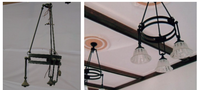
photo app.1-46 Billiard room on the 1st floor, before and after repair
