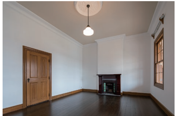
photo 11 Main building No. 2 room (after repair)
