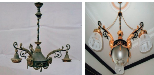
photo app.1-43 Reading room on the 2nd floor, before and after repair
