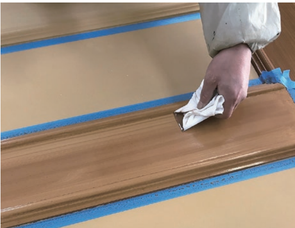
photo 27 Graining process (straight grain) combing
