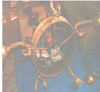
photo app.1-29 Dismantling
