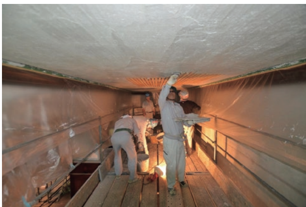
photo 16 West side public space ceiling
