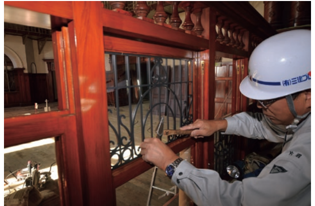
photo 39 Screen hardware installation
