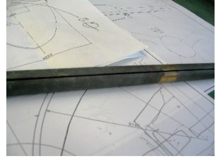
photo app.1-33 Central pipe brass joint damage crack
