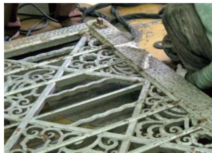
photo app.2-5 Cracks
