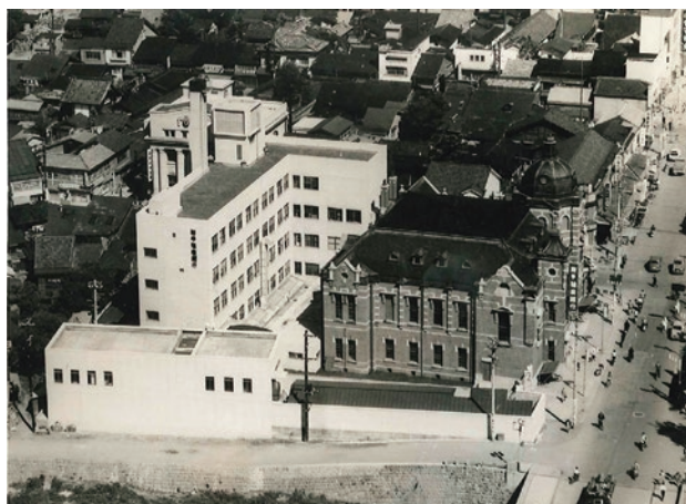
photo 4 Bank of Iwate (photographed in 1959, Bank of Iwate collection)
