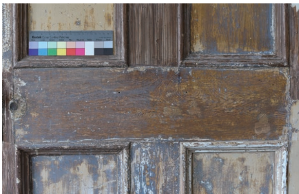
photo 5 Bottom graining-eyeball figured grain (Main building No. 4 room door middle stile)
