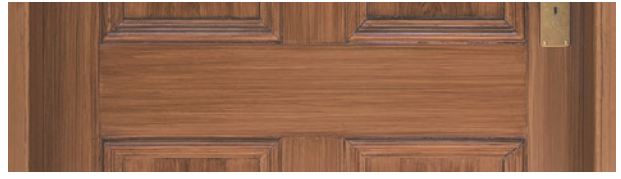
photo 9 Main building front door (after repair)
