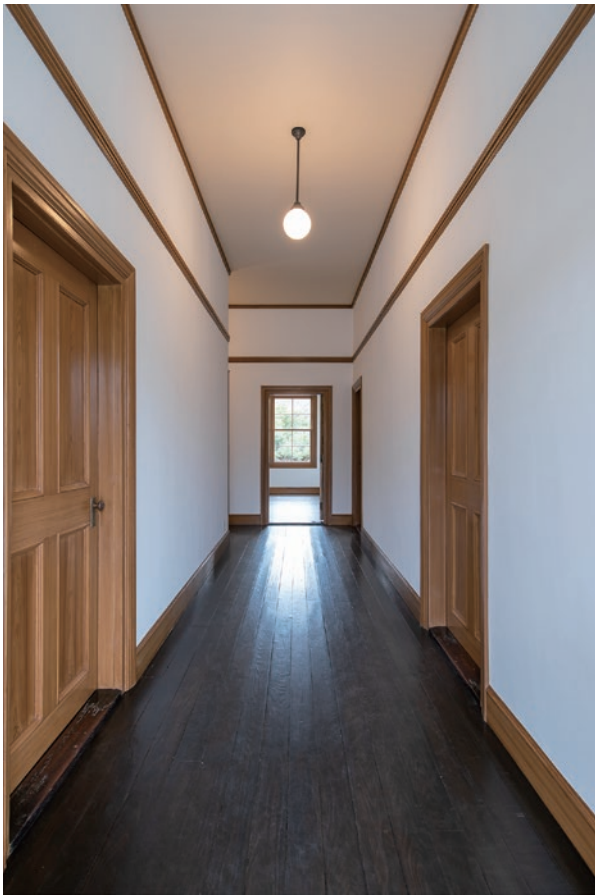
photo 12 Main building corridor 1-A (after repair)
