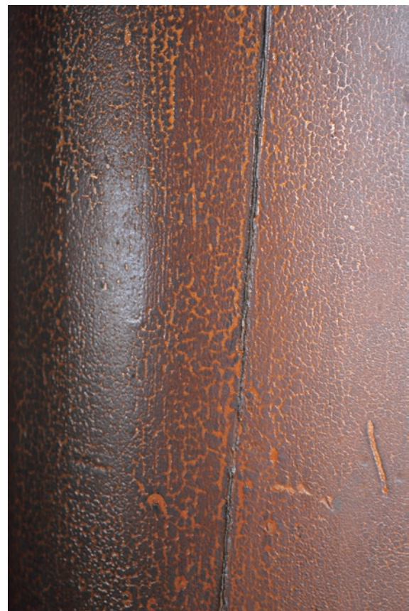
photo 14 Scale-like cracks in wooden parts of the wall
