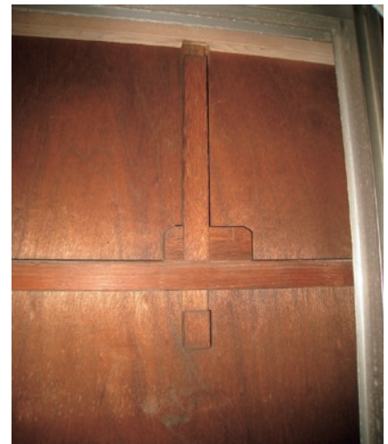
photo app.2-25 Monkey-type lock - left: direction of movement, right: when unlocked
