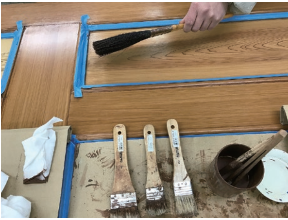
photo 23 Graining process ⑥ -6 panel board brush blur
