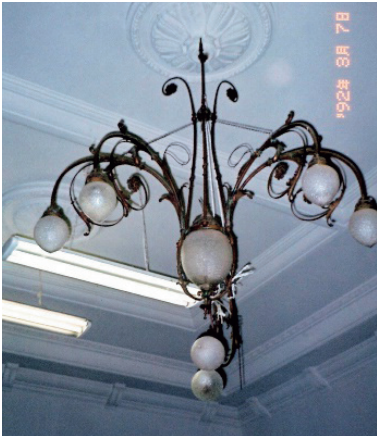
photo app.3-7 Photo when it was diverted to the general meeting room on the 2nd floor (Removed and stored afterward)
