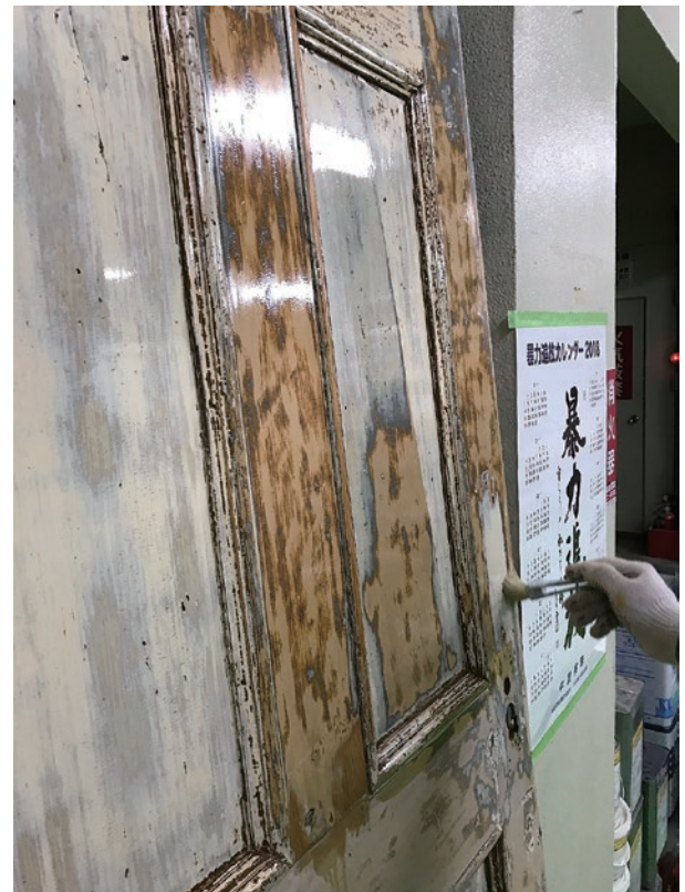
photo 15 Graining process ②③ sealer coating and undercoating
