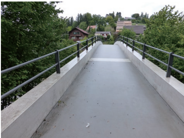
photo 29 Condition of the bridge's surface
