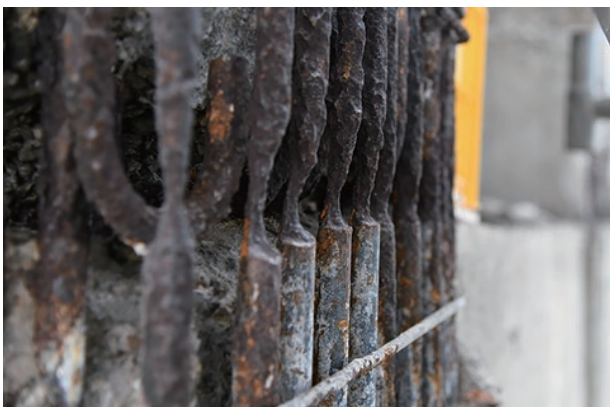
photo 2-6: Corroded rebar
