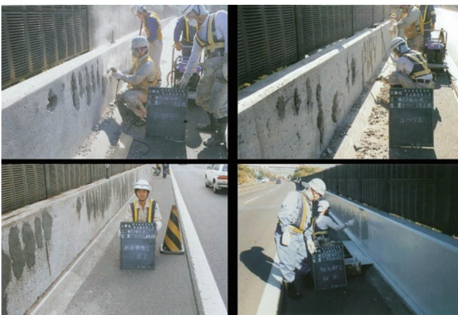
figure 7 Patch repair method (overview of the concrete construction being repaired 3 )
