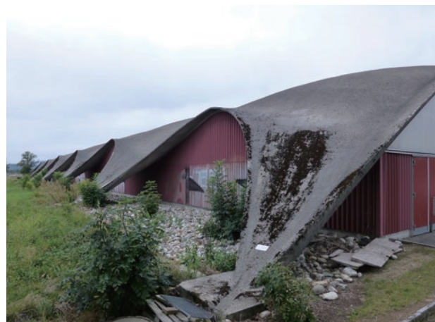
photo 51 A structure consisting of 6 connected shell roofs
