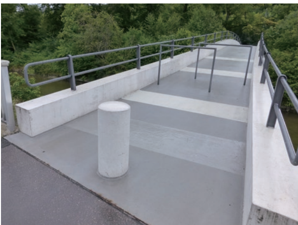
photo 30 General view of the floor slab
