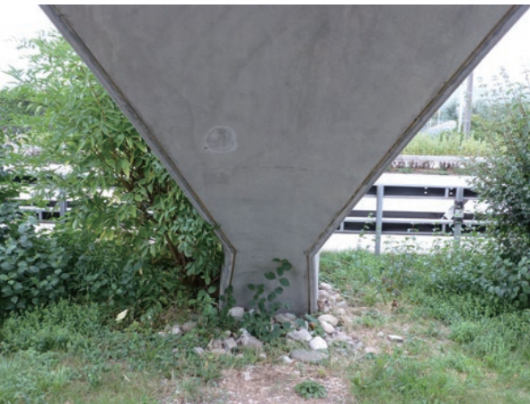
photo 58 The apex of each triangular concrete shell anchored to the ground
