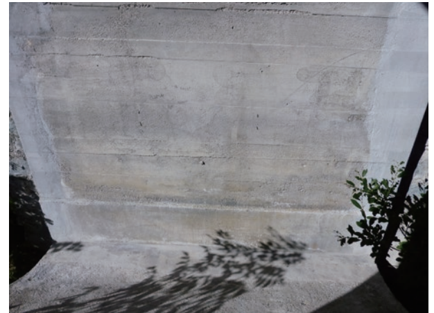
photo 48 Repaired bottom arch ring surface
