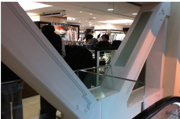
photo 7 Takashimaya Tokyo Department Store, reinforcement with bracing decorated to match the store interiors
