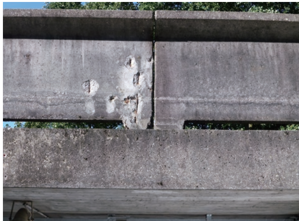
photo 64 Repaired concrete balustrade wall
