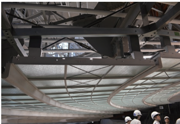
photo 28 Newly installed ceiling of glass fiber reinforced gypsum (GRG) panels
