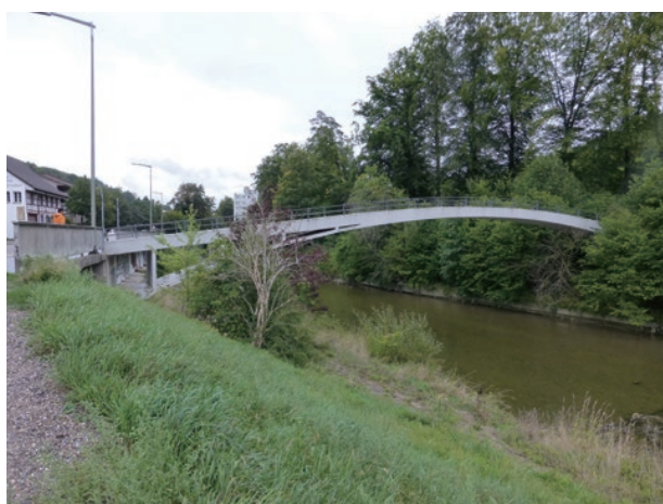
photo 27 Overall view of the Töss Footbridge
