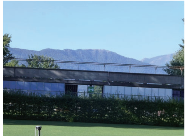
photo 60 Pedestrian bridge leading to a swimming pool
