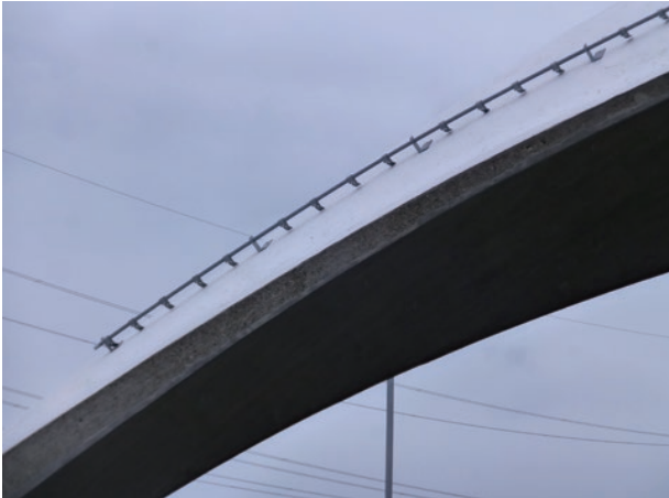
photo 57 Installed snow guards
