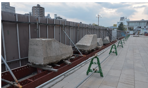
photo 6-9: The quadruple foundation elements were removed for underground preservation
