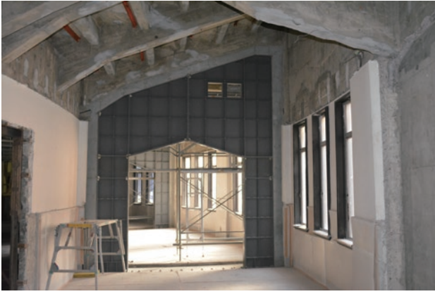
photo 26 Steel frame panel walls, corridor around auditorium
