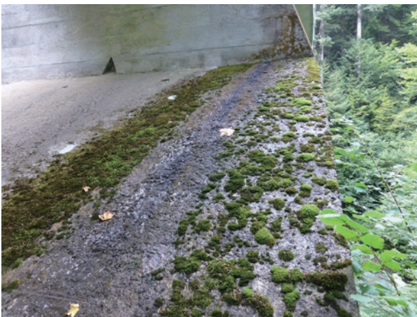
photo 14 Drainage system running from the arch rib
