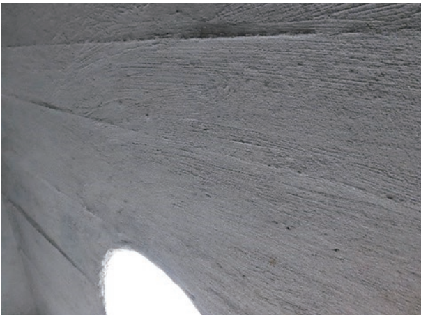
photo 40 Timber formwork used for the construction of the Salginatobel Bridge
