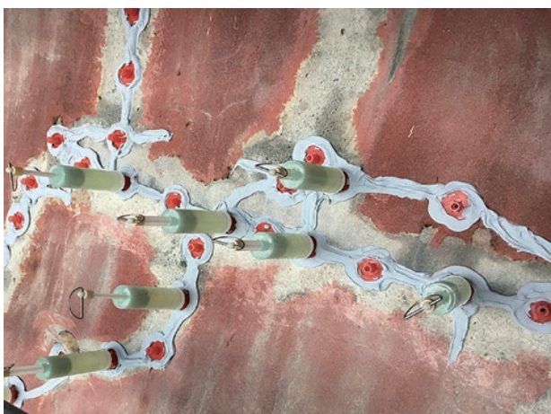
photo 3-6: Part of the protective film peeling off from the dam's upstream face (photo provided by : Tokyo Electric Power Company Holdings, Incorporated)
