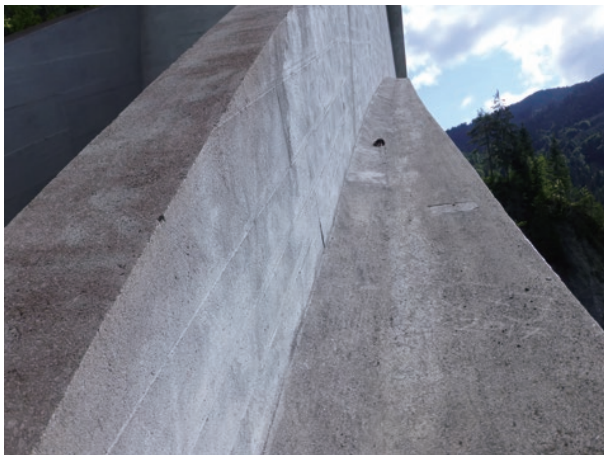
photo 39 South-side arch ring concrete
