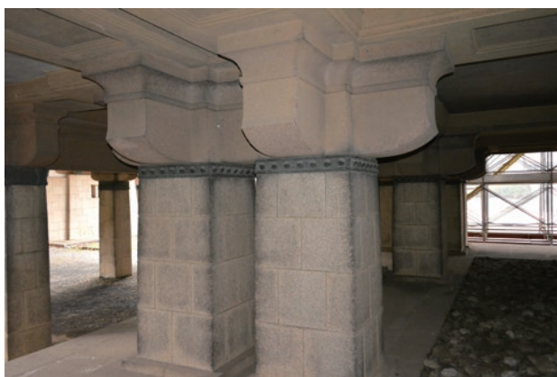
photo 3 Meiji Jingu Homotsuden Treasure Museum Middle Storehouse, first floor column
