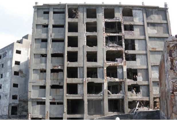
photo 7 Building no. 30 on Gunkan-jima (Hashima)
