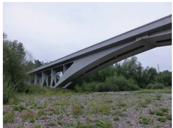
photo 20 Twin arches of the Felsegg Bridge
