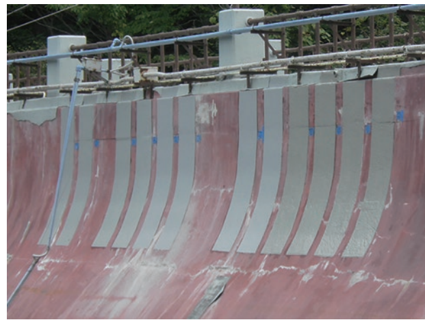
photo 3-4: Monitoring of the protective coating applied on a trial basis (photo provided by : Tokyo Electric Power Company Holdings, Incorporated)
