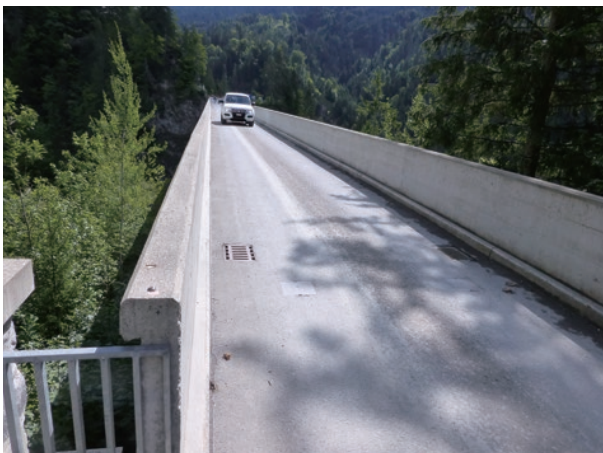
photo 34 Drainage system on the bridge surface (provision of catch-basins)
