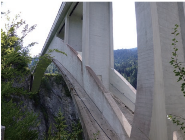
photo 37 Arch rings on the north and south sides
