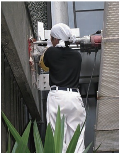
photo 5 Concrete core drilling
