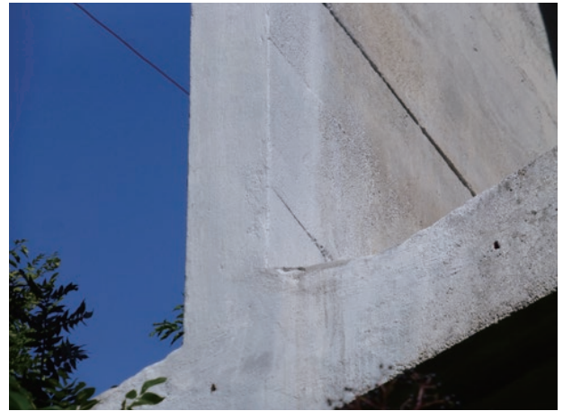
photo 47 Repaired spandrel wall base
