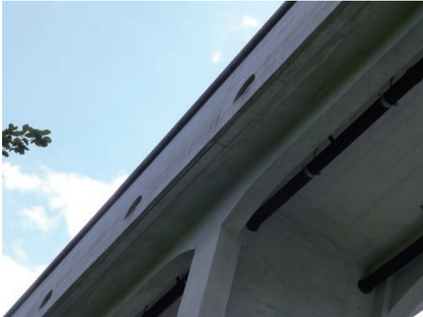
photo 33 Drainage holes viewed from off the bridge
