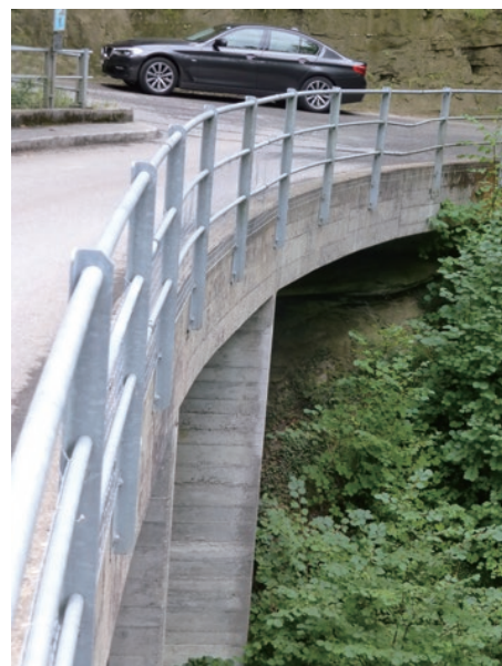
photo 16 Replacement of steel railings
