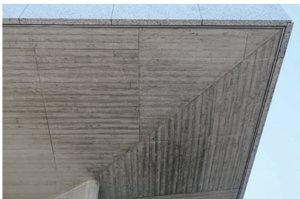
photo 6-2: Quasi-undressed concrete finished surface (which received its final coat in 2006)
