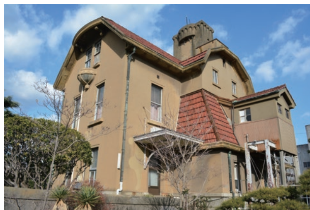
photo 2 Mikawa Family Residence (Important Cultural Property)
