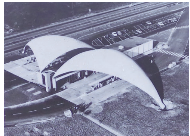
photo 56 Two-triangular concrete cupola roofs (cited from a photograph of a signboard installed on site)
