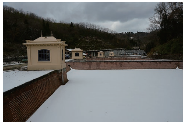
photo 4-2: Intake water control gate sheds
