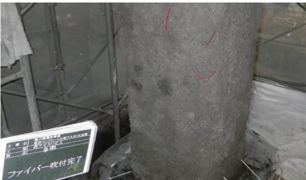
photo 7-3: Sprayed-on cellulose fibers (photo provided by : West Japan Railway Company)
