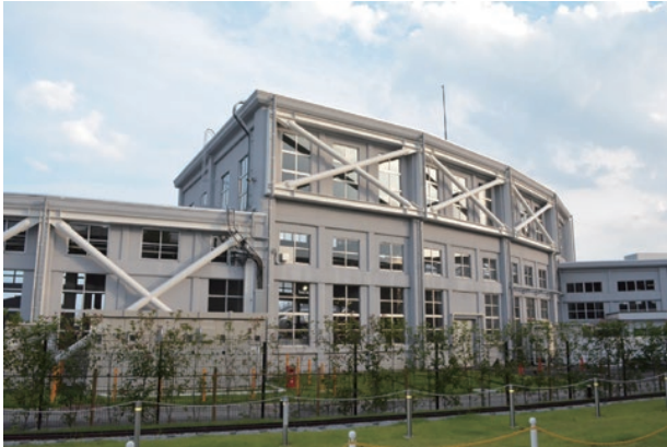
photo 6 Exterior, reinforcement with steel frame bracing
