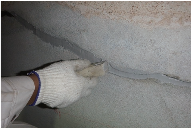
photo 5-5: Routing and sealing (photo provided by : Shimizu Corporation Hiroshima Branch)
