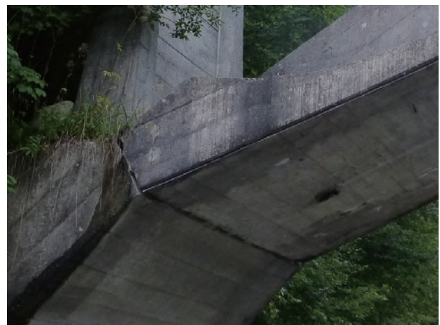
photo 10 Repaired hinge part of springing
