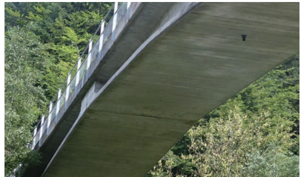
photo 9 Repaired hinge section
