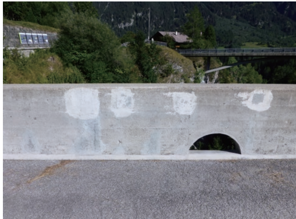
photo 45 Preventing rainwater from splashing over the outside of the bridge
