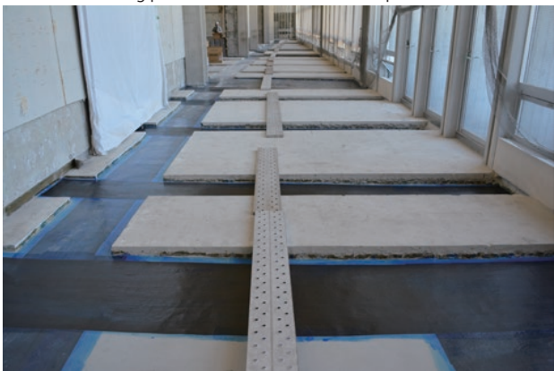
photo 20 Reinforcement of second floor upper surfaces with carbon fiber
