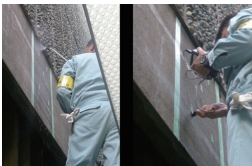
photo 11 Water repellency test on the concrete surface
