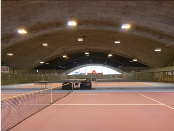
photo 52 Interior view of the shell roof design
