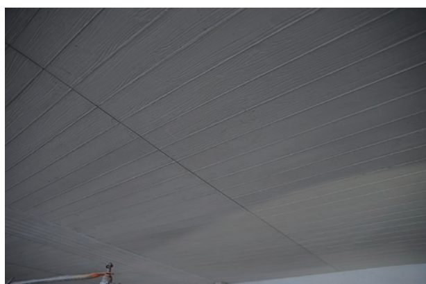
photo 6-5: Completed quasi-undressed concrete finish
