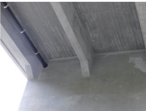
photo 21 Retrofitted drainpipe (1)
