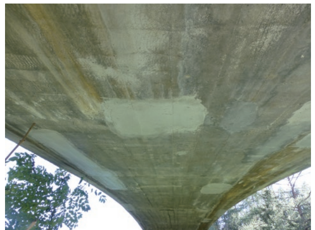
photo 49 Repaired spandrel wall bottom surface
