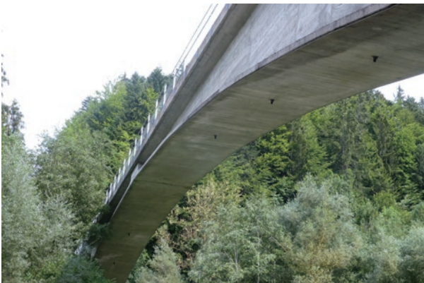
photo 4 Three drainpipes were provided at the bottom center of the arch.
