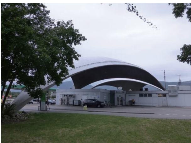
photo 59 Anchor of concrete shells
