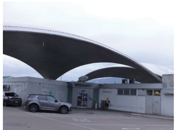
photo 55 Deitingen south service station concrete shell roofs
