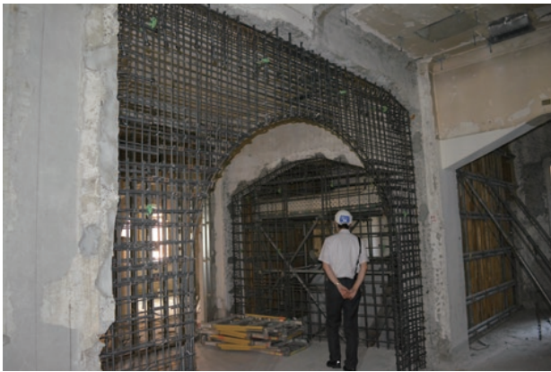
photo 24 Reinforced concrete anti-seismic wall, placement of reinforcement bars
