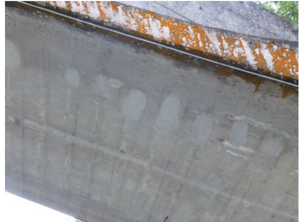
photo 8 Repaired arch ring (There is not much difference in color between the concrete used for the repair and the original structure. Water dams were installed on the side edges of the arch ring.)
