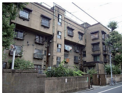
photo 1 Dojunkai Uenoshita Apartment Building
