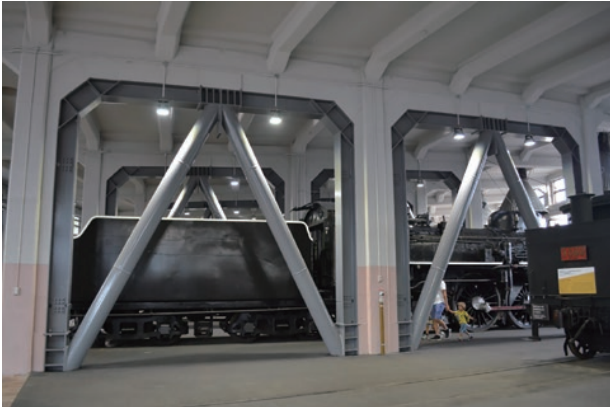
photo 5 Interior, reinforcement with steel frame bracing
