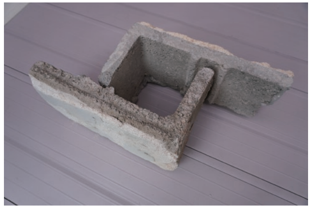
photo 9 Chin blocks acquired at the time of dismantlement of Suma Church
