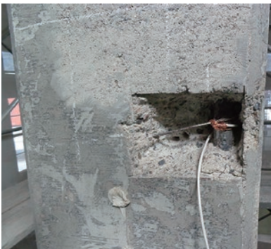
photo 7-1: Internal electrode set up inside the concrete (photo provided by : West Japan Railway Company)
