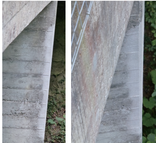
photo 15 Repaired spandrel wall
