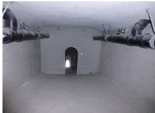
photo 35 Arrangement of drainpipes inside the girder
