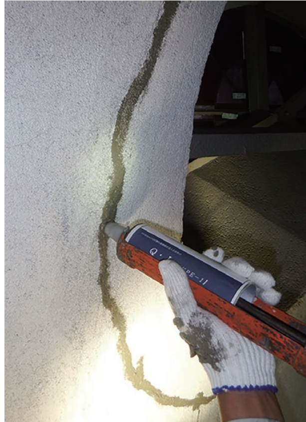
photo 5-4: Injecting ultra-fine polymer cement (photo provided by : Shimizu Corporation Hiroshima Branch)
