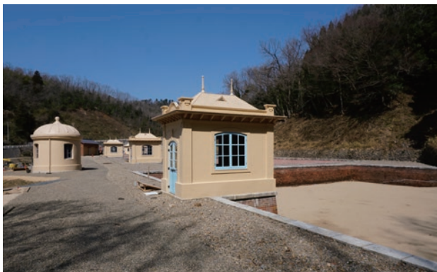
photo 1 Water control shed No. 5 (rectangular plan, in center) on the edge of filtration pond (right). Wells No. 4 and No. 3 can be seen toward the back. On left is the shed of Junction Well (circular plan) after restoration.
