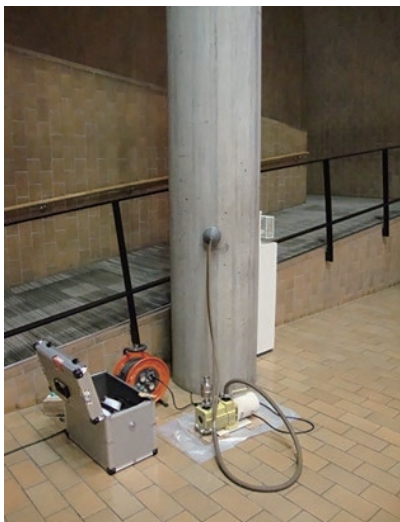
photo 9 Air-permeability test for the estimation of carbonation
