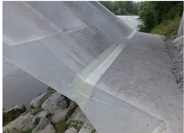
photo 24 Repaired hinge
