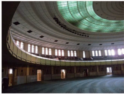
Ceiling from below
