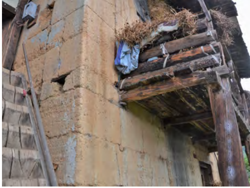
Low height layers of the rammed earth wall
