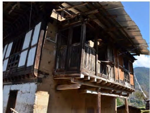
Overhanging section on the south of the second floor
