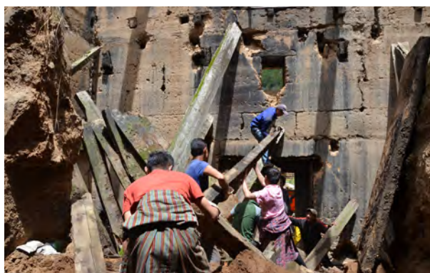
Removing collapsed wooden members from the building
