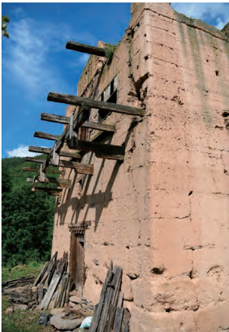
Condition of the rammed earth walls (front corner section)
