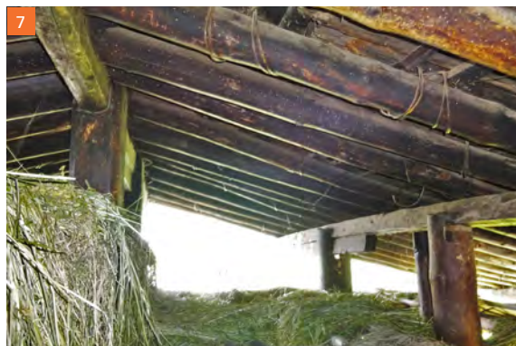
7 Ridge struts (rectangular, on the left) and other roof struts (round, on the right)
