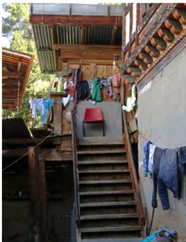
Stairway on the out side of the front
