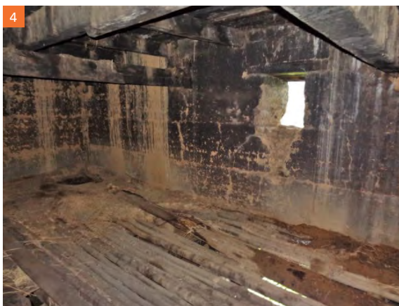
4 West room on the first floor
