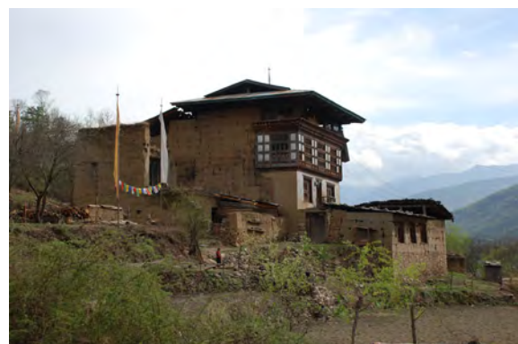
Traditional house enclosure and surrounding structures (Doteng, Paro Dzongkhag)
