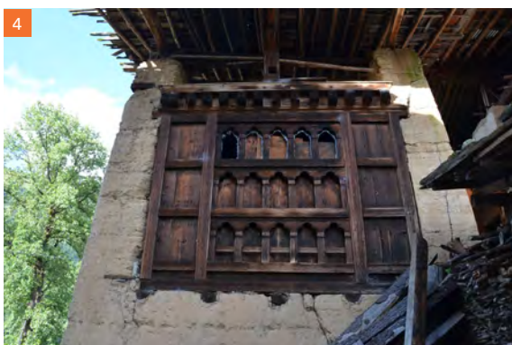
4 Details of the rabse window on the west wall
