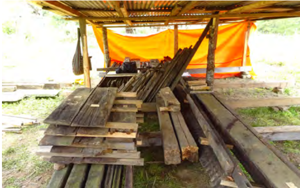
Salvaged members stored inside the temporary shelter
