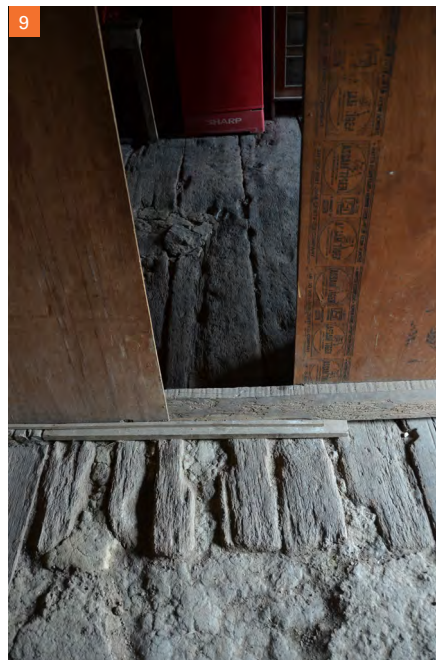
7 Altar room on the south side of the second floor 8 Attic space 9 Floorboards crossing under the plywood wall on the first floor
