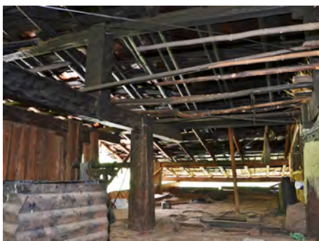
Roof structure extended to the extension section
