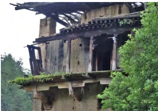
Lham Pelzom House, Details of the west façade in June 2013
