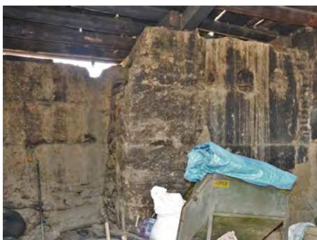
Rammed earth wall in the southwest corner of the earlier building
