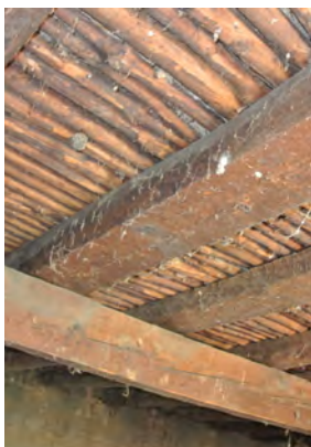
Fascine of the ceiling on the ground floor
