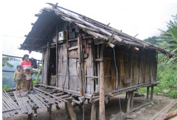
Traditional house built out of organic materials (Ramtoe, Samtse Dzongkhag)
