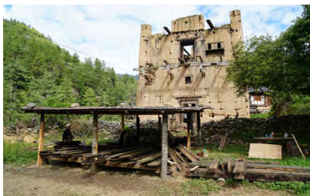
Temporary shelter for the storage of salvaged wooden members built in front of the house
