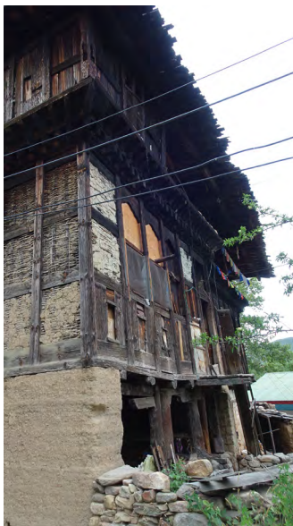
Details of the west façade (from north)
