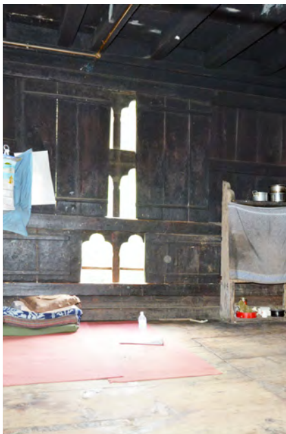
Rabsel on the east side of the living room on the first floor
