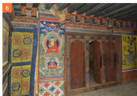
4 Stairwell on the second floor 5 Living room on the second floor 6 Altar room on the second floor
