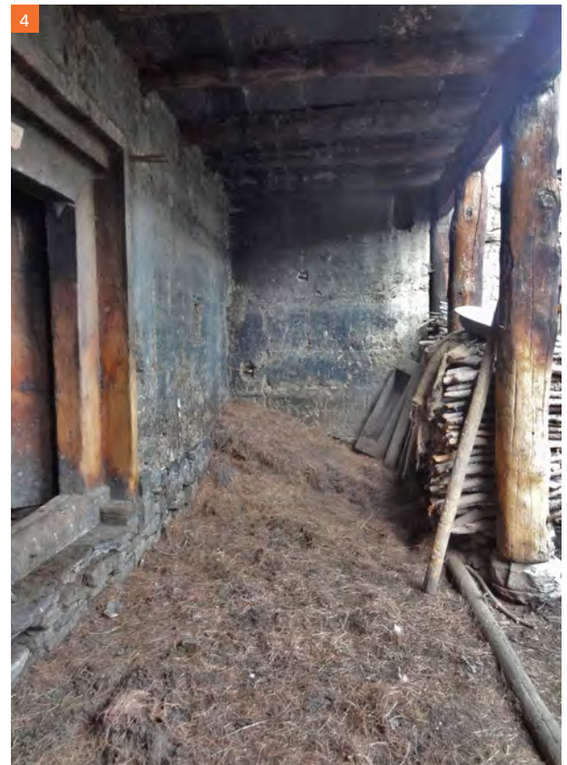
4 Front space of the entrance on the ground floor
