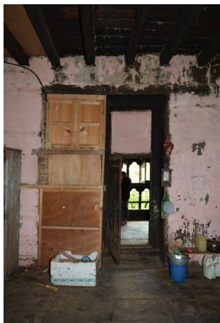
Modification of the opening between the room on the first floor
