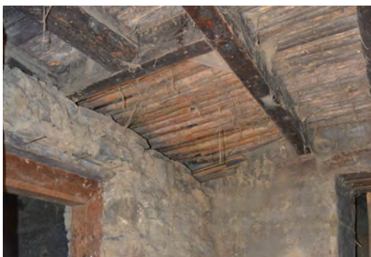
Traces of the opening in the first floor viewed from below
