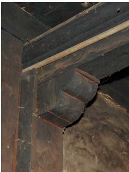
Molding under the beam and a bracket with carving
