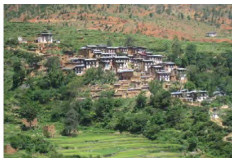
Different categories of built heritage Above left: Dzong, Above right: Lhakhang, Below left: Traditional houses, Below right: Cultural landscape
