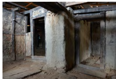
Wooden partition and rammed earth wall on the second floor
