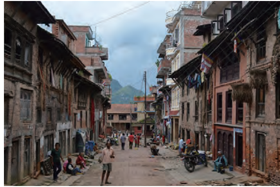
Fig. 2-6-9 View from the centre of the street (bldg.S15) to the east, on the 2nd August 2014 (photographer: DNT)
