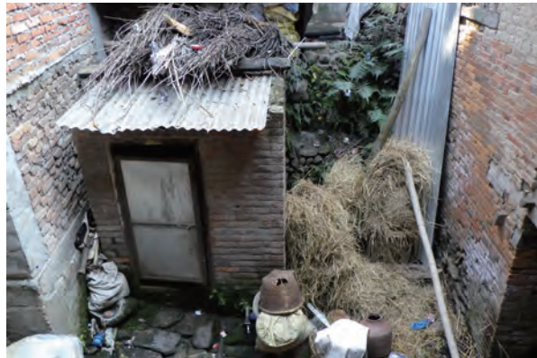
Fig. 2-6-22 Installation of common lavatory in the courtyard (S15, rear side)
