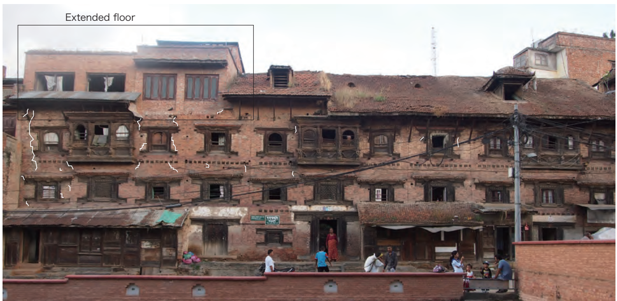
Fig. 4-2-3 Cracks are seen on the left side, under the extended floor more than right side where traditional roof style remains (Kirtipur), taken by author on 18th Sep. 2015
