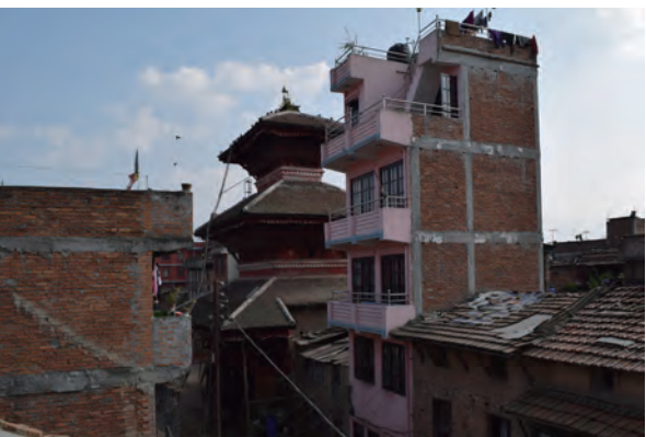
Fig. 4-2-12 water storage tank of the house (S17) was falled and damaged the roof of low-rise house (S18)
