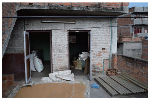
Fig. 2-6-24 Drying cereals in the sun on the roof floor (N13)
