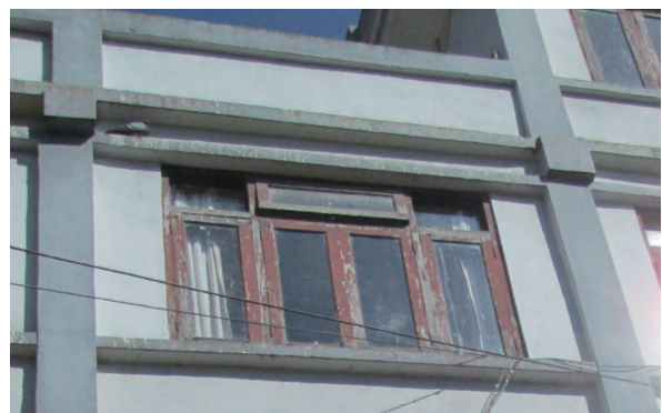
Modern window of b. Personalized type house
