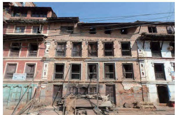
Fig. 4-2-24 Extension at the fourth floor
