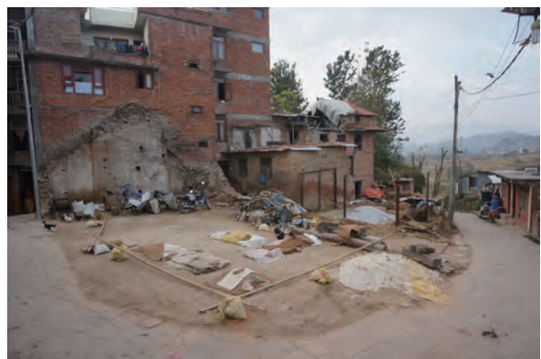
Fig. 2-5-5 Nhyabu Mill (Collapsed)
