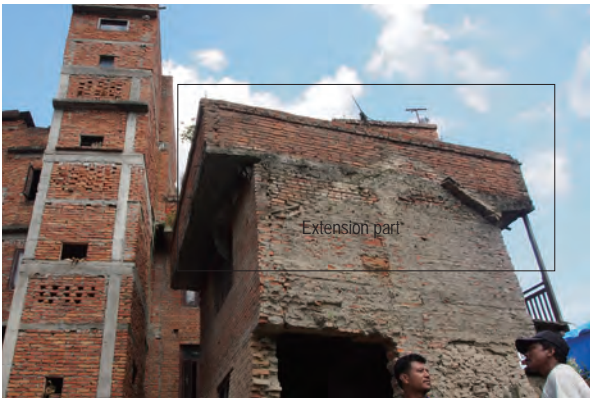
Fig. 4-2-6 Example of extension of brick and reinforced concrete on the brick house (An example from outside of the investigated site)
