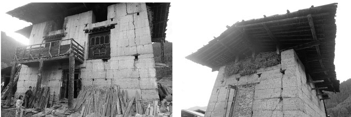
Photo 7.,8. Phub Lam house, front view (left), side and back (right)
