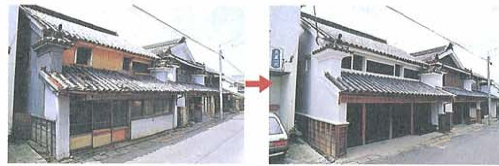
Repair of a historic building (Machiya) at Miramimachi, Waki-machi
