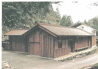
Facilitating a water tank for fire protection at Omoriginzan, Oda-shi
