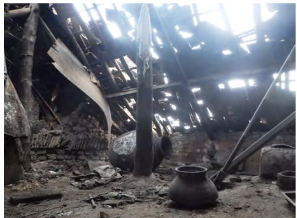
Fig. 2-6-31 Inside of traditional house kitchen. Tiled roof is posted over low walls of 60cm high. (N05)
