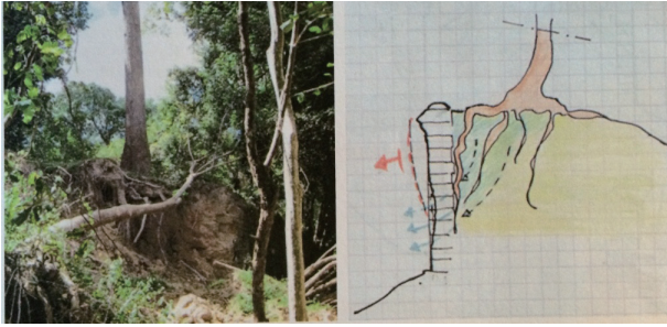
Fig.10 樹根の影響 Effect of the tree root
