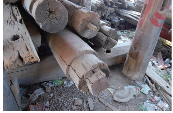
Ph.16 Square and round tenons on top of the pillars (abandoned members of a monastic building in Bagan)
