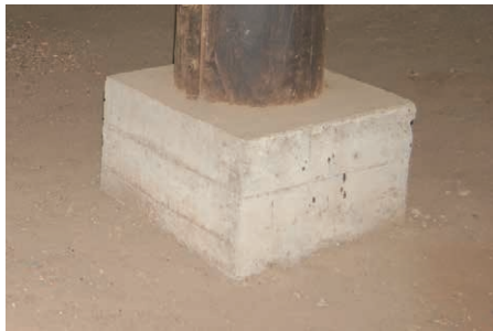
Ph.44 RC foundation at the bottom of a pillar
