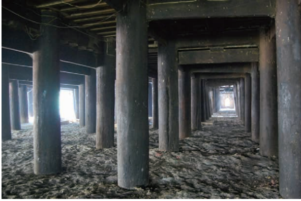
Ph.15 Below the floor of Bagaya monastery, Innwa (bay under the ridgepole on the right)
