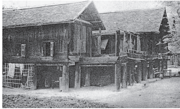
Note: Only one door for loading and unloading. A unique door for a Kye, 4 feet wide up to the header height, the opening is closed & opened by sliding a heavy duty plank generally 4 1/2 ft. X 8 inches, 2 inch thick planks are slid down one at a time between two columns preventing the paddy from spilling out. Mud platform to dry paddy./Ta linn.
