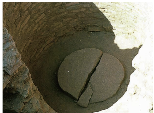
Ph.23 Foundation stone possibly for supporting a pillar (S. Fraiser-Lu, Splendour in Wood, Bangkok, 2001)
