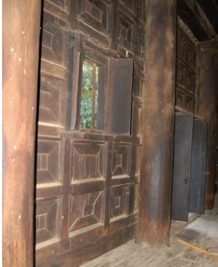
Ph.26 The inside of the exterior wall (Bagaya monastery, Innwa)
