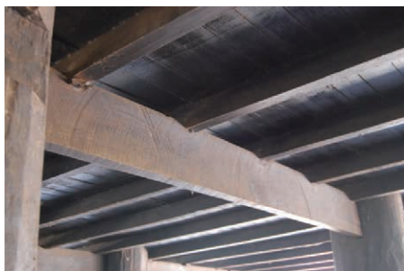
Ph.45 Joints between floor joists and a tie beam
