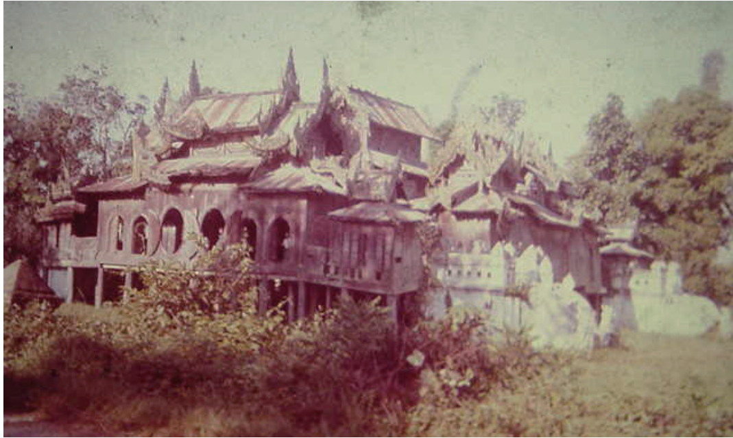
This is the photo taken in 1968 by the author. The 'building' is in ruins falling apart, floor line and columns are out of plumb and some embellishments of excellent arts & crafts work have disappeared. However it was still occupied by the Sayadaw! The roof embellishments and at the eaves are slightly different from the Kon Baung Period Monastery, and the oval openings appears to have nothern influence!
