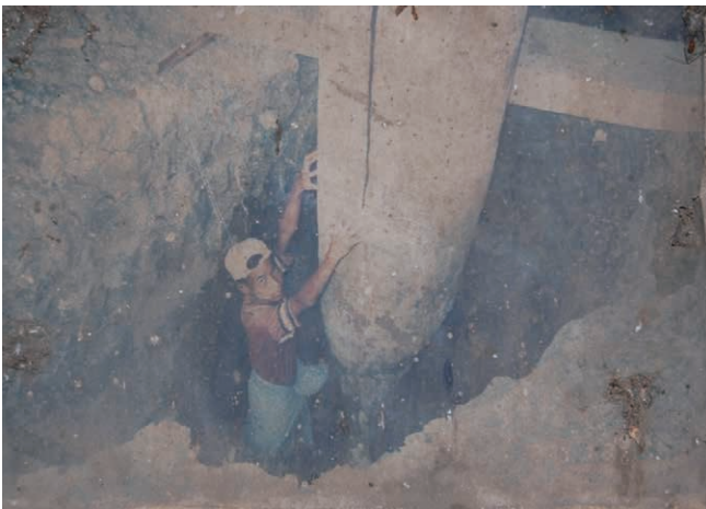
Ph.14 An earthfast pillar at Mindin monastery (old photo during the restoration)
