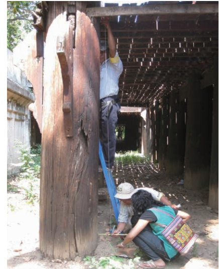
Ph.1 Training on the preservation of historical wooden buildings (Innwa)
