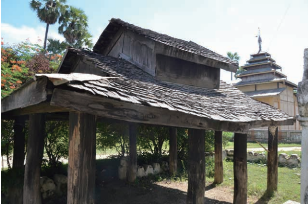
Ph.36 Roofs with overlapping shingles (Pakhanngge monastery)
