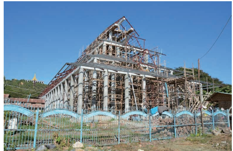
Ph.46 Royal shrine under reconstruction with RC structure
