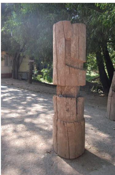
Ph.17 Mortise and dado at the upper section of a pillar
