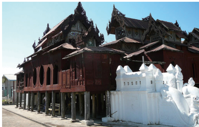
Shwe Yan Pye after Repairs 'Renovation and Presentation'
