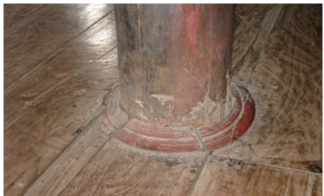
Ph.29 Column pedestal on the floor (Shwenandaw monastery)
