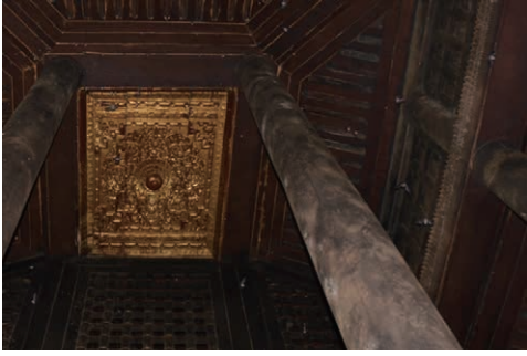
Ph.24 Abrasion marks on the upper part of a pillar (Bagaya monastery, Innwa)
