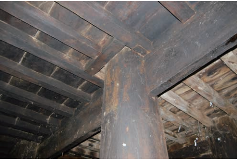
Ph.25 Floor structure seen from the below (Bagaya monastery, Innwa)
