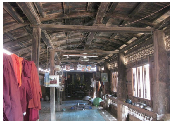
Ph.35 Example of a convex curved roof (a secondary building at Yok-son monastery, Sale)
