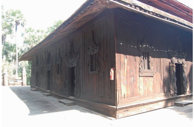
Ph.27 The outside of the exterior wall (Bagaya monastery, Innwa)
