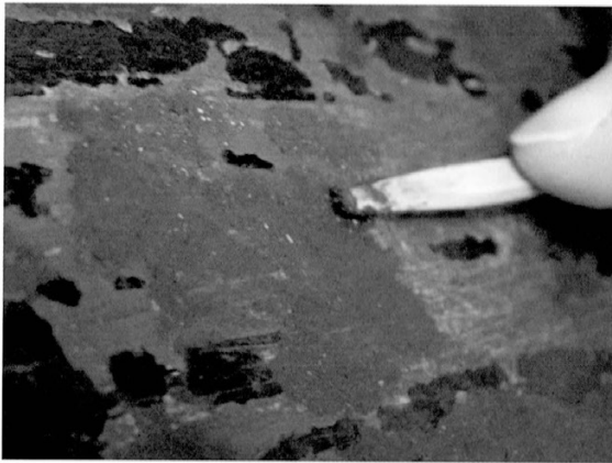
Fig. 9.18 底面破損部の刻苧付け Applying kokuso to the damaged part on the bottom of the box
