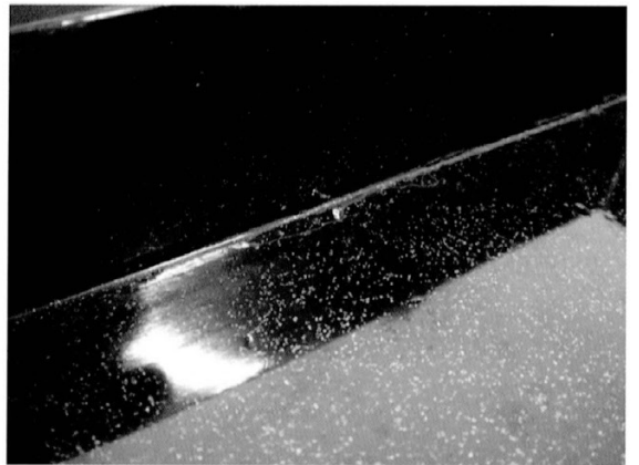
b 修復後 After restoration
