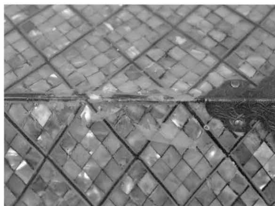
a 修復前 Before restoration
