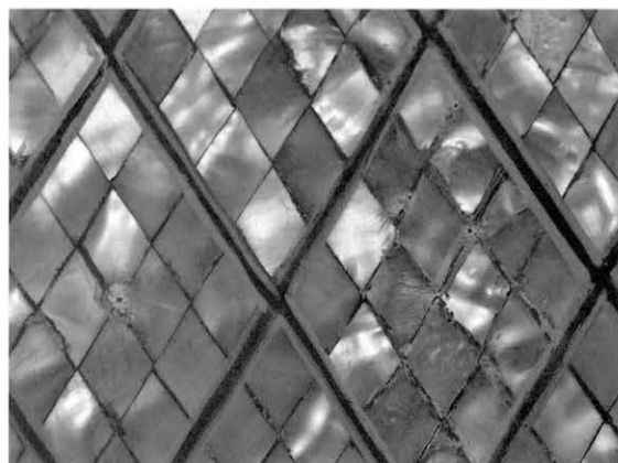
a 修復前 Before restoration
