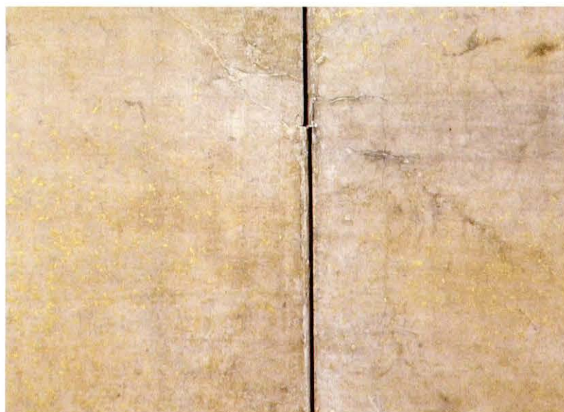
b 修復後 After restoration
