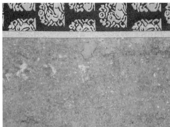
b 修復後 After restoration
