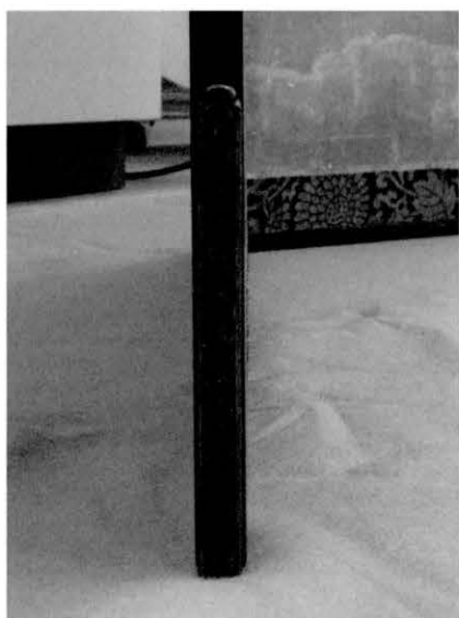
a 修復前 Before restoration
