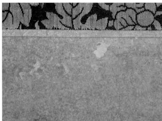
a 修復前 Before restoration
