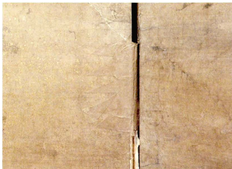
a 修復前 Before restoration
