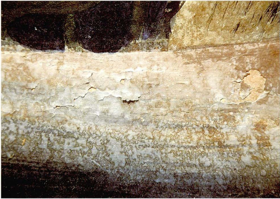
a 修復前 Before restoration
