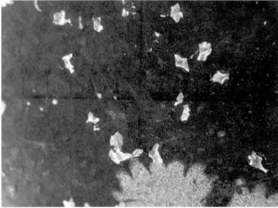
図7 塗膜劣化 (× 20) Fig. 7 Deteriorated coating film (x 20)
