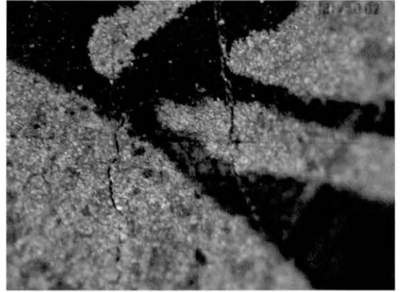
図8 塗膜劣化、亀裂 (× 20) Fig. 8 Deteriorated coating film, crack (x 20)
