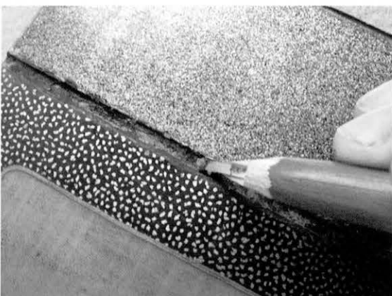
図18 後補接着剤 除去 Fig. 18 Removal of the adhesive agent of a past restoration
