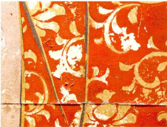
(3)-1 修復前 絵具の剥離・嵩腫部 Before treatment: flaking and lifting of paint pigment
