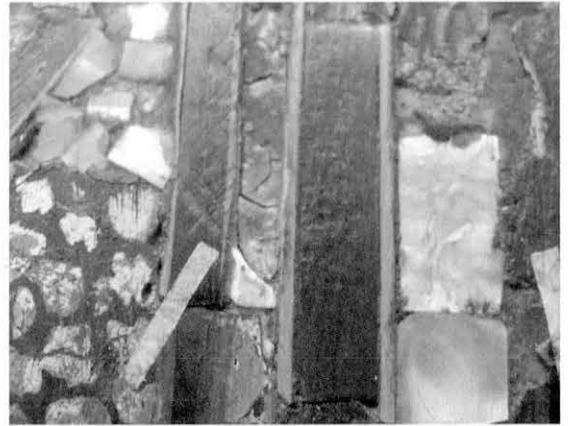
木象嵌による修復 拡大 Restoration in Europe by inlaying wood, enlarged, 2006
