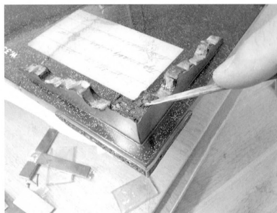
図21 接着用刻苧の充填 Fig. 21 Filling with kokuso for adhesion
