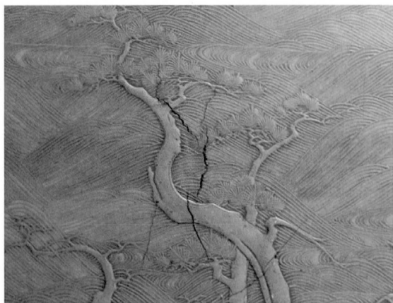
図45 修復前（亀裂部分） Fig. 45 Before restoration (cracked portion)
