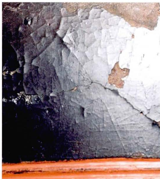
3 修理前 Before restoration
