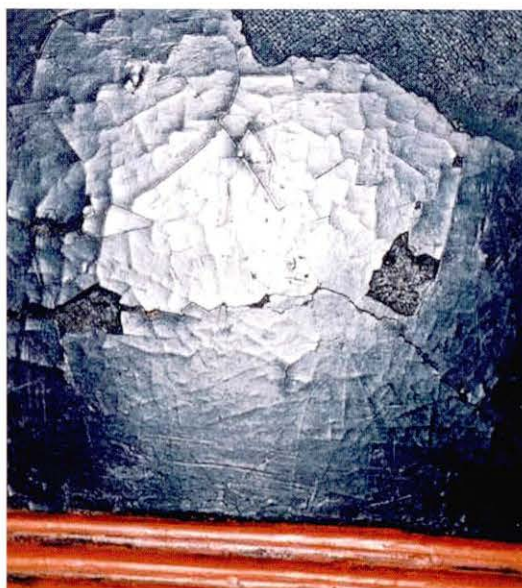
4 修理後 After restoration
