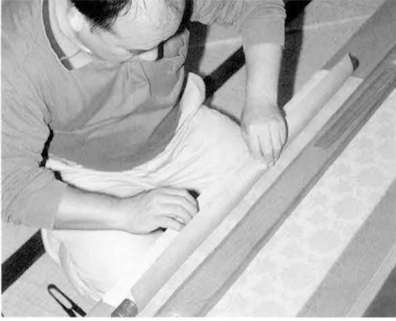
188 仕上げ Finishing work
