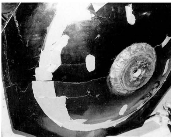
図63 屋蓋の解体の前に塗膜を養生する Protection of the urushi coating of the roof before disassembly
