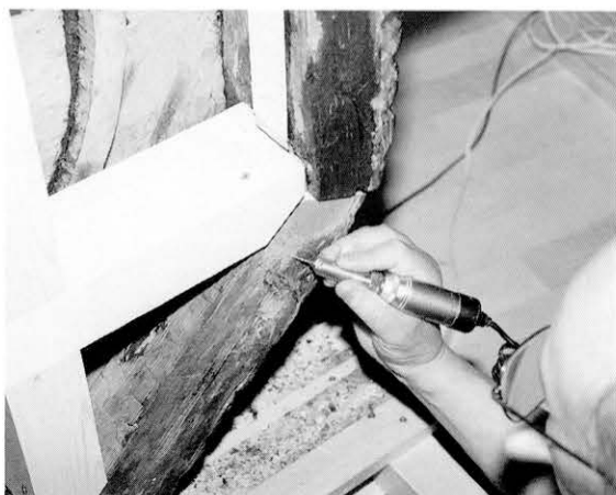
図103 木屎表面の研磨 Polishing the surface of kokuso
