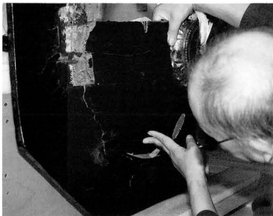
図65 屋蓋の塗膜の剝離解体作業 Removing the urushi coating on the roof
