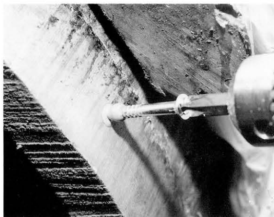
図80 真鍮製の木ネジ Brass screw
