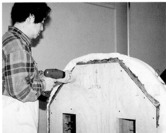
図49 解体のため底部合板を外す Taking off the plywood board in disassembly
