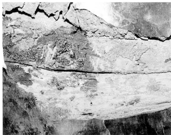
図68 塗膜を剥がした後の屋蓋の素地の状態 Condition of the substrate of the roof after the urushi coating was removed
