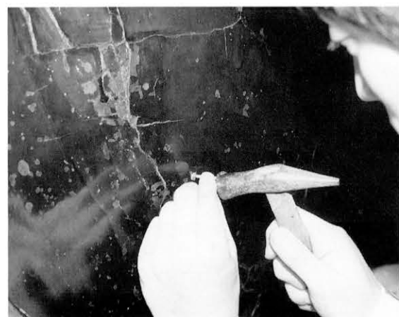
図94 木釘の打込み Driving wooden nails
