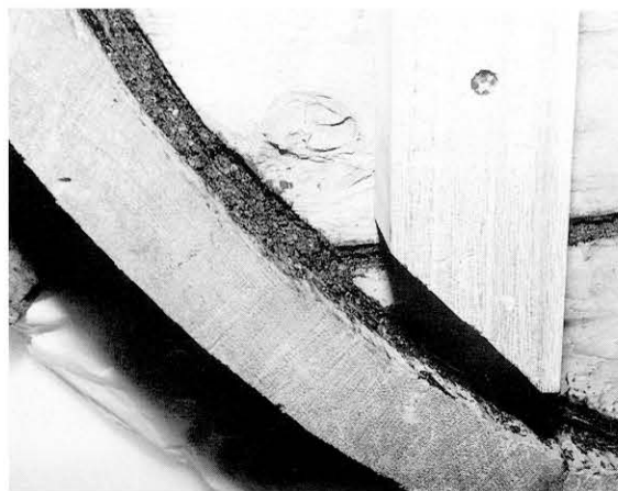
図82 木屑漆を充填 Filling kokuso to the base
