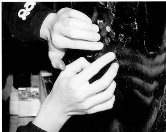
図95 剝離した塗膜を麦漆で貼りつける Re-fixing exfoliated coating film
