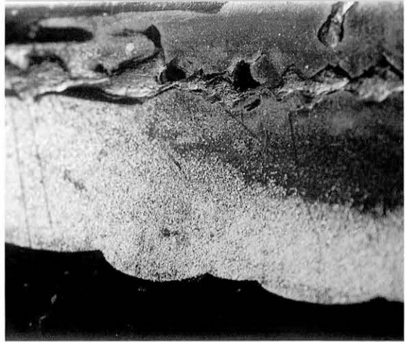
67 同 (修理後) Foundation applied in the past treatment (after restoration)
