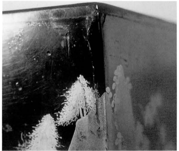
73 同 (修理後) Proper right back top corner (after restoration)
