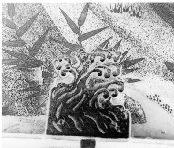
80 波形の金具正面扉左下 (修理前) Metal fitting (before restoration)
