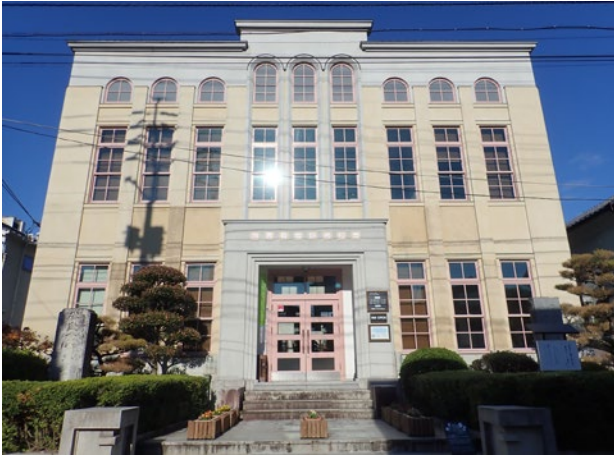
Photo visitor center (former Uchiko police station)
