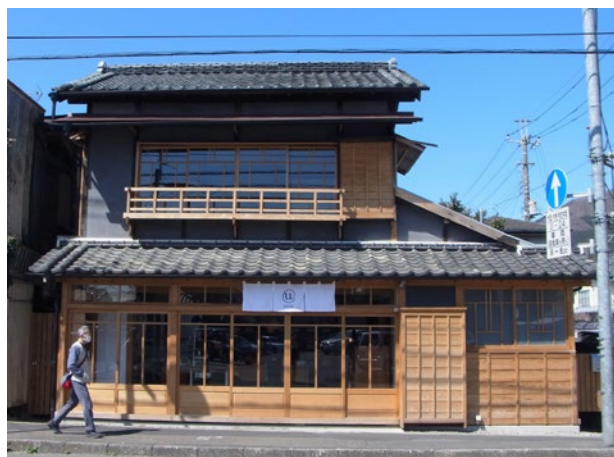
Photo 11 com+position (Former Hasegawa dye house)
