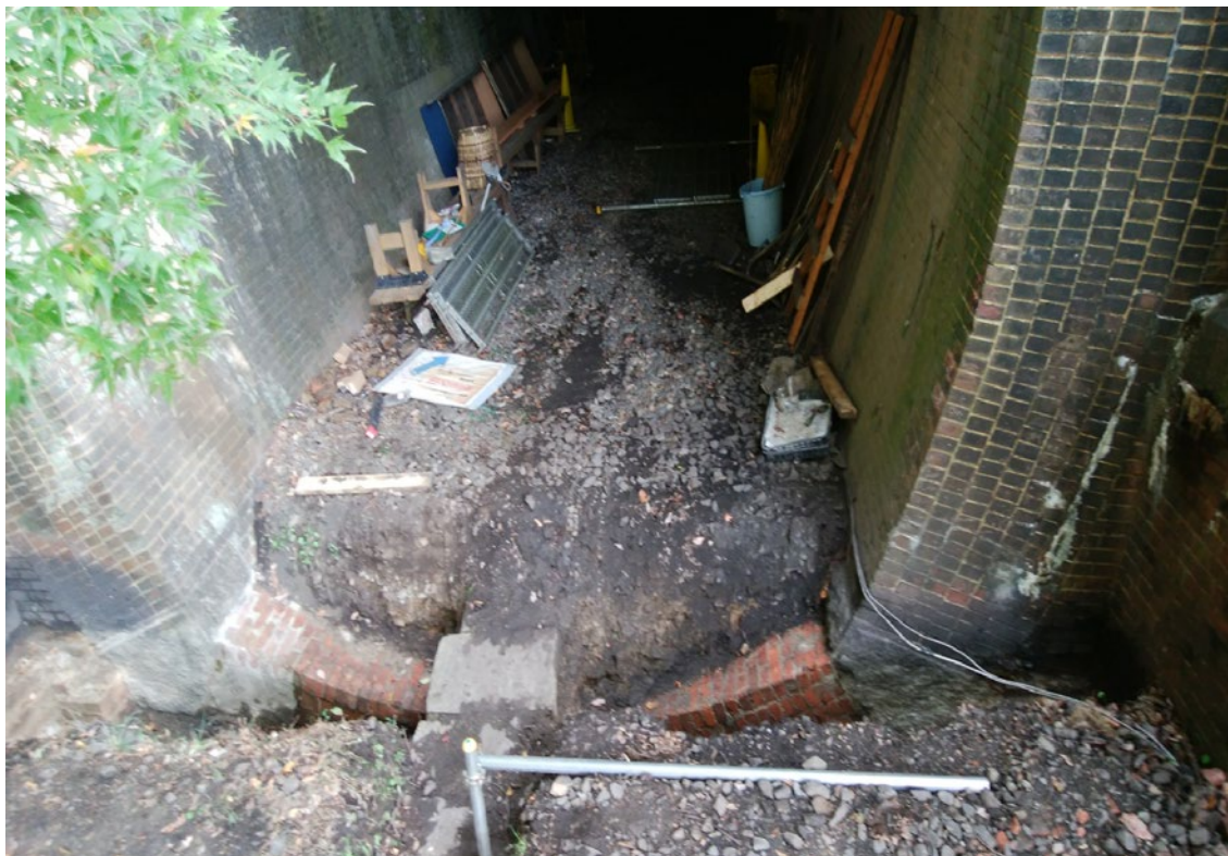
Photo 2 Invert excavation scene
