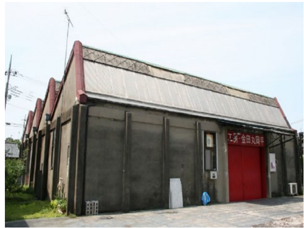
Photo 4 Saw roof factory (Former Kakei Goro's atelier)
