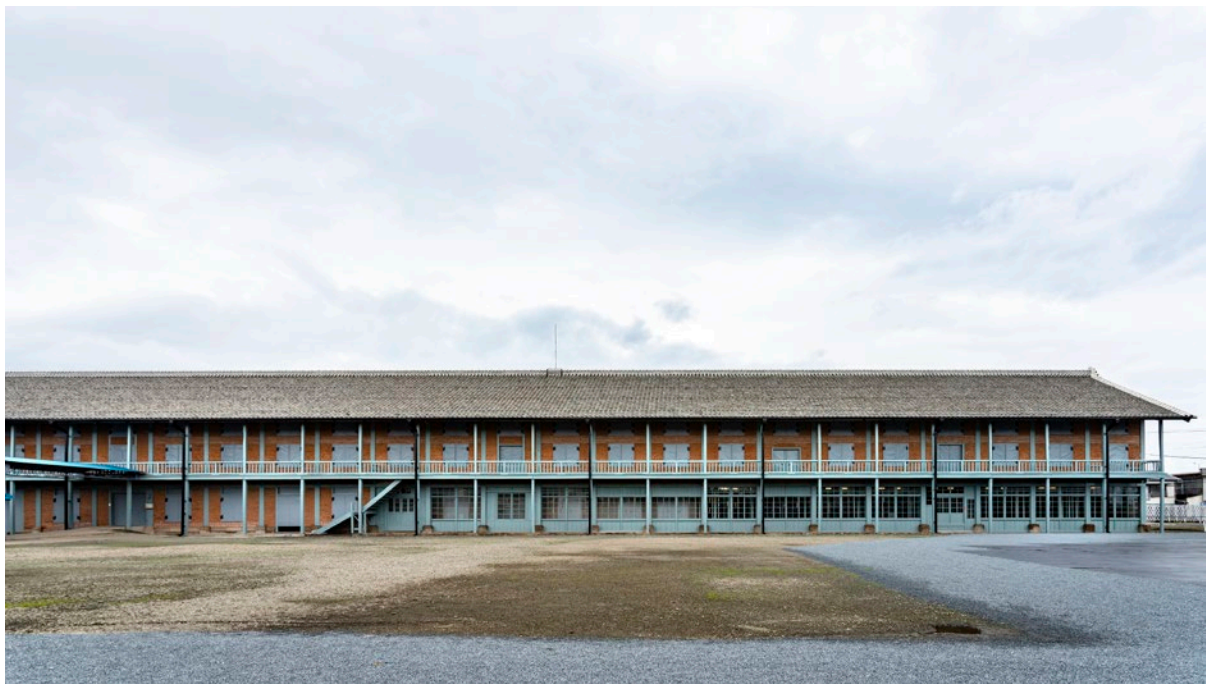
Photo 1 West Cocoon Warehouse, after repair / photo taken by : Sewaki Takeshi
