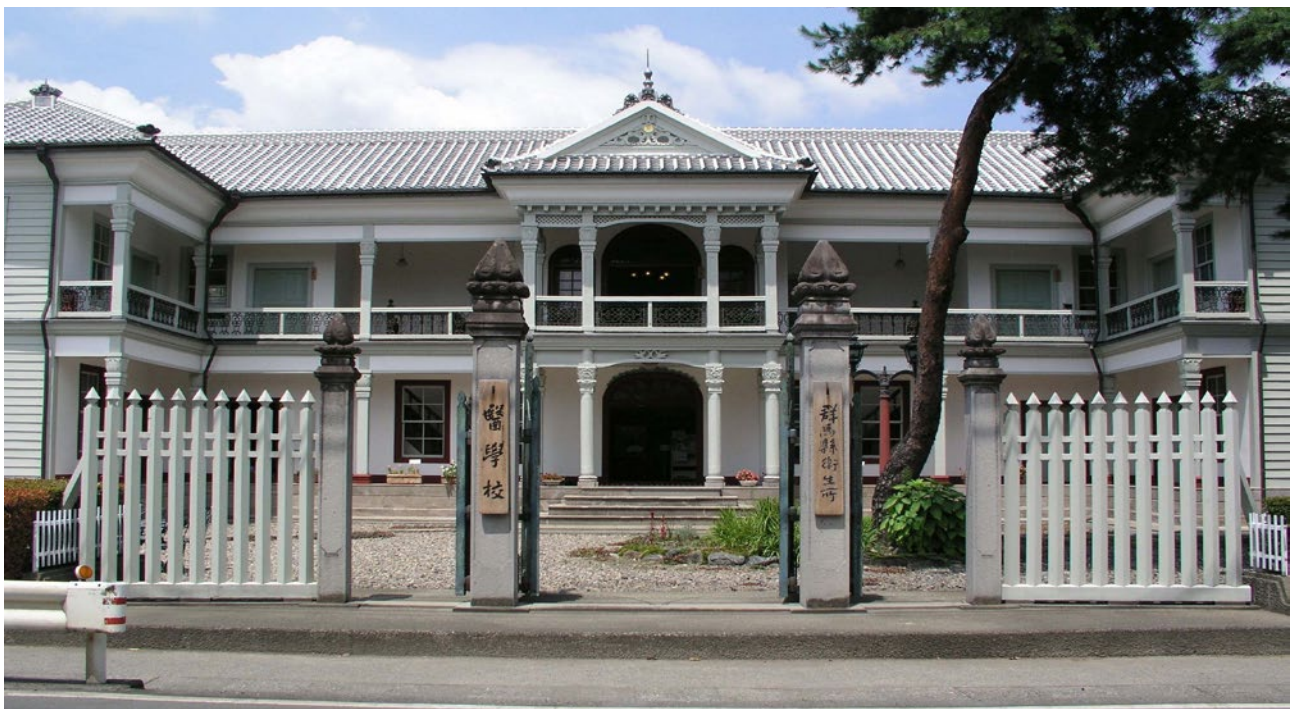
Photo 2 Kiryu Meijikan (Former Gunma Prefecture Sanitary Center, Important Cultural Property)
