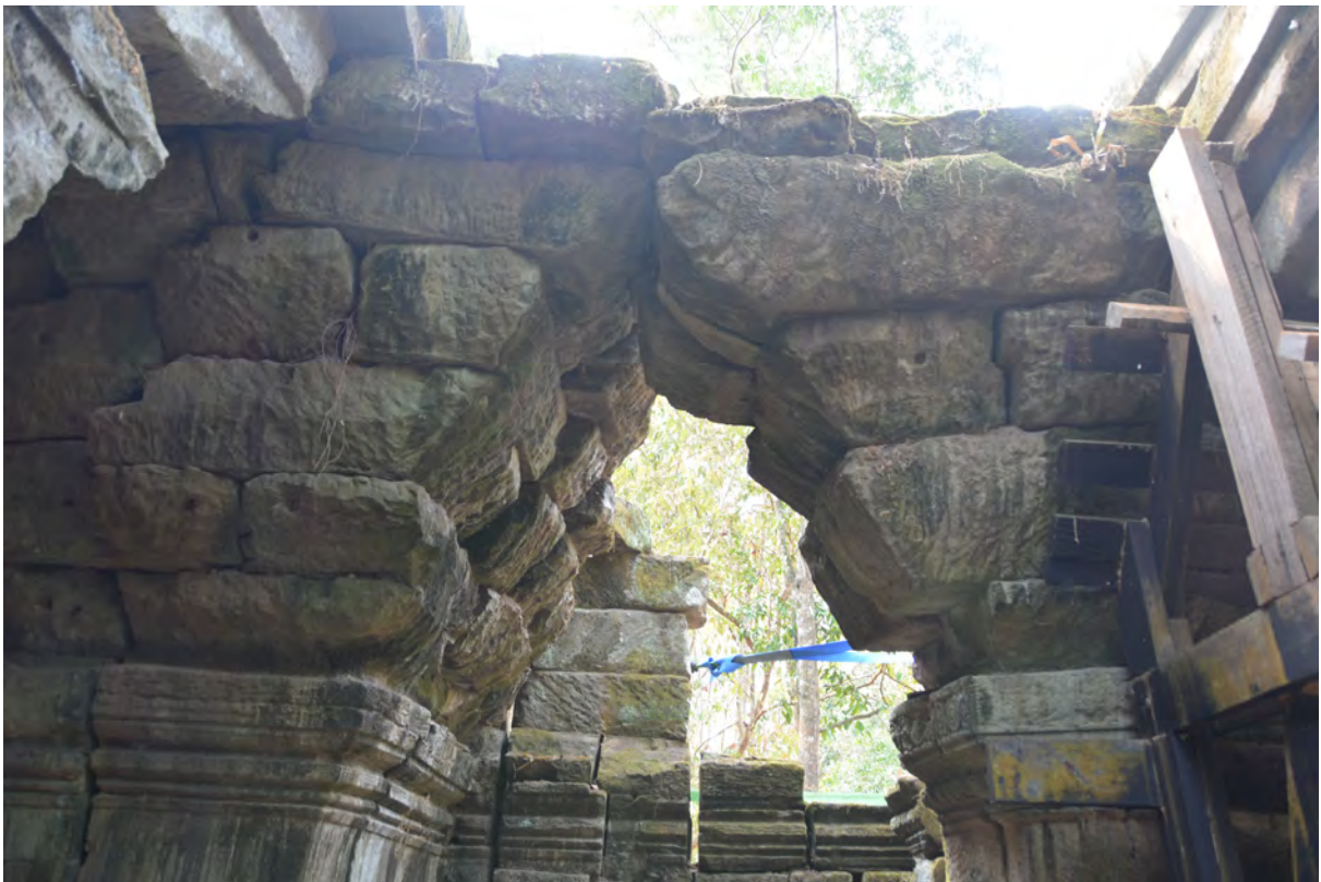
South ceiling before dismantlement in March, 2019
