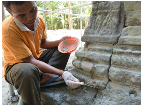
Figure 9.2.97 Retouching work with filling mortar
