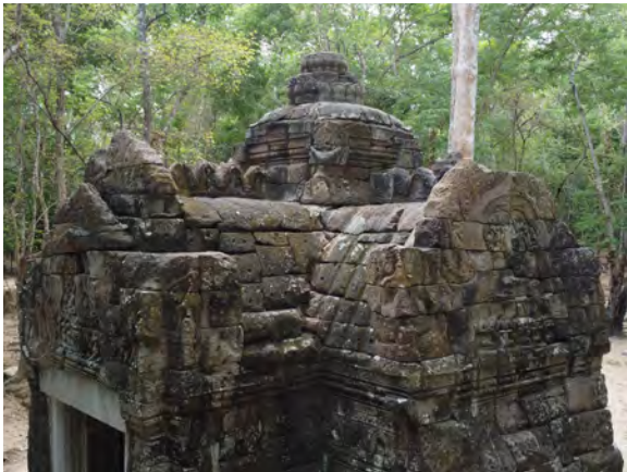
Figure 5.2.32 Difference in the construction method between the northern and eastern pediments
