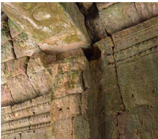
Figure 3.2.51 A trace of a wooden member at the causeway, Ta Som Temple
