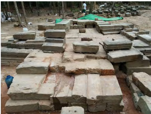
Figure 9.2.9 Work progress in May, 2020 (North view)
