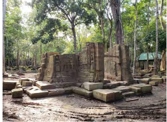
Figure 9.2.14 Work progress in September, 2020 (Southeast view)
