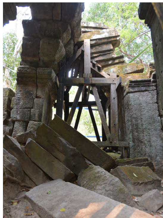
Figure 2.1.4 Inside the East Gate before restoration
