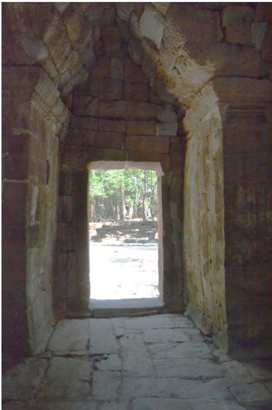
West inner elevation after restoration
