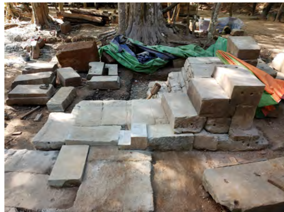
Figure 9.2.47 Use of sandstone fragments to fill gaps
