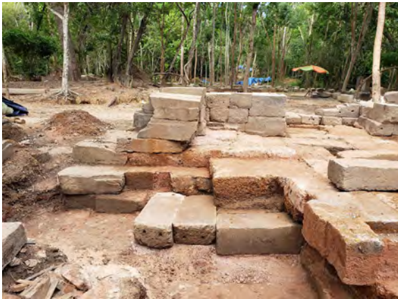
Figure 9.2.52 New substrate laterite on the west side of the north wing
