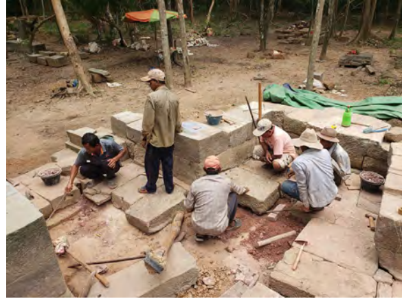
Figure 9.2.57 Use of lime mortar to adjust the floor level
