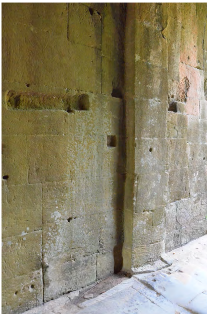
Figure 3.2.47 Traces of the wooden members at the causeway, Preah Khan Temple
