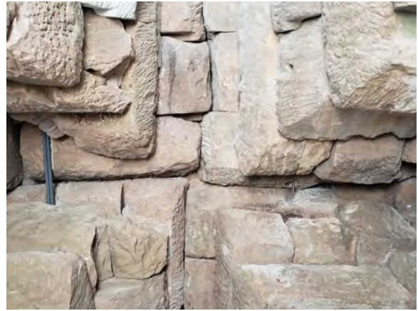
Figure 9.2.89 Interior view of the cross-vault structure
