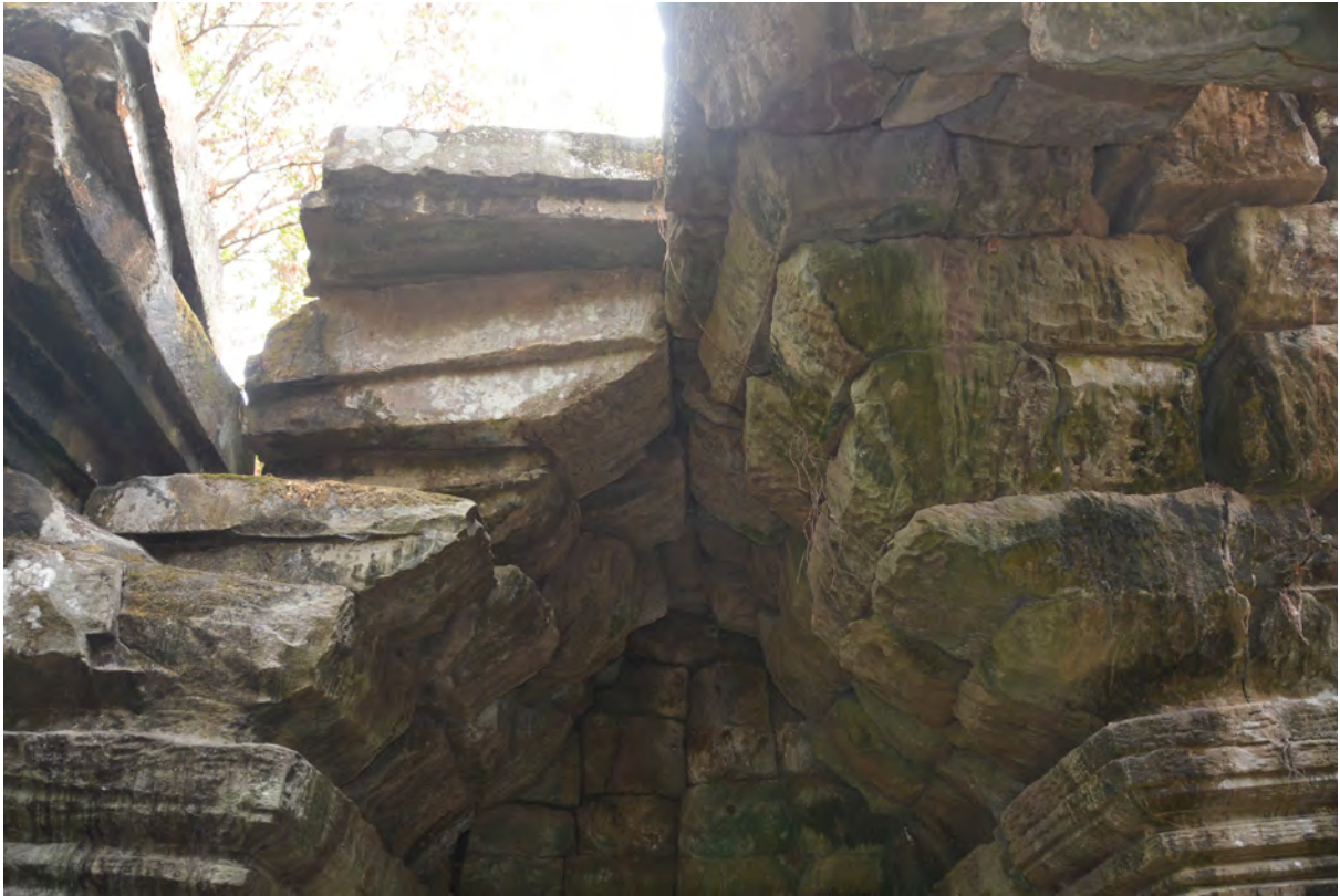
East ceiling before dismantlement in March, 2019
