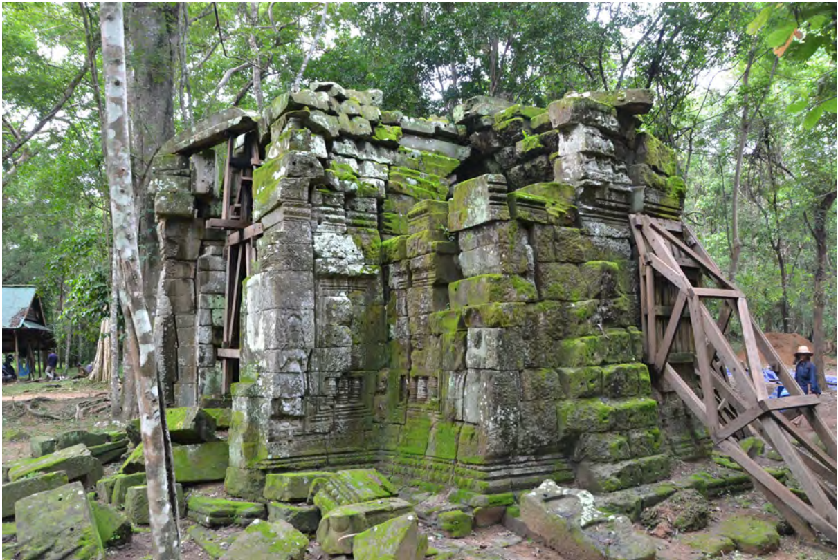
Southwest elevation before restoration in July, 2017
