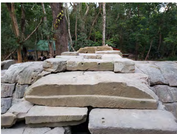
Figure 9.2.86 Sandstone at the top of the roof structure
