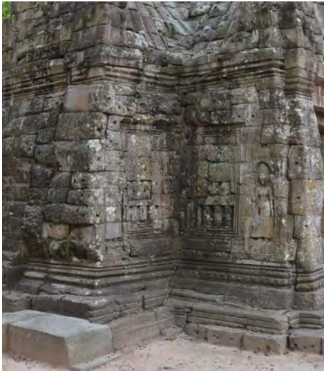
Figure 3.2.4 Internal corner of the East Gate
