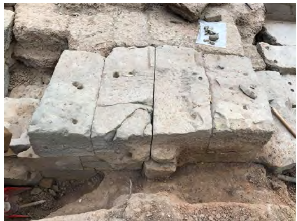
Figure 5.2.40 North side of the exterior sandstone of the East Gate's base structure, cut and processed to accommodate the 'Outermost Enclosure' base laterite
