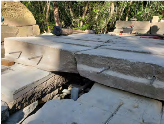
Figure 9.2.82 Consolidation of the cross-vault structure in the east-west direction
