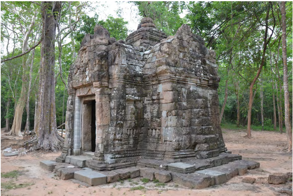
Southwest elevation after restoration
