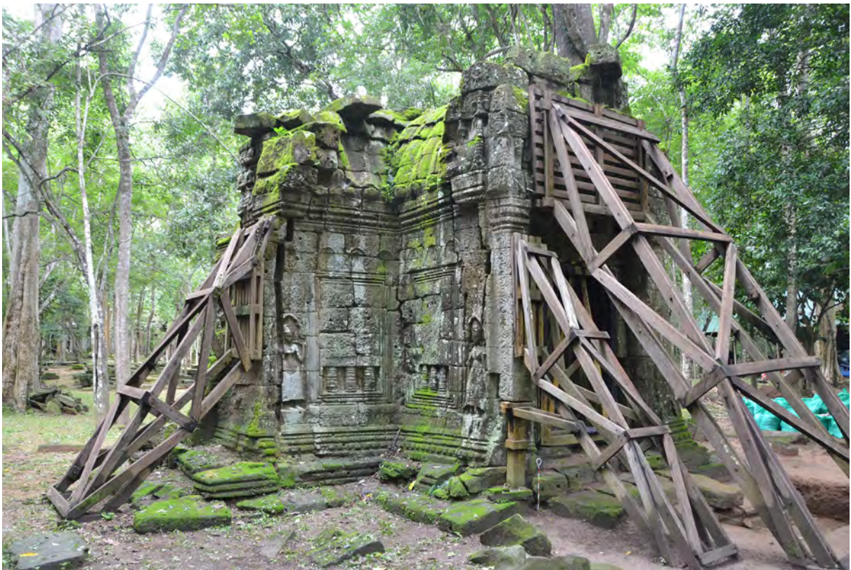
Southeast elevation before restoration in July, 2017
