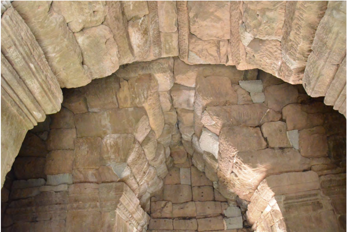
West side of the ceiling after restoration
