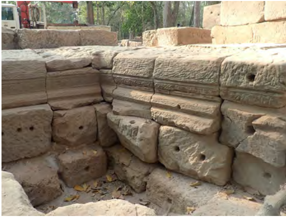
Figure 5.2.37 Engravings on the exterior sandstones, indicating the original ground level
