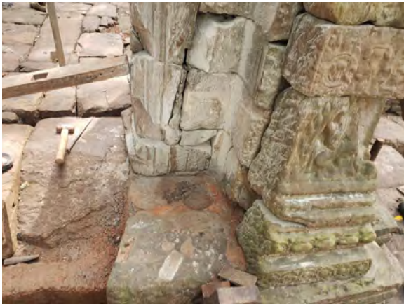
Figure 5.2.26 Circular mortise for a colonette in the southwestern corner
