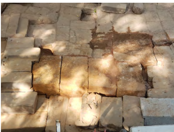
Figure 9.2.42 New laterite replacing deteriorated substrate laterite in the west wing
