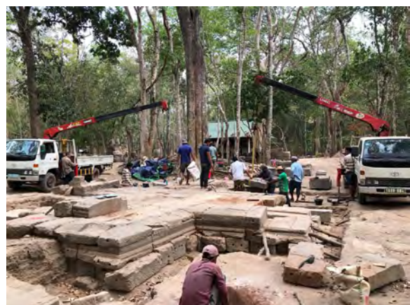
Figure 9.2.6 Work progress in April, 2020 (Southeast view)
