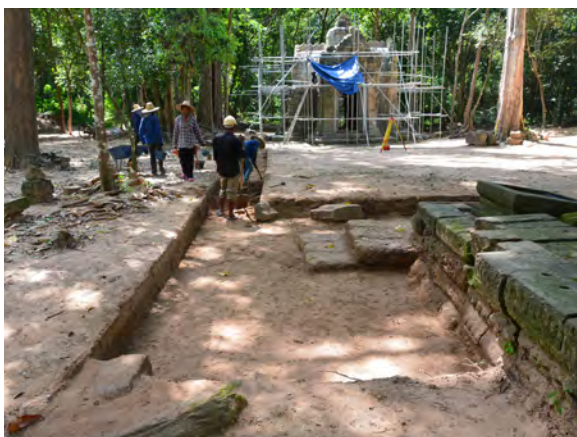
Figure 9.3.3 Digging the western drainage channel
