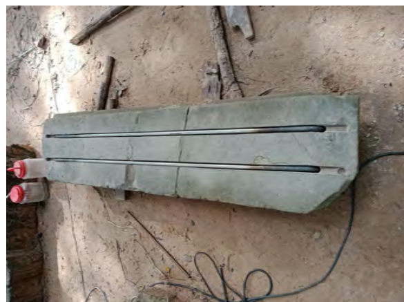
Figure 9.2.87 Repairing the topmost layer's roof sandstone
