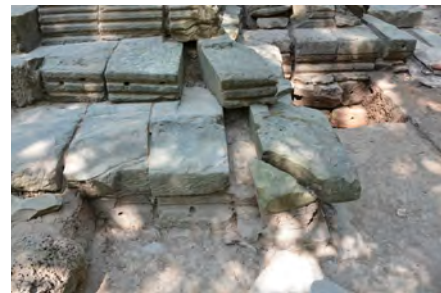
Figure 8.1.1 Displacement of the stones on the base structure's outer periphery
