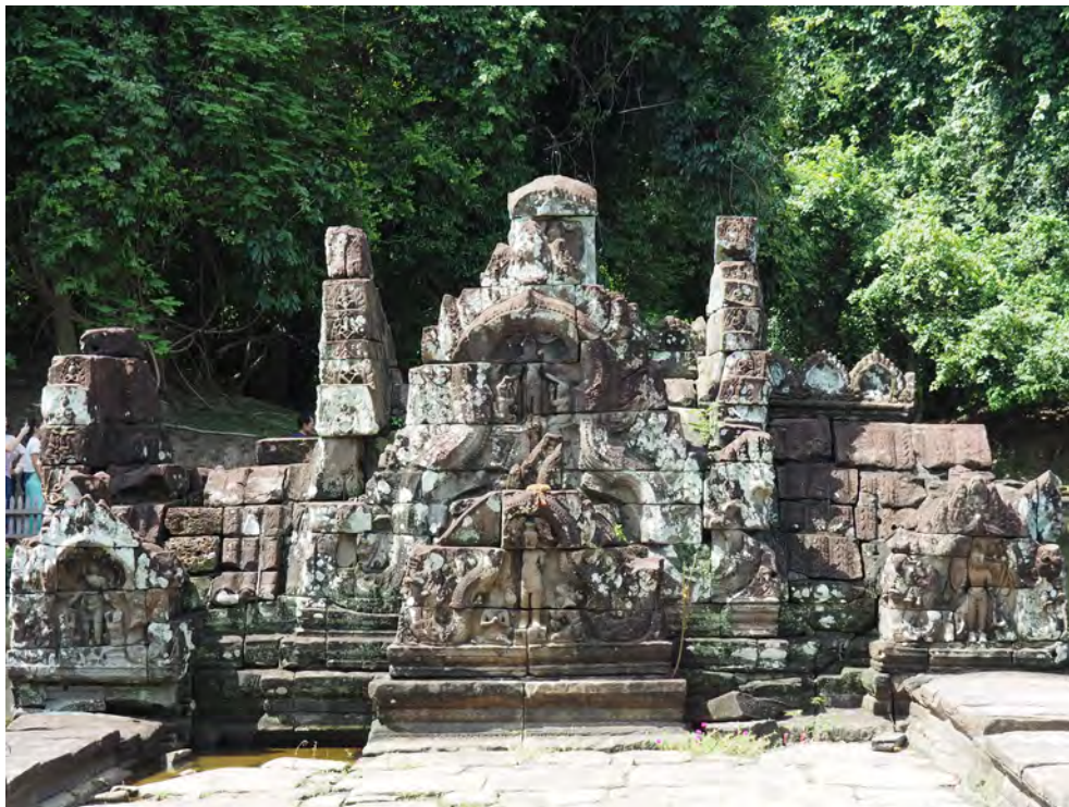
Figure 10.1.15 North pediment on the east secondary pool, Neak Pean
