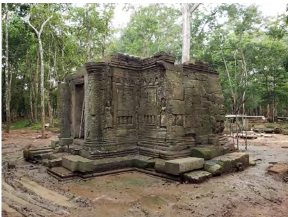
Figure 9.2.17 Work progress in October, 2020 (Northeast view)
