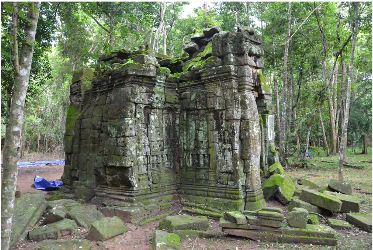
Northwest elevation before restoration in July, 2017
