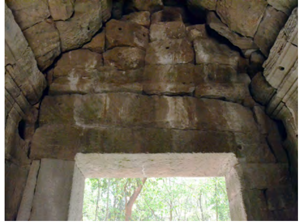
Figure 5.2.19 Traces of holes in the wall into which a wooden-horizontal member would have been inserted at the eastern entrance
