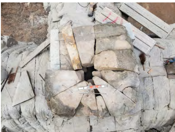
Figure 9.2.92 Reassembly of the finial
