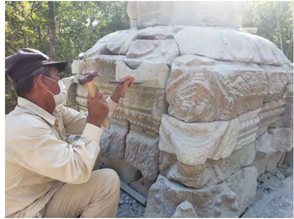
Figure 9.2.103 Engraving the finial's new stones
