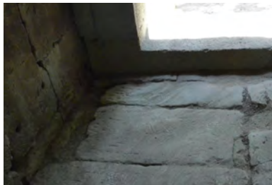
Figure 3.2.17 / Figure 3.2.18 Traces of the wooden members of the east entrance, East Gate
