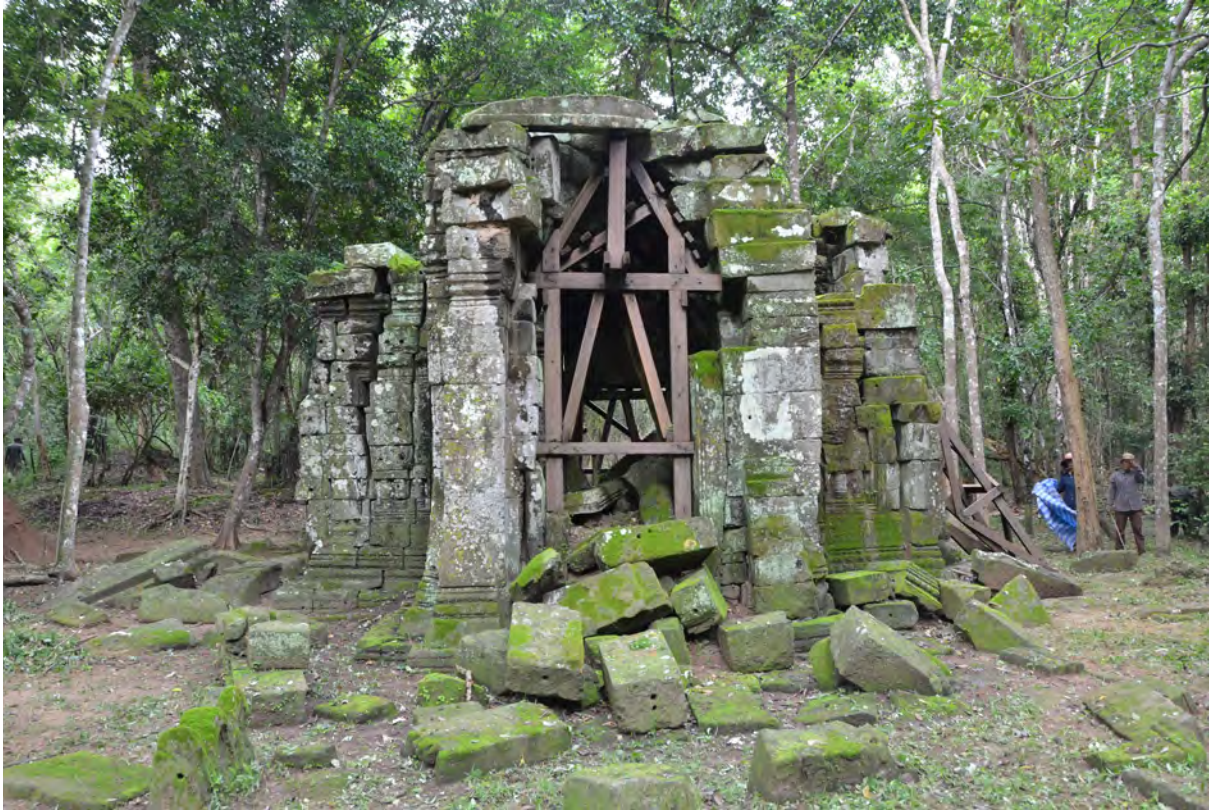
West elevation before restoration in July, 2017
