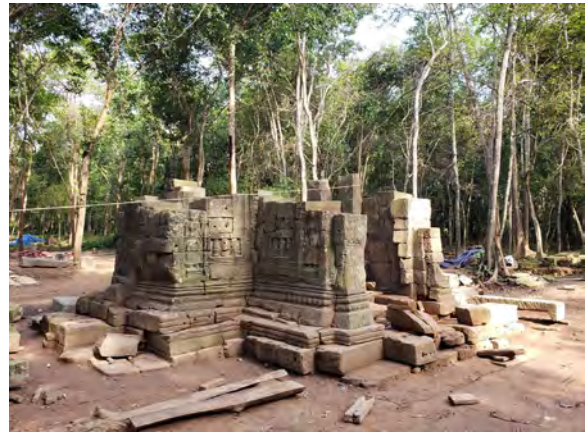
Figure 9.2.16 Work progress in September, 2020 (Northwest view)
