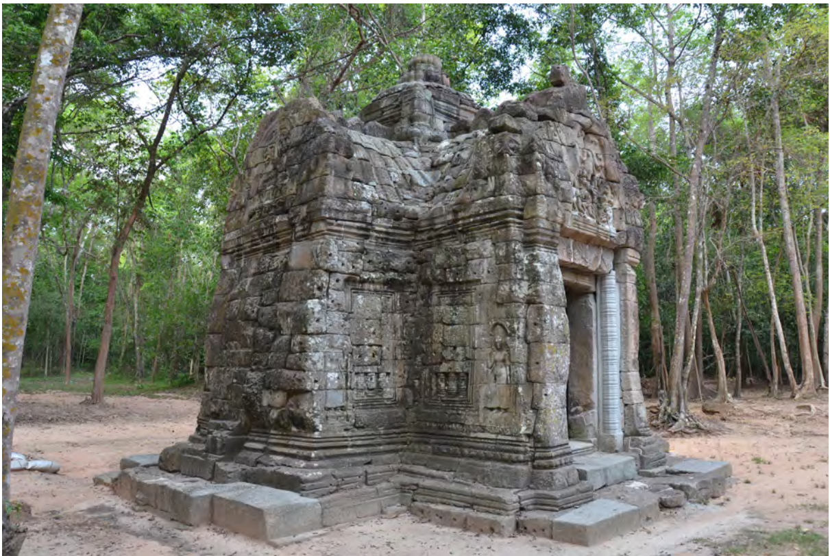
Southwest elevation after restoration
