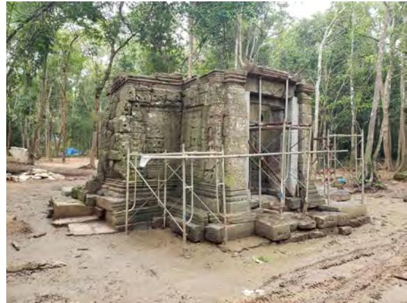
Figure 9.2.20 Work progress in October, 2020 (Northwest view)
