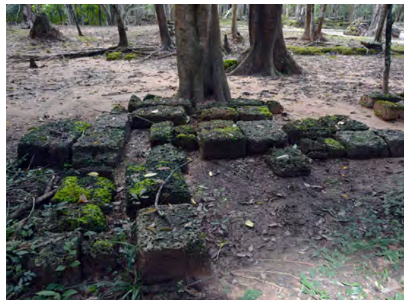
Figure 9.2.118 Original substrate laterite blocks below the floor sandstones that could not be reused during restoration
