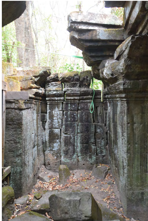
North inner elevation before dismantlement
