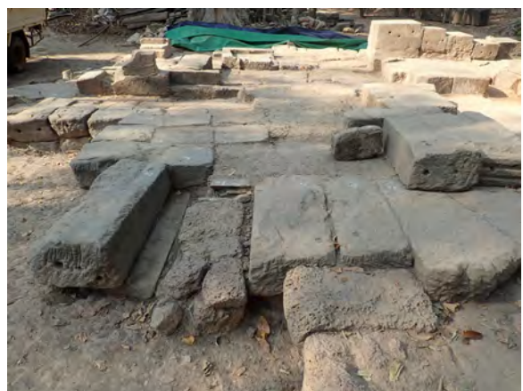
Figure 5.2.42 Laterite block irregularly inserted at the southwestern outer corner of the East Gate's south wing
