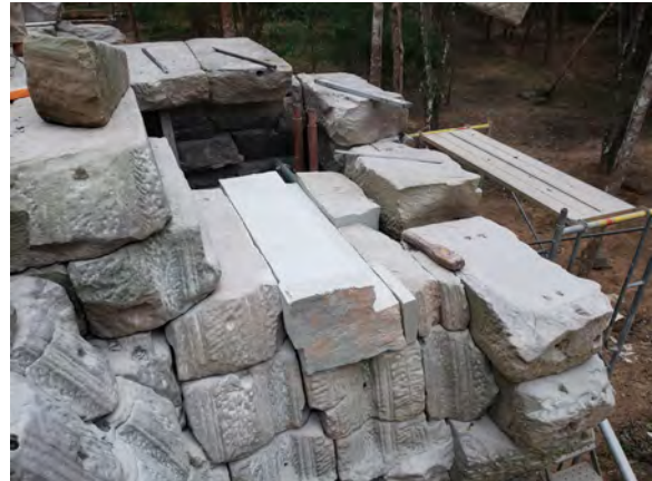
Figure 9.2.79 Reassembly of the roof structure
