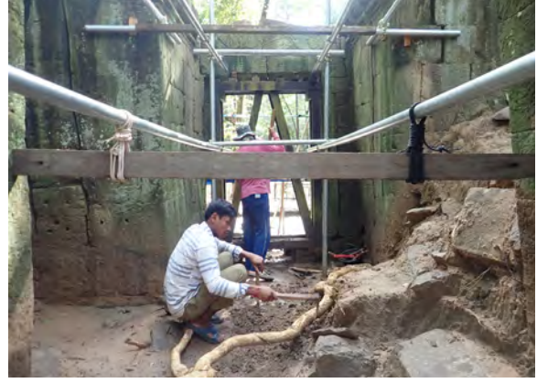
Figure 4.2.7 Cleaning work inside the East Gate
