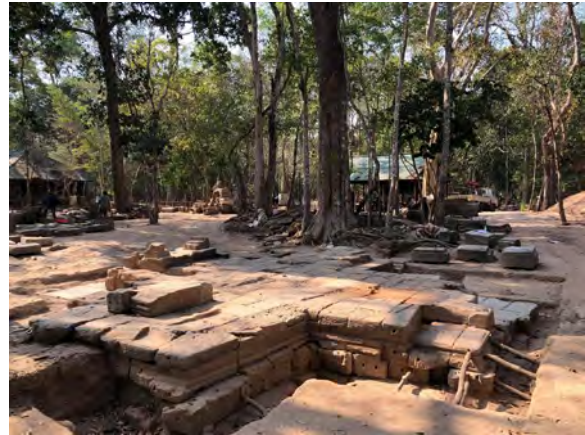
Figure 9.2.2 Work progress in March, 2020 (Southeast view)
