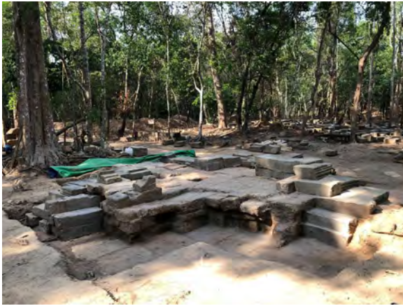
Figure 9.2.7 Work progress in April, 2020 (Southwest view)
