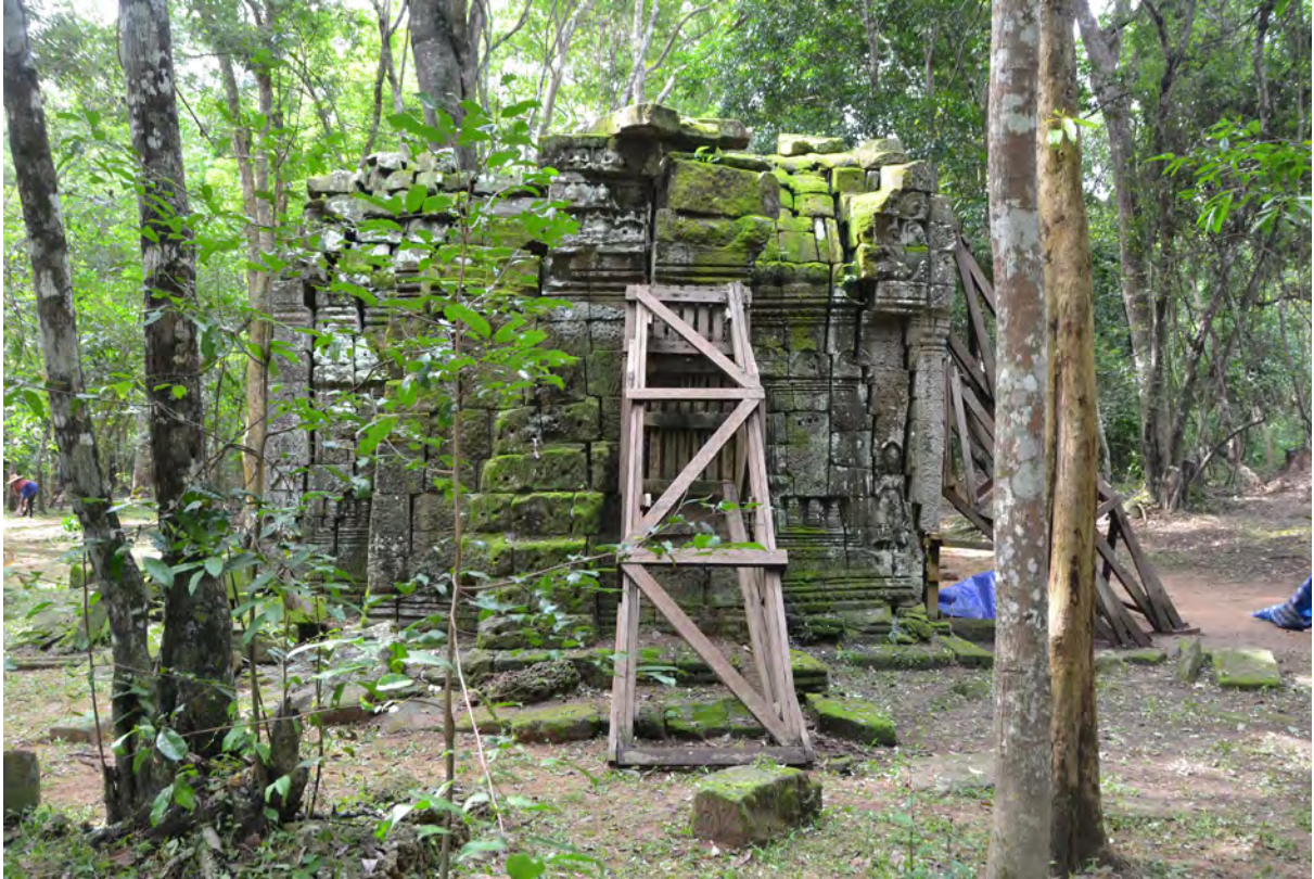
South elevation before restoration in July, 2017
