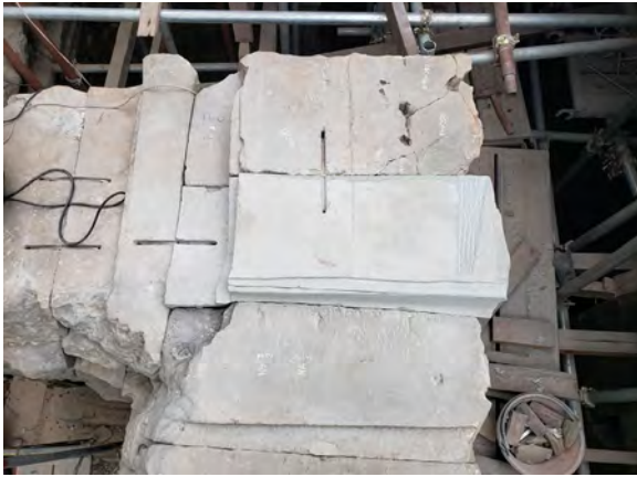
Figure 9.2.78 Stainless steel clamps used to consolidate the roof structure's inner corner
