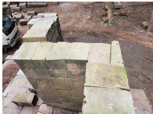
Figure 5.2.14 Stone joints at wall corners
