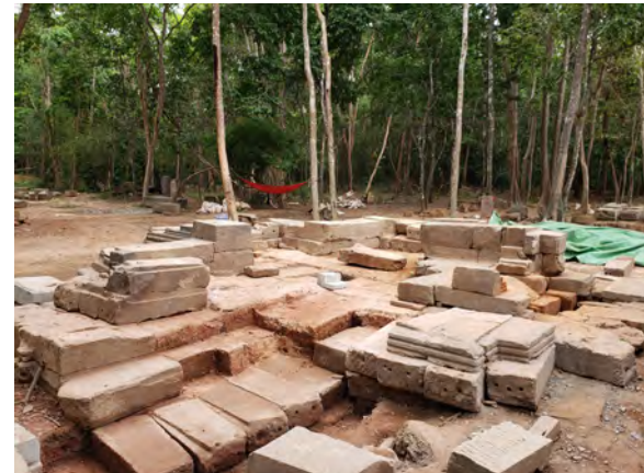
Figure 9.2.53 Reassembly of the exterior sandstones in the northwest area
