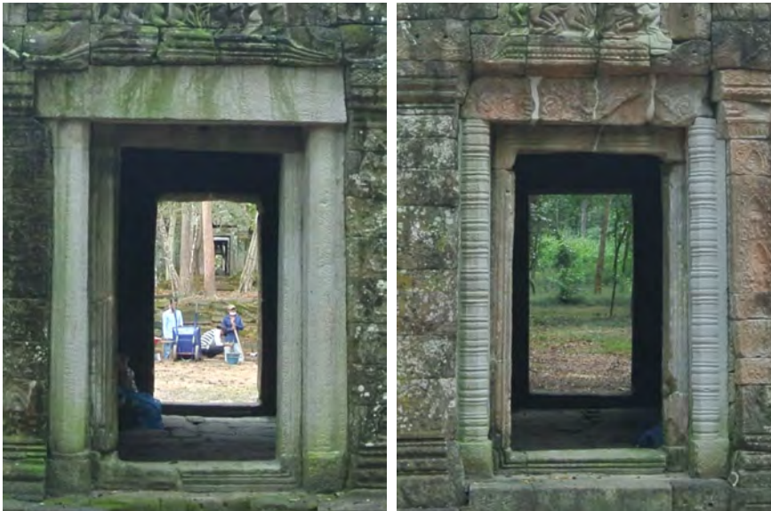
Figure 8.3.7 Lintel and colonettes after restoration (eastern and western faces)
