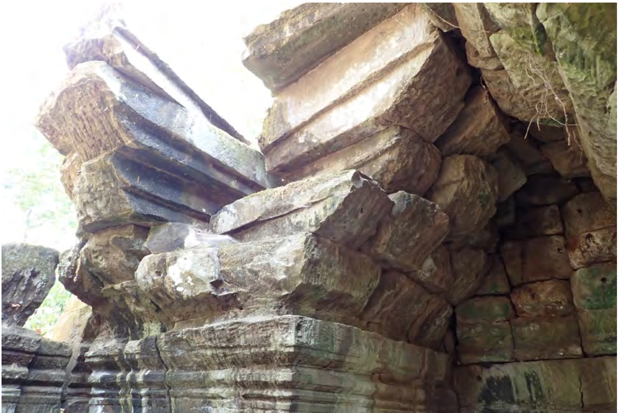
Northeast ceiling before dismantlement in January, 2019
