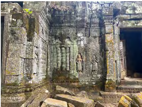
Figure 3.2.12 South side of north wing
