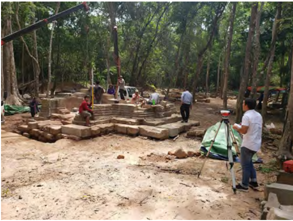
Figure 9.2.58 Checking the base structure's level during reassembly
