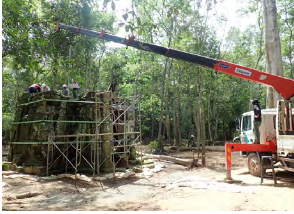
Figure 4.2.6 Dismantlement of roof structure using a crane truck
