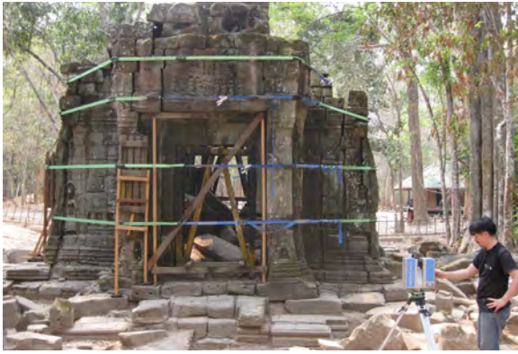
Figure 4.1.10 3D laser scanning
