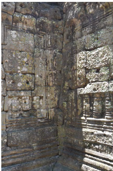
Figure 3.2.20 Wall intersection, East Gate
