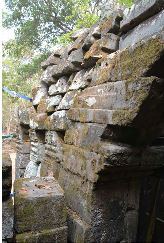
South side of the west wing's roof before dismantlement in March, 2019
