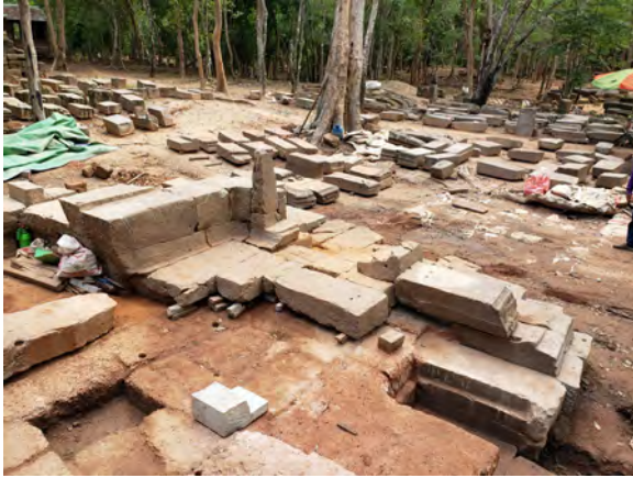
Figure 9.2.56 Trial reassembly of the floor sandstones
