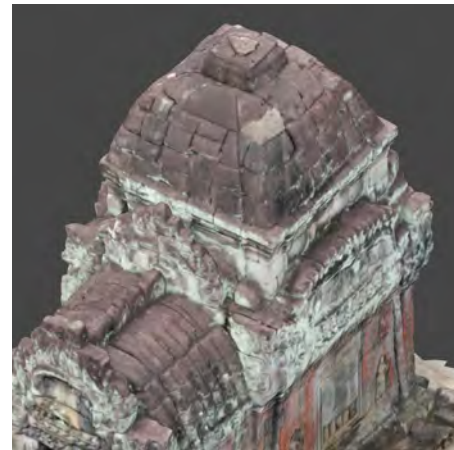
Figure 3.2.39 Roof structure of the Sub-shrine
