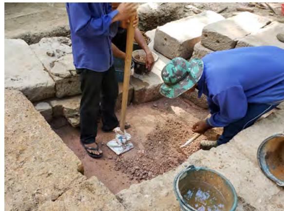
Figure 9.2.41 Compaction of Layer 20's top surface in the west wing
