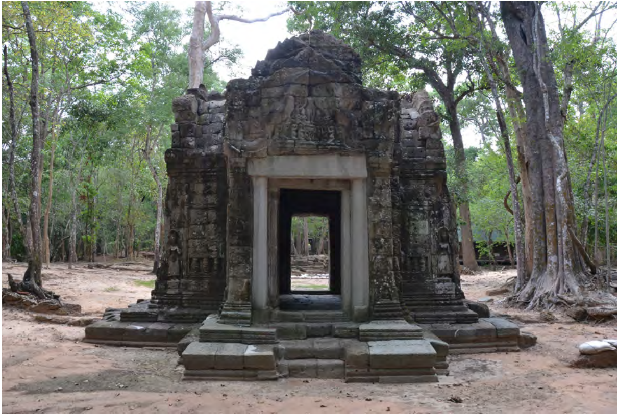
East elevation after restoration
