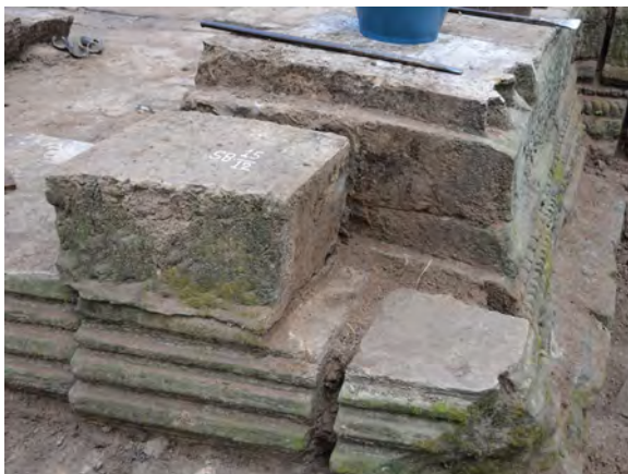
Figure 5.2.13 Extremely small sandstone at the base structure's outer corner
