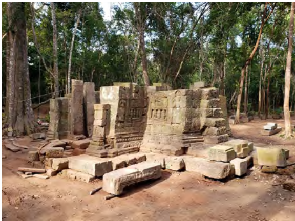
Figure 9.2.15 Work progress in September, 2020 (Southwest view)
