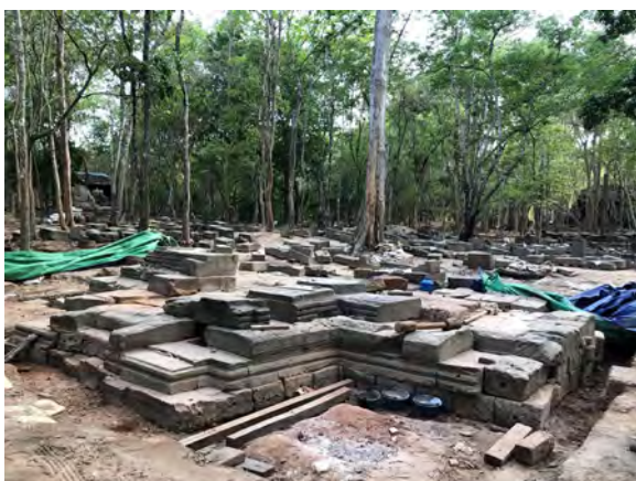
Figure 9.2.5 Work progress in April, 2020 (Northeast view)
