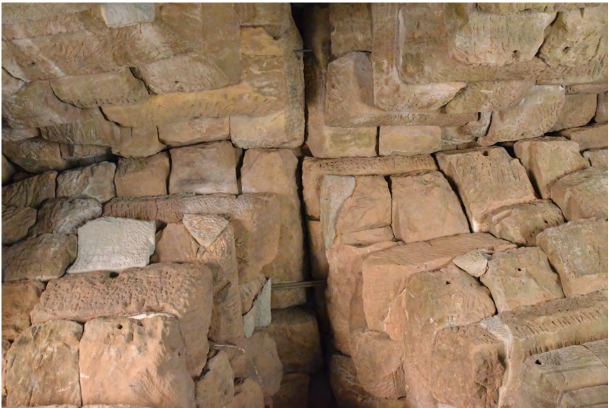
Ceiling after restoration
