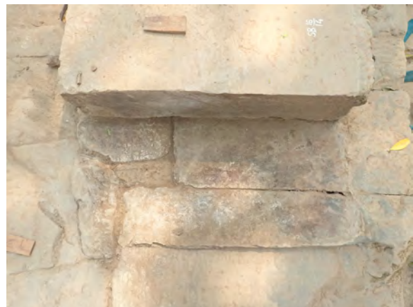
Figure 5.2.12 A gap filled with an adjustment material comprising soil mixed with either sandstone or laterite chips
