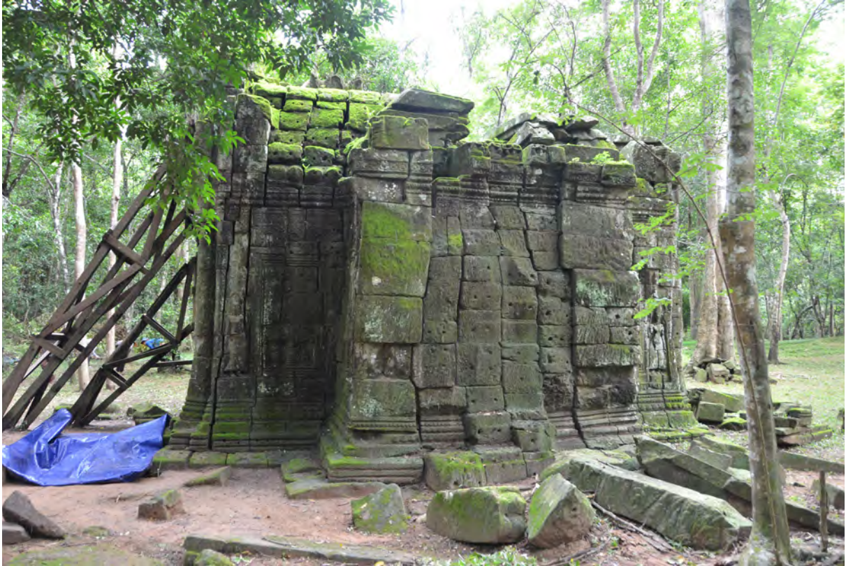
North elevation before restoration in July, 2017
