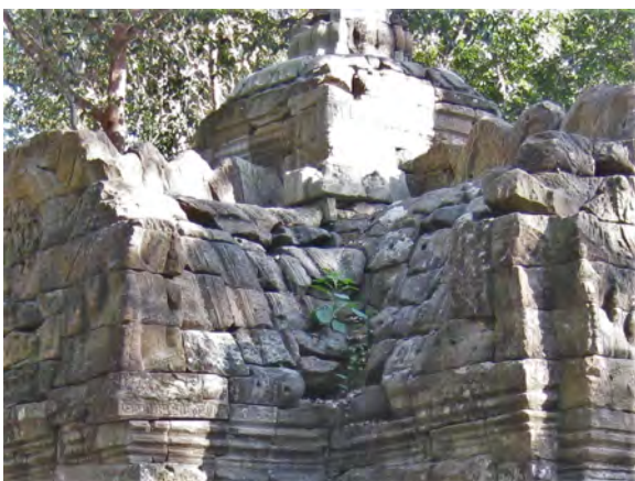
Figure 9.2.98 Roof at the northwest corner before retouching
