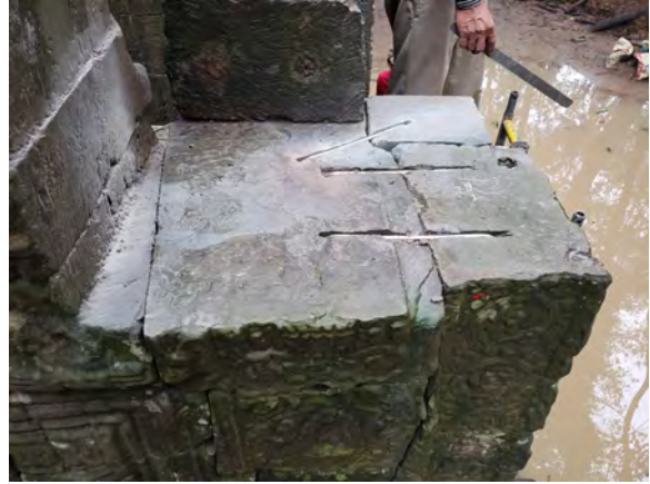
Figure 9.2.67 Stainless steel clamps inserted to prevent stone displacement
