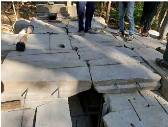
Figure 8.3.4 Insertion of stainless steel rods at the centre of the roof
