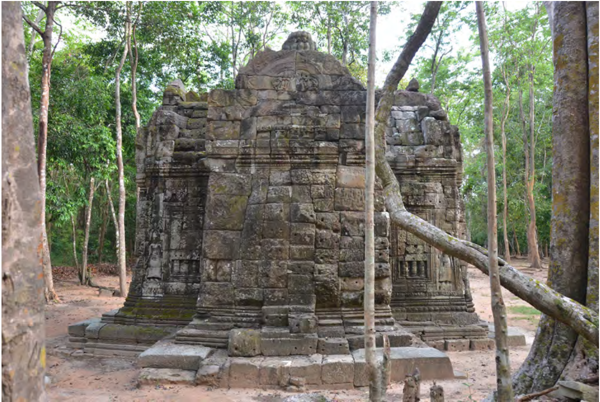
North elevation after restoration
