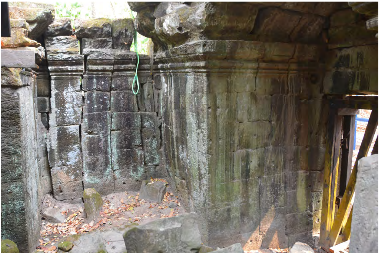
Northeast inner wall before dismantlement in March, 2019
