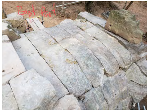
Figure 9.2.85 Curved ditch to place the roof ridge
