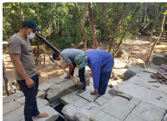
Figure 9.2.81 Consolidation of the cross-vault structure in the east-west direction
