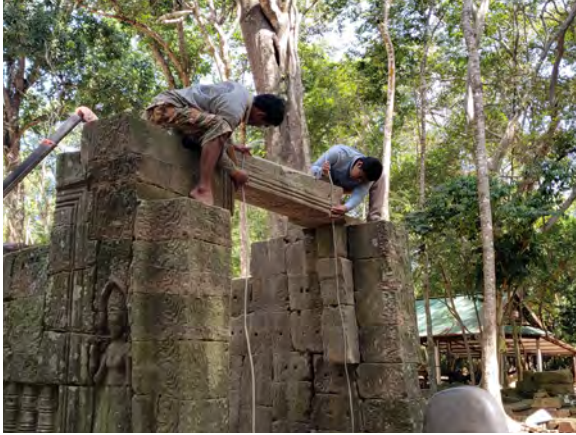
Figure 9.2.66 Trial reassembly of the door frame at the east entrance
