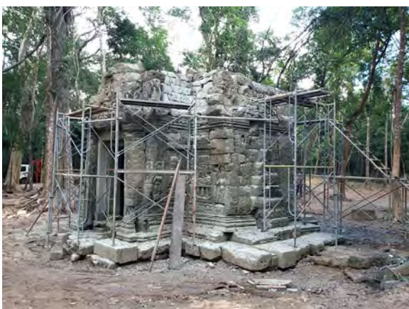
Figure 9.2.23 Work progress in November, 2020 (Southwest view)
