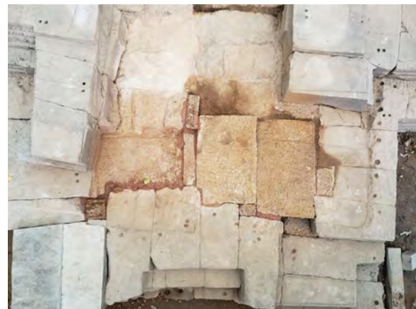
Figure 9.2.37 New laterite replacing deteriorated substrate laterite in the east wing
