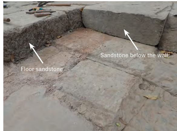
Figure 5.2.4 Difference in processing precision
