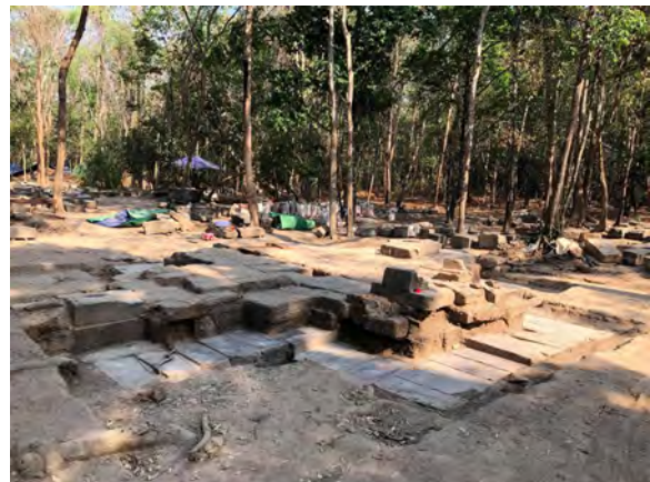
Figure 9.2.4 Work progress in March, 2020 (Northwest view)
