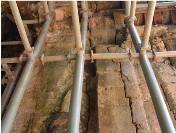
Figure 3.2.45 Traces of the wooden members at the causeway, Ta Prohm Temple
