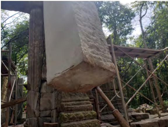
Figure 9.2.68 Mortise created on the new colonette's bottom surface
