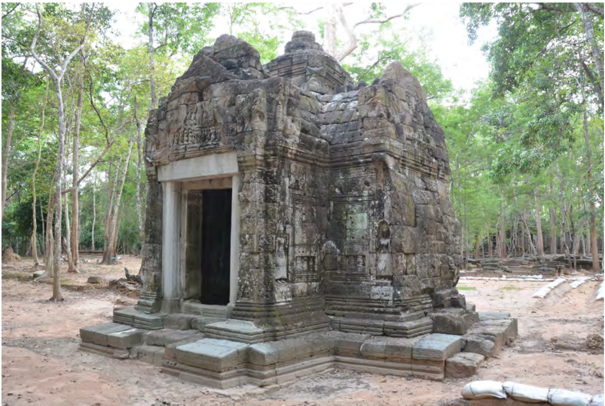
Northeast elevation after restoration
