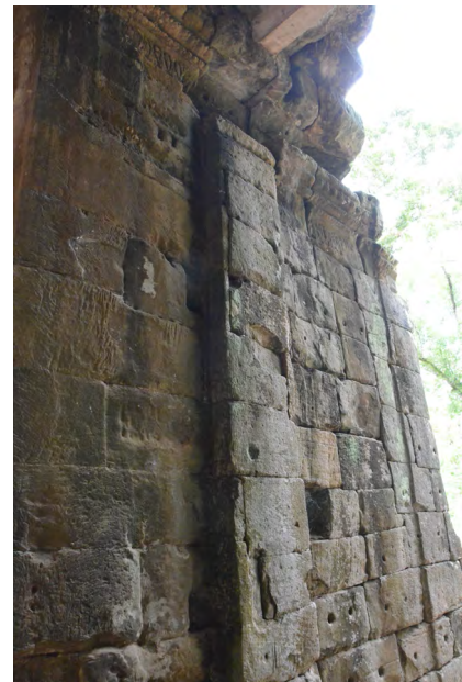
Figure 3.2.50 Traces of the wooden members at the causeway, Banteay Kdei Temple
