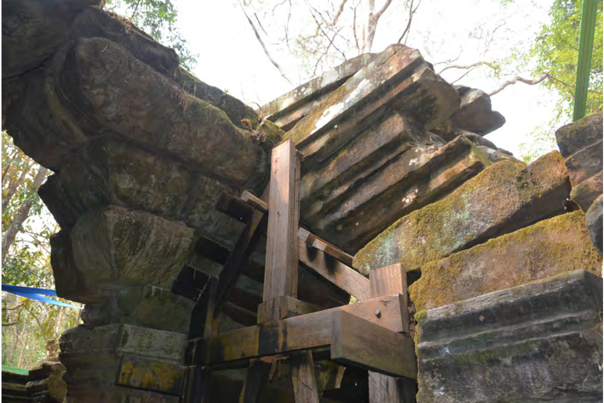
South ceiling before dismantlement in March, 2019
