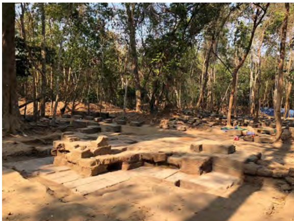
Figure 9.2.3 Work progress in March, 2020 (Southwest view)
