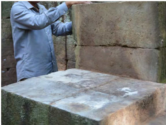
Figure 5.2.3 Smoothed upper surfaces of the sandstone wall
