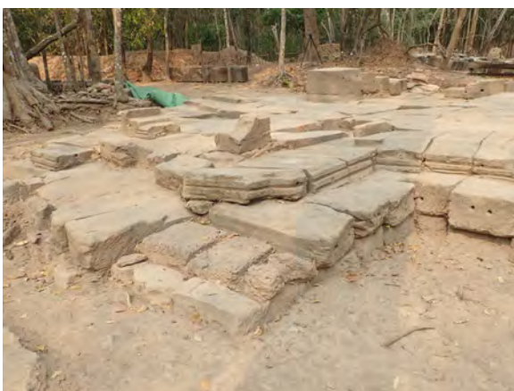
Figure 5.2.41 Laterite block irregularly placed at the southwestern outer corner of the East Gate's western entrance
