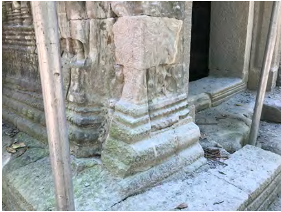
Figure 9.2.102 Repair with sandstone fragments
