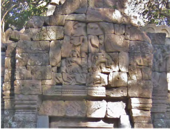
Figure 9.2.100 West lintel and pediment before retouching
