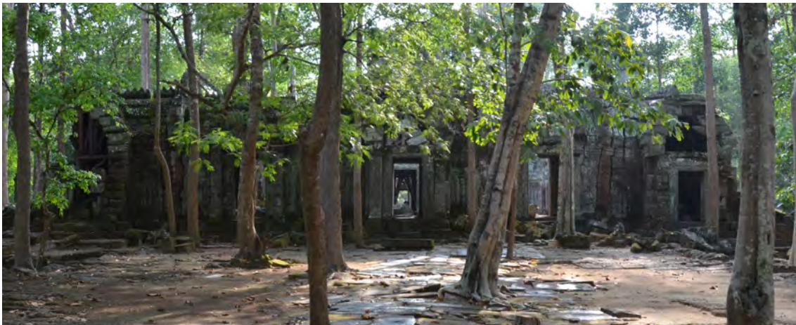
Figure 3.2.9 Entire view of the east side of the Inner Gallery
