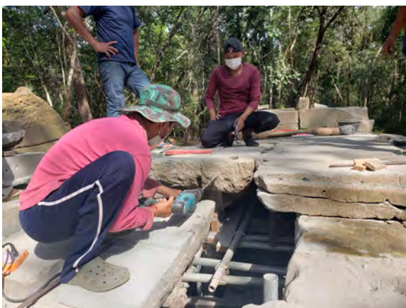
Figure 9.2.80 Consolidation of the cross-vault structure in the east-west direction
