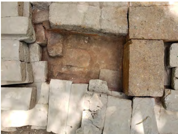
Figure 9.2.40 Condition of the substrate laterite in the west wing (Layer 20)
