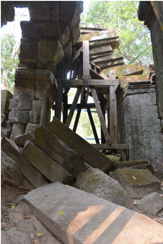
West inner elevation before dismantlement
