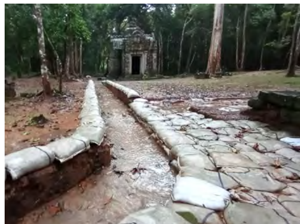
Figure11.1.4 Water drainage during the rainy season
