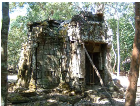
Figure 2.1.1 East Gate before restoration in 2004
