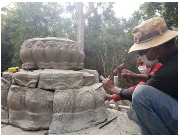
Figure 9.2.104 Engraving the finial's new stones
