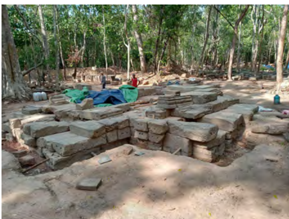
Figure 9.2.11 Work progress in May, 2020 (Southwest view)
