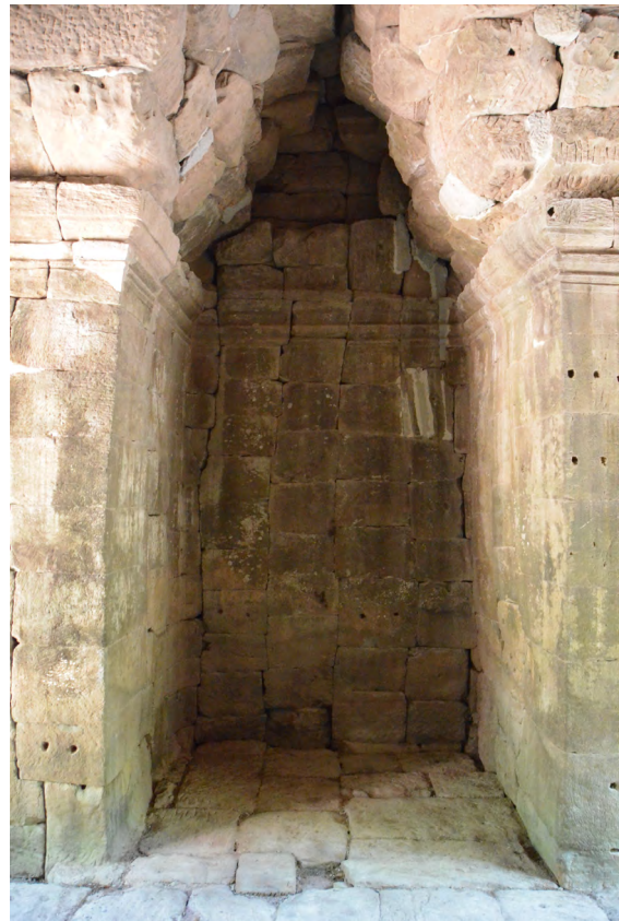
North inner elevation after restoration
