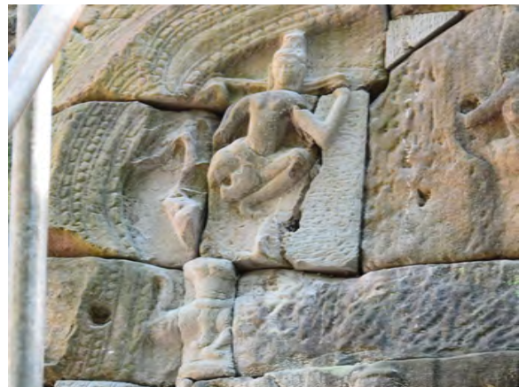
Figure 8.3.5 Supplementary new stones at the southern pediment (work in progress)
