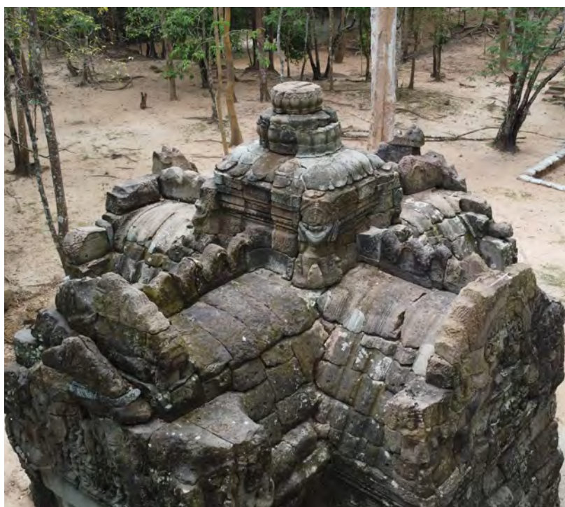
Figure 3.2.14 Roof structure of the East Gate
