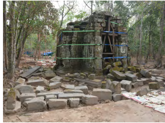
Figure 2.1.3 Collapsed members of the East Gate found during the excavation
