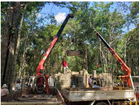
Figure 9.2.60 Reassembly of the wall using two crane tracks
