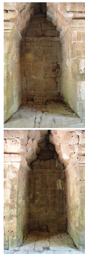
Figure 3.2.2 (top) South interior view Figure 3.2.3 (bottom) North interior view
