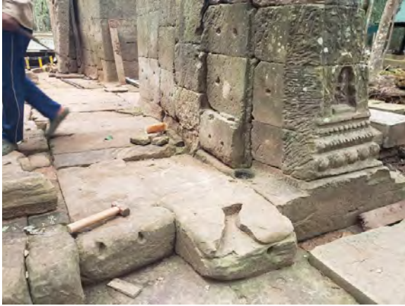
Figure 5.2.24 Circular mortise in the northeastern corner where the colonette stands
