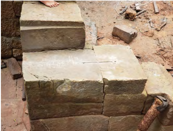
Figure 9.2.62 Stainless steel clamps inserted to prevent stone displacement
