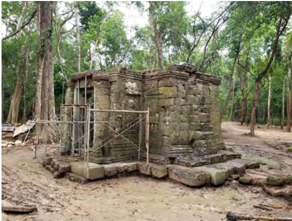
Figure 9.2.19 Work progress in October, 2020 (Southwest view)
