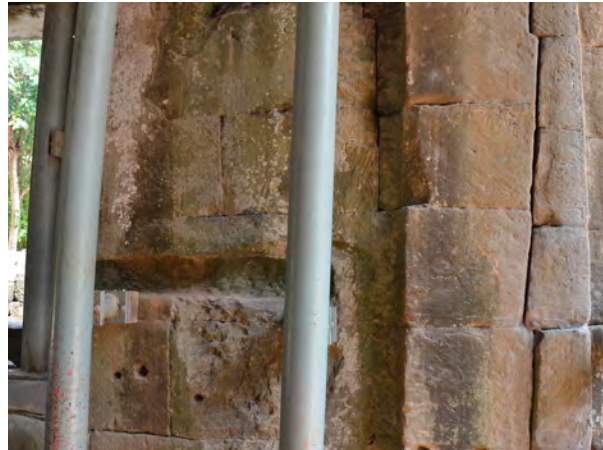
Figure 3.2.46 Traces of the wooden members at the causeway, Ta Prohm Temple
