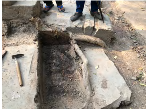
Figure 9.2.27 Tree root's penetration of the base structure
