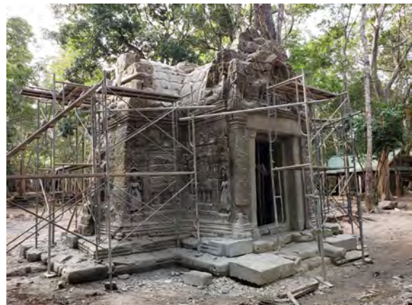
Figure 9.2.22 Work progress in November, 2020 (Southeast view)
