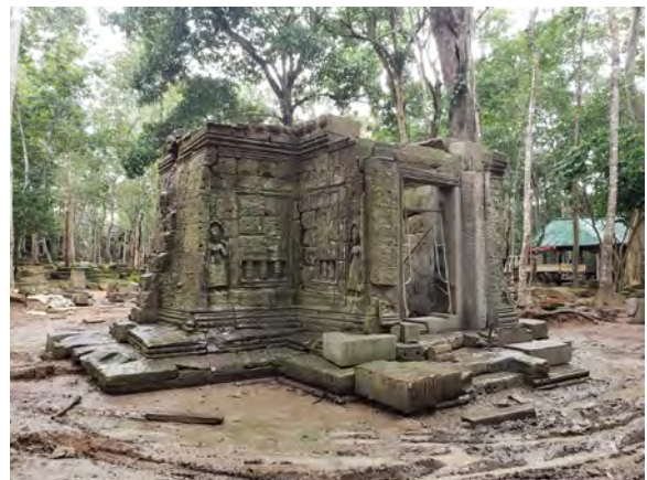
Figure 9.2.18 Work progress in October, 2020 (Southeast view)
