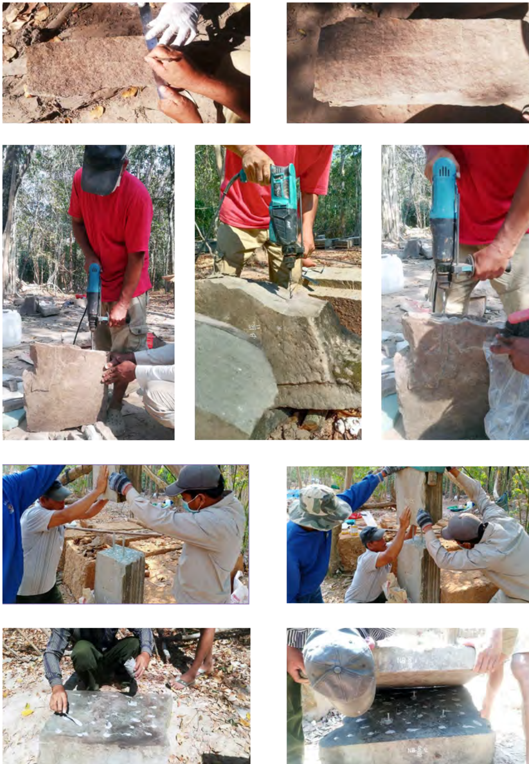
Figure 9.1.10 Drilling and gluing process
