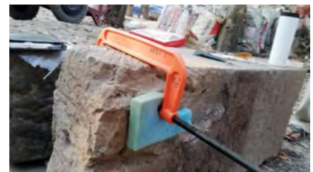
Figure 9.1.9 Use of adhesives for connecting the broken stone pieces
