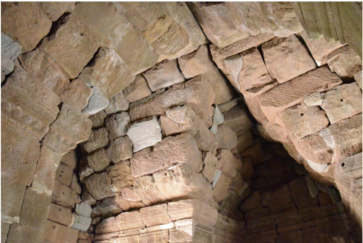
Northwest side of the ceiling after restoration
