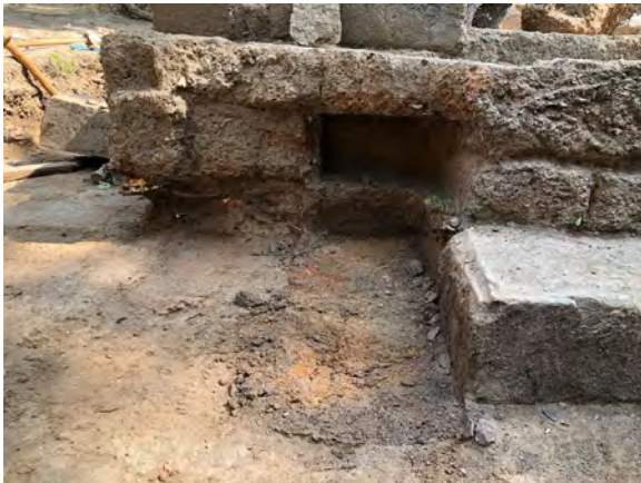
Figure 5.2.9 Absence of substrate laterite
