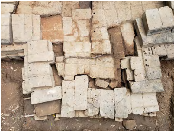
Figure 9.2.38 Condition of the substrate laterite in the west wing (Layer 18)
