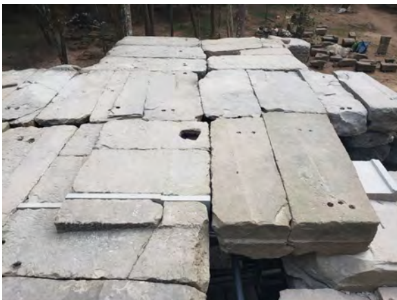
Figure 5.2.34 Roof stone layout on layer 01, with a palm-sized hole artificially drilled into the northeastern roof stone's upper surface
