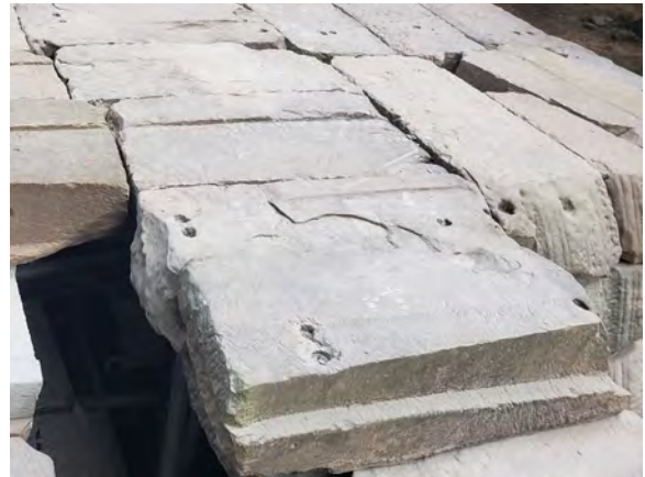
Figure 5.2.33 Sloped step-shaped roof stone joints
