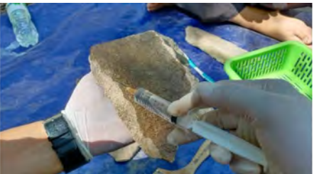
Figure 9.1.8 Stone reinforcement process
