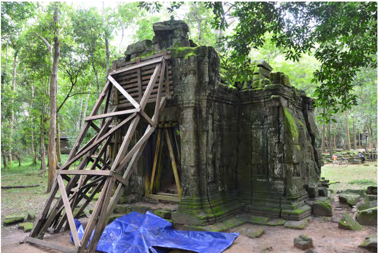
Northeast elevation before restoration in July, 2017
