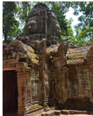
Figure 3.2.34 The external corner of the wall
