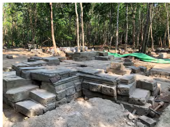
Figure 9.2.12 Work progress in May, 2020 (Northwest view)
