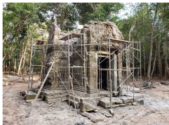
Figure 9.2.24 Work progress in November, 2020 (Northwest view)
