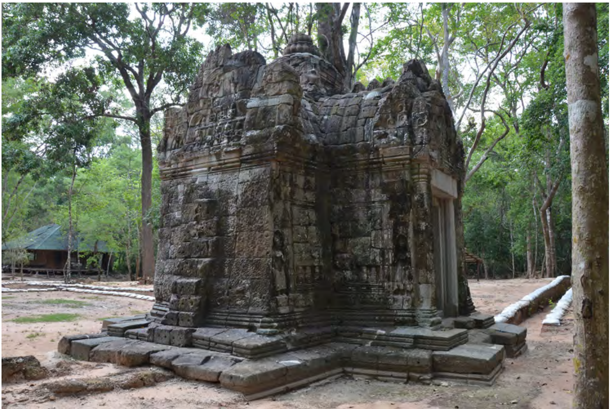
Southeast elevation after restoration
