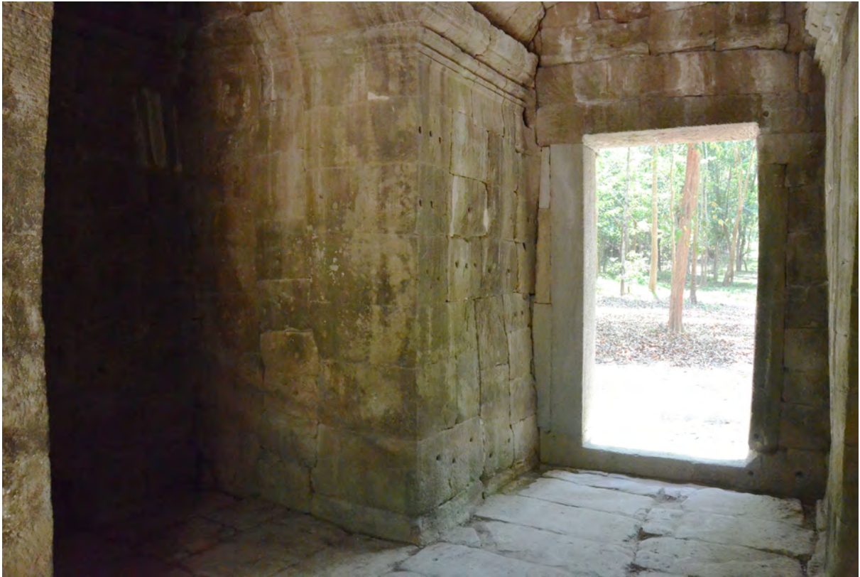
Northeast inner elevation after restoration
