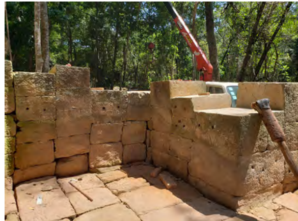
Figure 9.2.59 Wall reassembly
