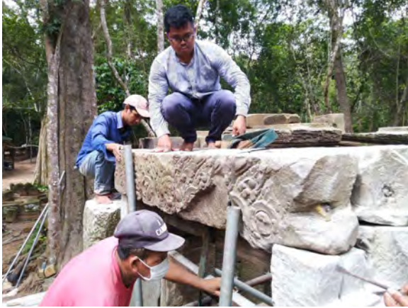
Figure 9.2.76 Assembly of the original lintel after repair
