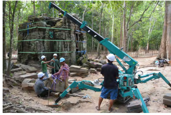
Figure 4.1.11 Organization of scattered stones using a spider crane
