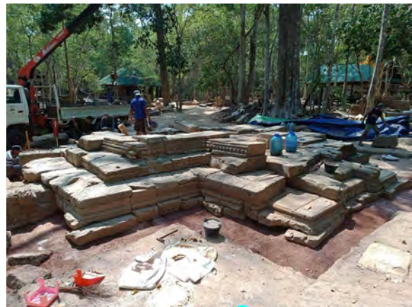
Figure 9.2.10 Work progress in May, 2020 (Southeast view)
