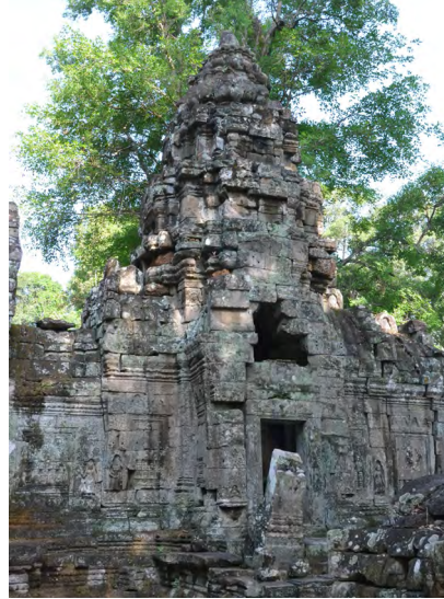
Figure 3.2.30 The South Gate of the East Gate
