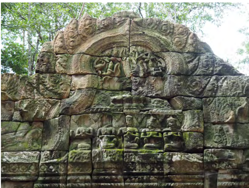
Figure 10.16 North pediment of the East Gate, the Outermost Enclosure, Ta Nei
