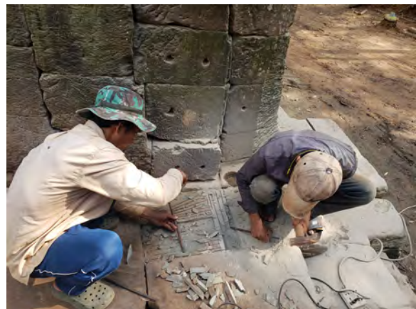
Figure 9.2.61 Scraping new sandstones' surface to place the door frame
