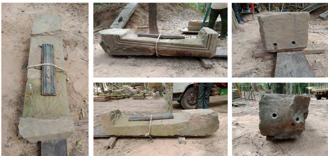
Figure 9.2.65 Horizontal door frame reinforcement
