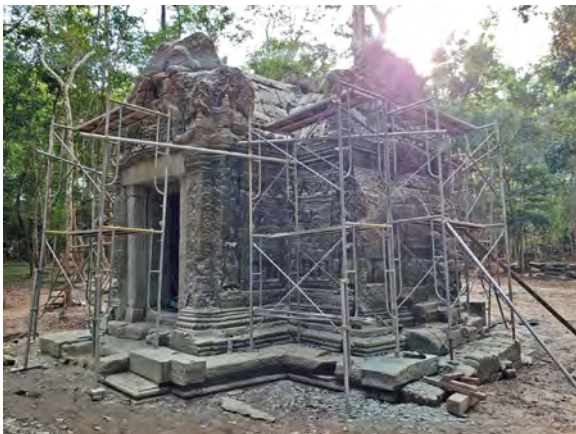
Figure 9.2.21 Work progress in November, 2020 (Northeast view)
