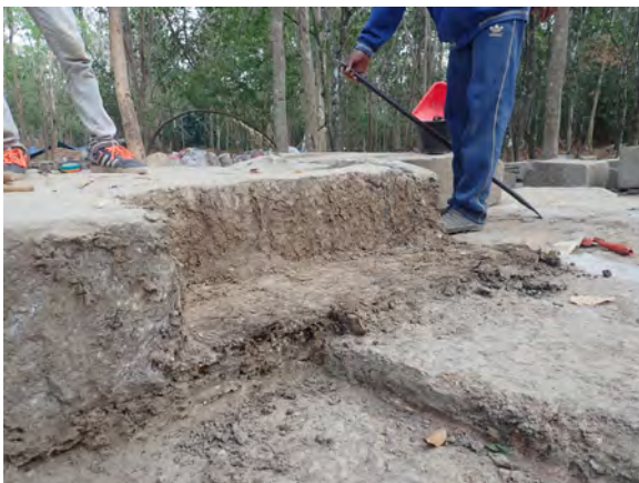
Figure 5.2.11 Material used to adjust the floor sandstones' unevenness
