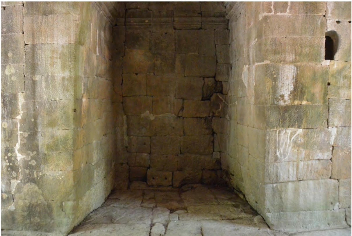
South inner elevation after restoration
