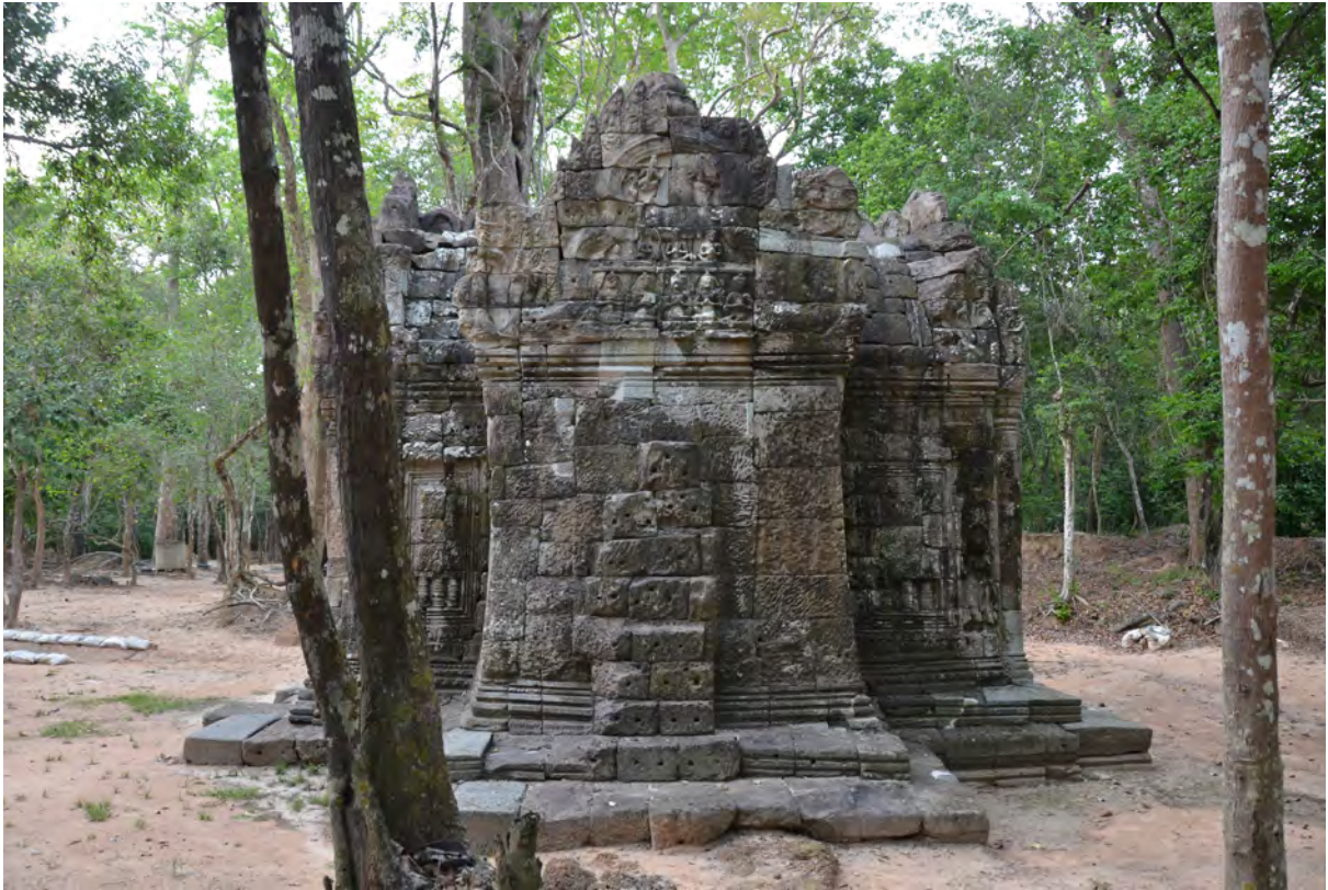
South elevation after restoration
