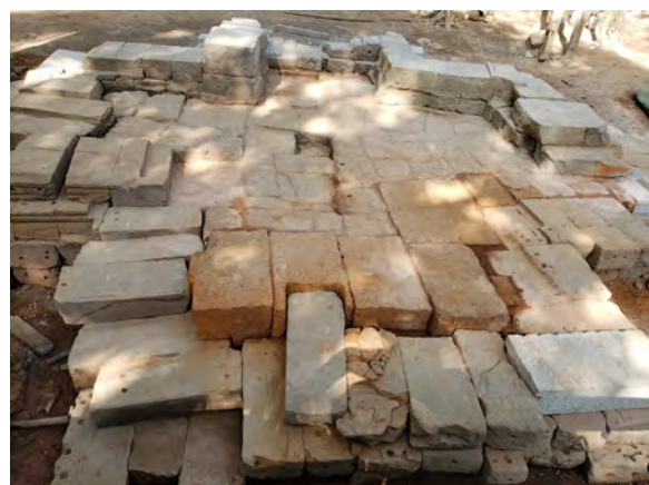
Figure 9.2.43 New laterite replacing deteriorated substrate laterite in the west wing
