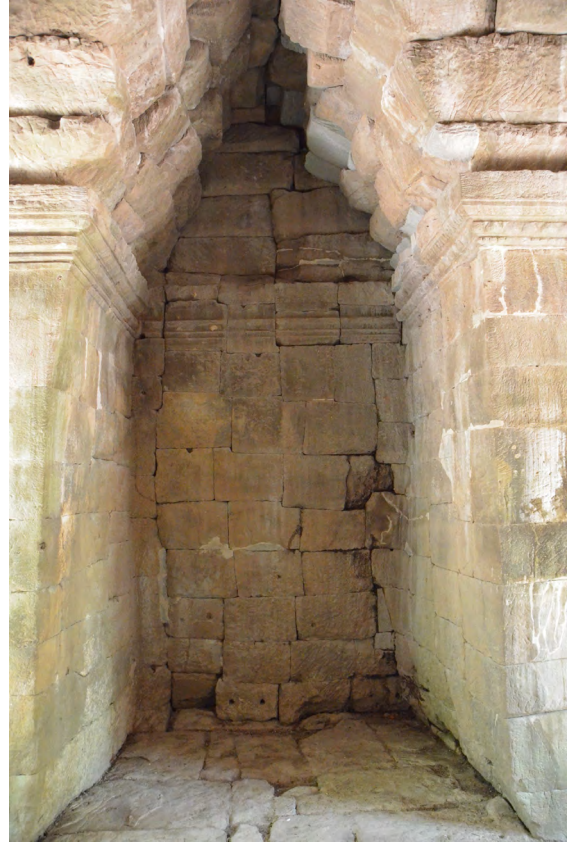
South inner elevation after restoration
