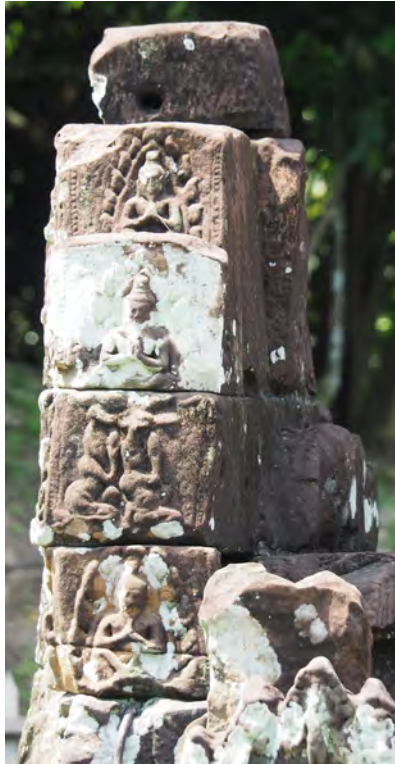
Figure 10.1.13 North side of the frame of the east pediment on the east secondary pool, Neak Pean
