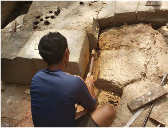
Figure 9.2.50 Cutting the displaced laterite to fix the exterior sandstones
