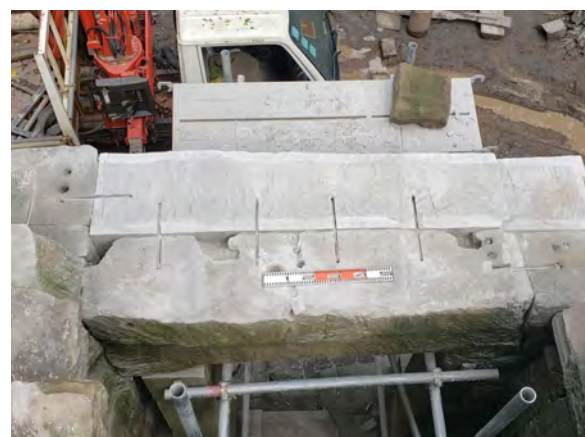
Figure 8.3.3 Metal clamp fixing on the eastern lintel's upper surface
