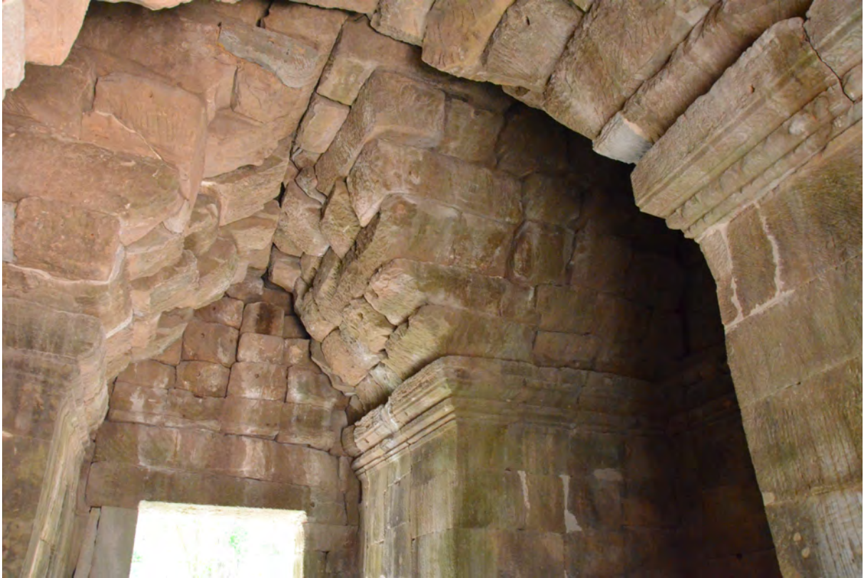
Southeast side of the ceiling after restoration
