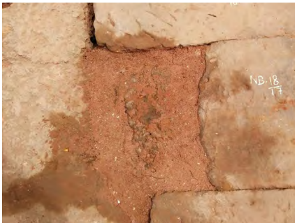
Figure 9.2.46 Use of lime mortar to fill gaps
