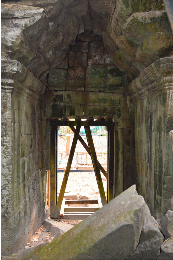
East inner elevation before dismantlement
