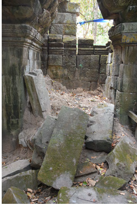
South inner elevation before dismantlement
