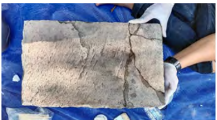
Figure 9.1.9 Use of adhesives for connecting the broken stone pieces
