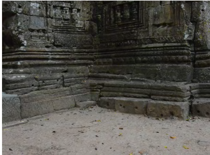
Figure 3.2.5 Traces of adjustment of the difference in height at the base
