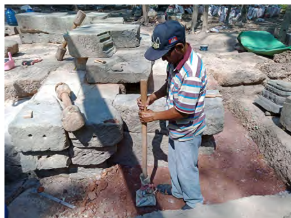
Figure 9.2.49 Compaction of lime mortar in the area surrounding the base structure
