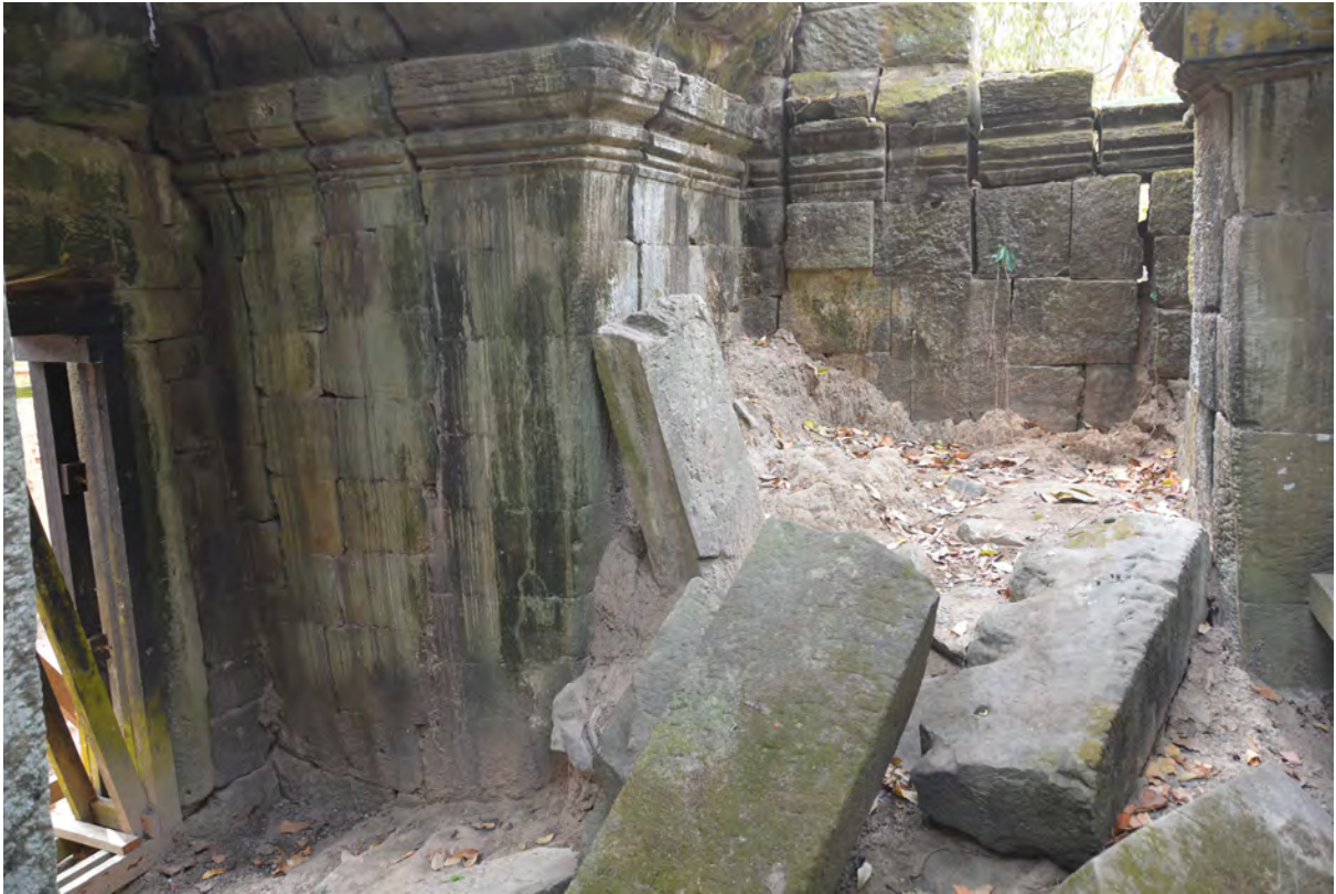
Southeast inner wall before dismantlement in March, 2019
