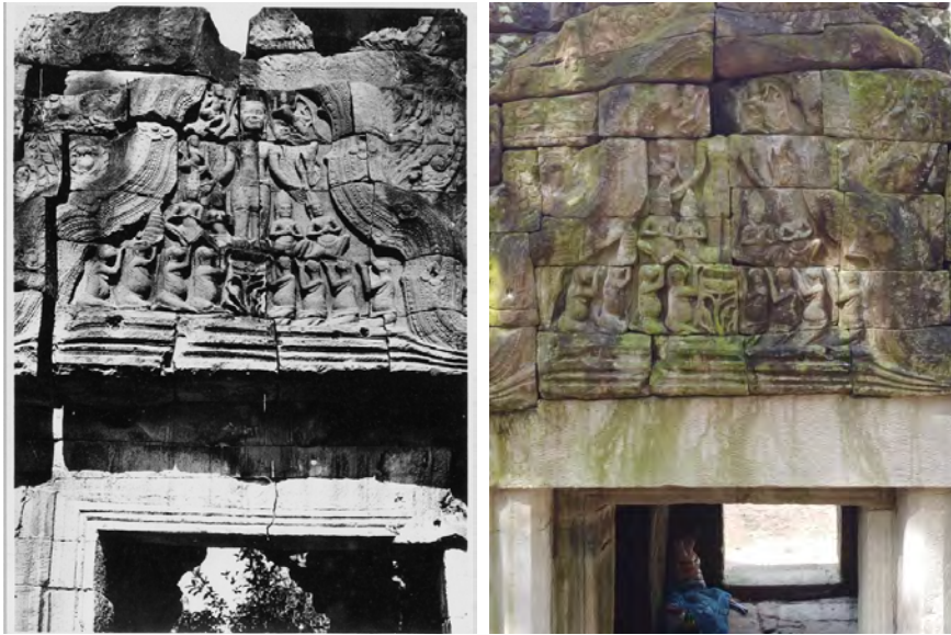
Figure 8.3.6 Eastern pediment, photos from ca. 1930 (Left: EFEO_CAM08916) and after restoration (Right)
