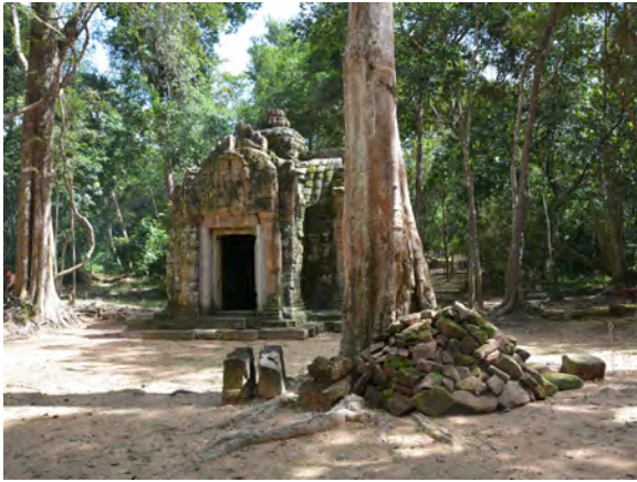
Figure 9.2.115 Original sandstone members not reused during the restoration
