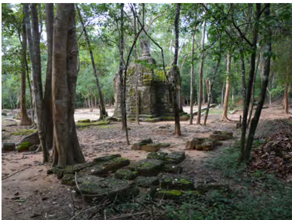
Figure 9.2.117 Original substrate laterite blocks below the floor sandstones that could not be reused during restoration
