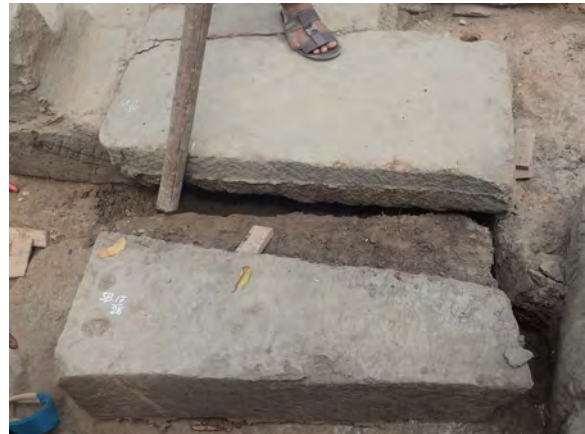
Figure 5.2.10 Exterior sandstone placed under floor sandstone
