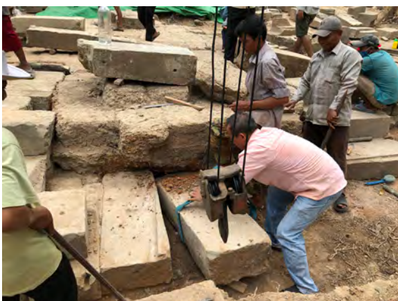
Figure 9.2.30 Dismantling the exterior sandstone
