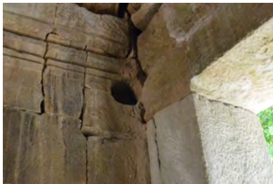
Figure 3.2.17 / Figure 3.2.18 Traces of the wooden members of the east entrance, East Gate
