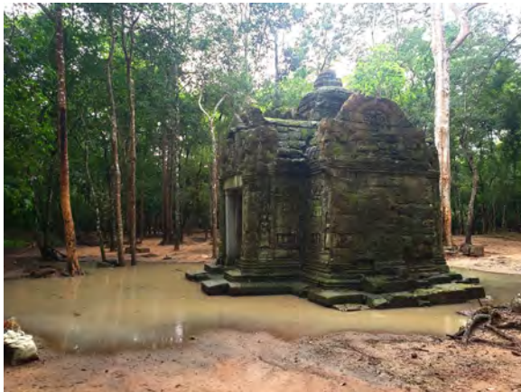
Figure 9.3.1 Water stagnation surrounding the East Gate (November 2021)
