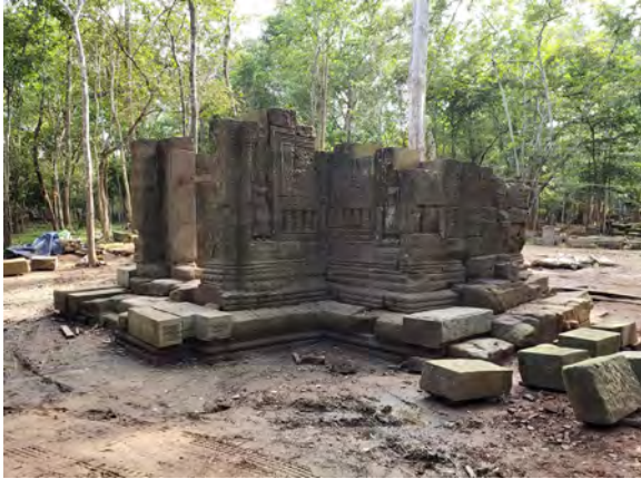
Figure 9.2.13 Work progress in September, 2020 (Northeast view)
