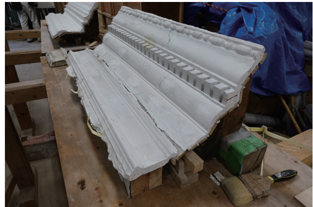
Pic10. Plastered cornice dismantled by the method of Oobarashi (Photography by the author)
