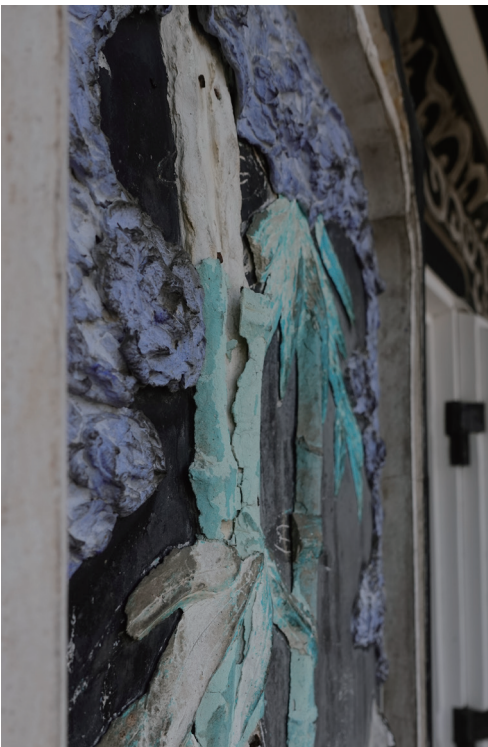
Pic21 (left). The flaking of plaster finish on the surface
