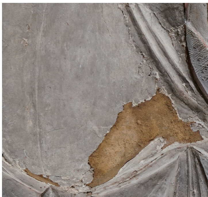
Pic11. Exposure of base sheet due to plaster removal (Photography by the author)
