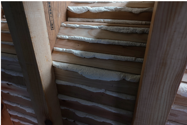
Pic9. Experimental installation on assembled wooden laths (Photography by the author)
