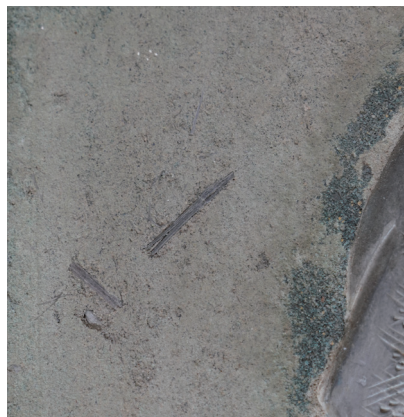
Pic5. Rough straws on the clay wall (Photography by the author)
