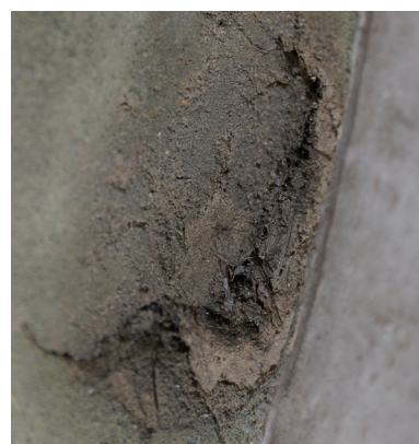
Pic12. Resin impregnation treatment (Photography by the author)
