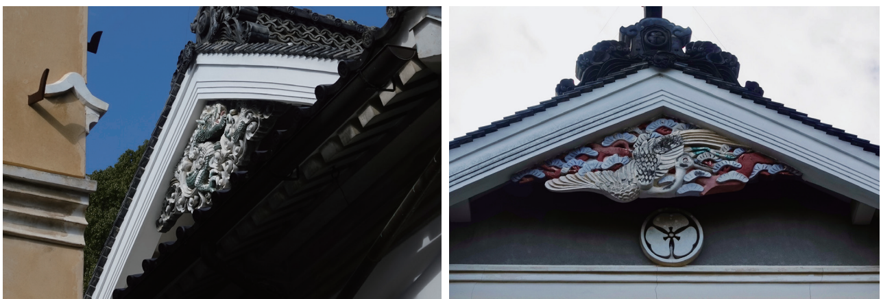
Pic27. Kotee applied to the gegyo of Honhaga-ke Residence (Photography by the author)
