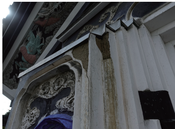
Pic24. Fracks of plaster and flowed-out clay wall (Photography by the author)
