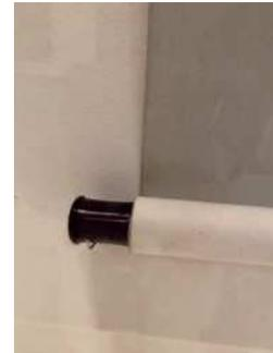
Figure 11 Lower baton (jikushu) rolled and supported with wall mounted brackets. The metal is covered with silicon tubing.
